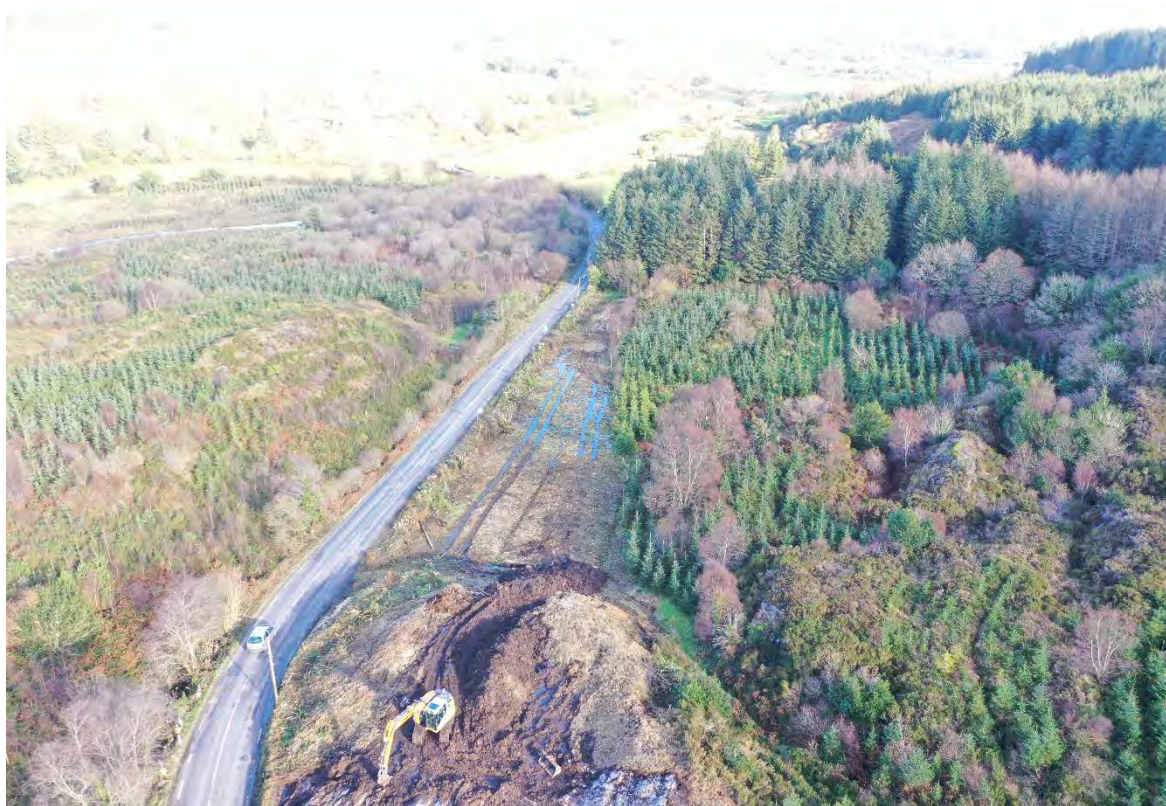
Figure 4 Aerial view looking east along the R585
