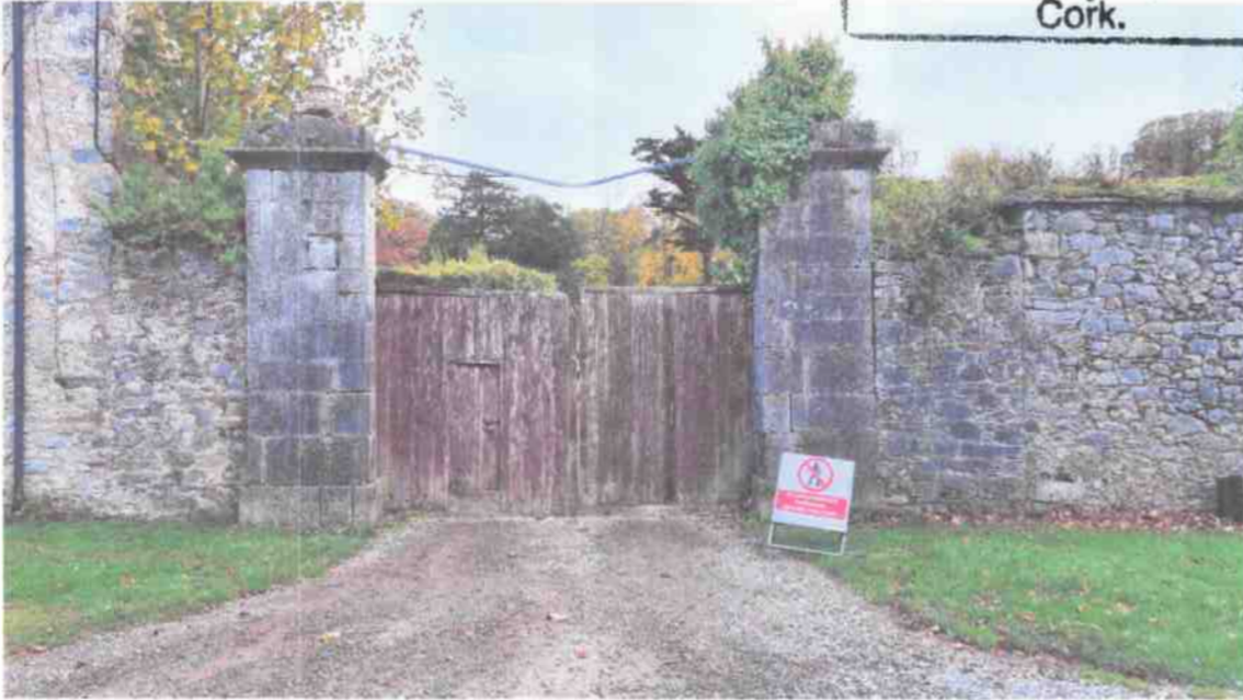
Fig 3 View facing north onto the access road.
