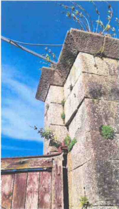
Fig. 45 Condition of ironmongery before the works
