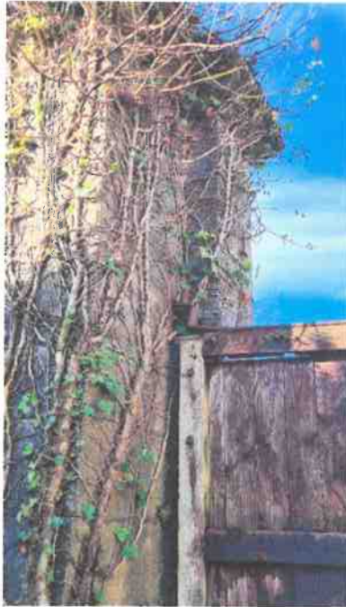
Fig. 3 Southwest pier - top
