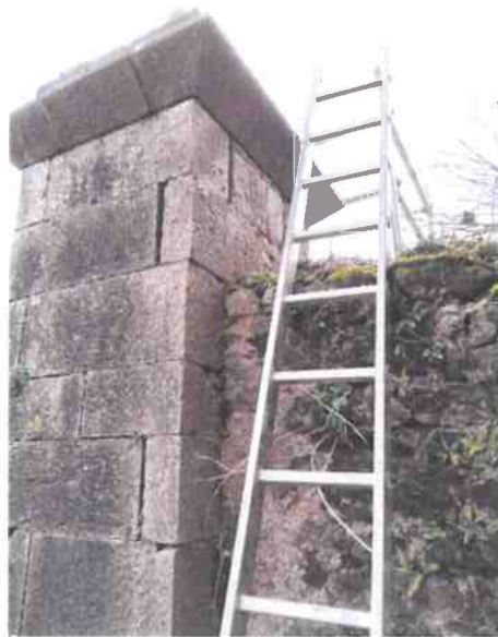
Fig. 15 inside Northeast pier
