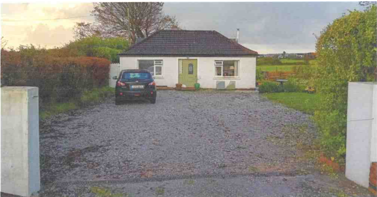
View from North-West (Road) on pre-existing Gable
