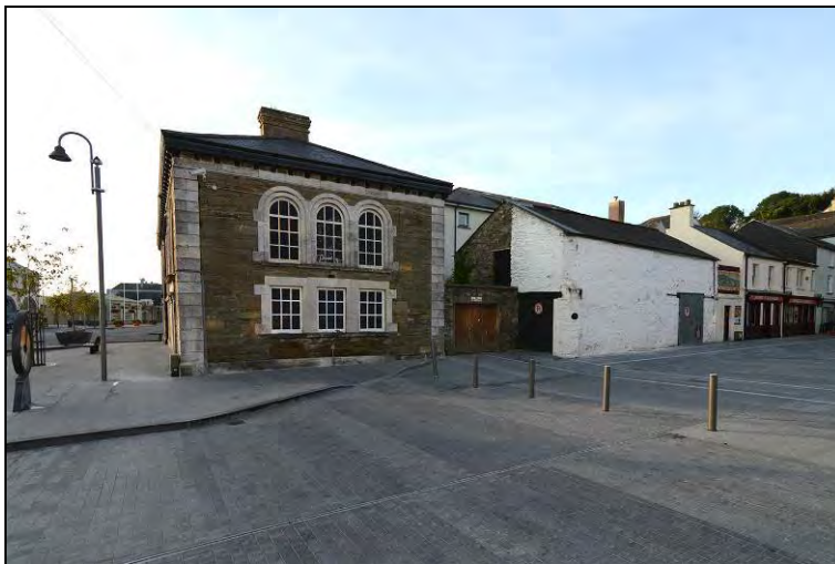
Photograph 7: North elevation of the Courthouse, and the Soup-Kitchen adjoining it.
