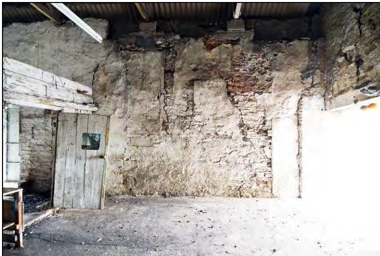
Photograph 16: Interior north elevation of the eastern space.
