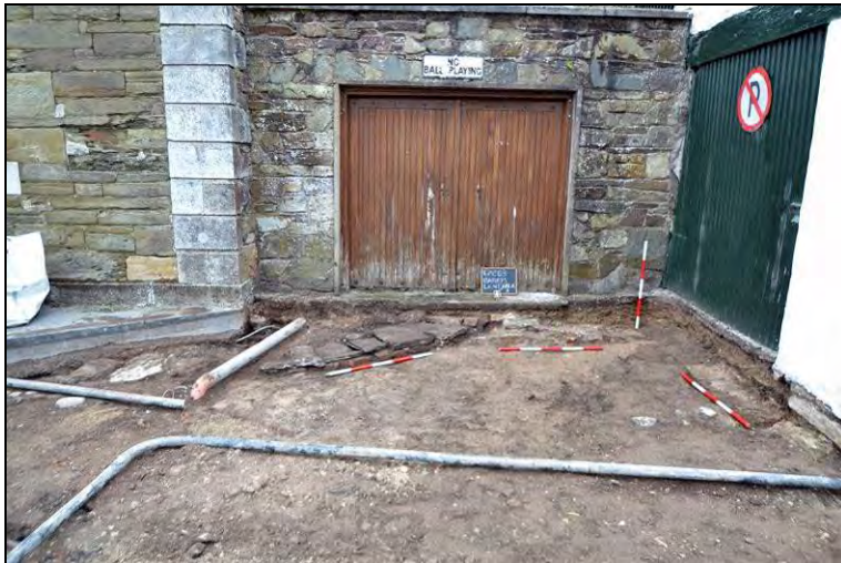
Photograph 28: Vehicle entrances to the Courthouse and the Soup Kitchen, 2018.
