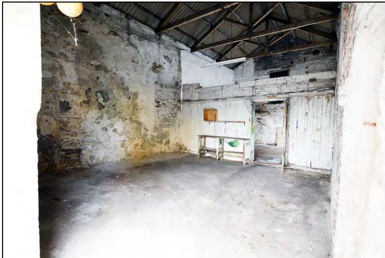
Photograph 13: View looking southwest into the east half of the Soup Kitchen. Note the timber partition, a combination of recycled window shutters, panels and boards.
