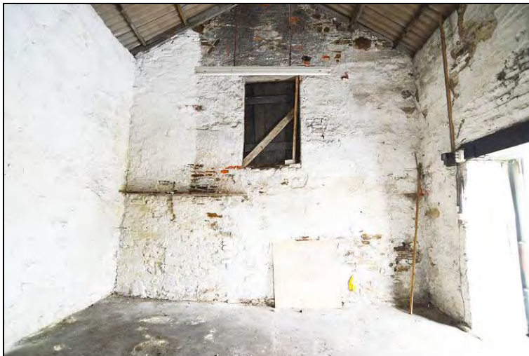
Photograph 19: Interior elevation of the east gable, from the western space.
