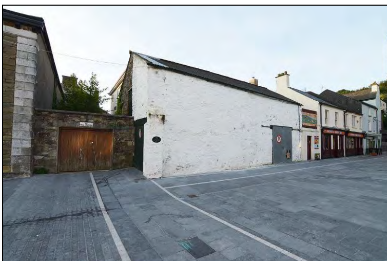
Photograph 8: North elevation of the Soup-Kitchen.
