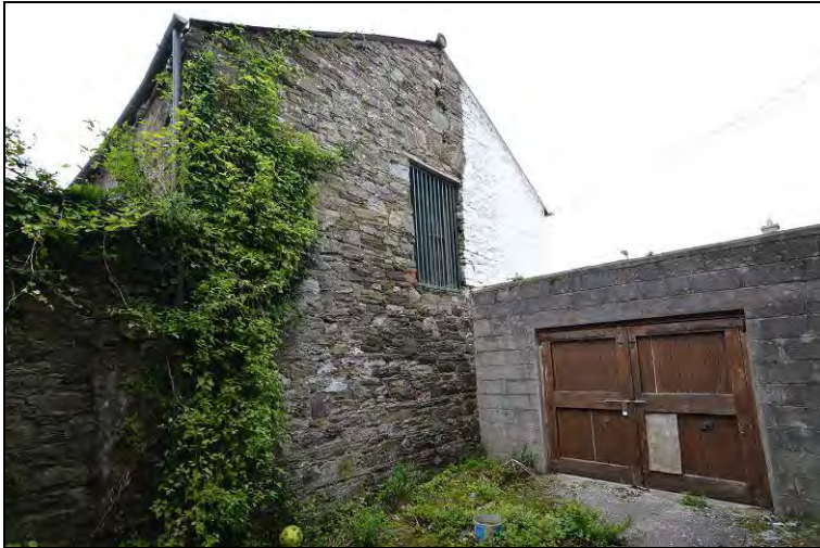
Photograph 9: Gabled east elevation of the Soup-Kitchen.
