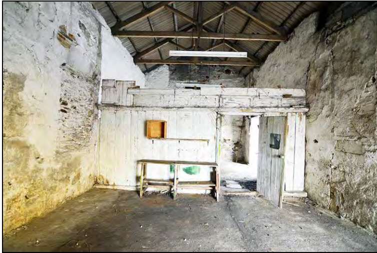
Photograph 15: Timber partition, viewed from the eastern space.
