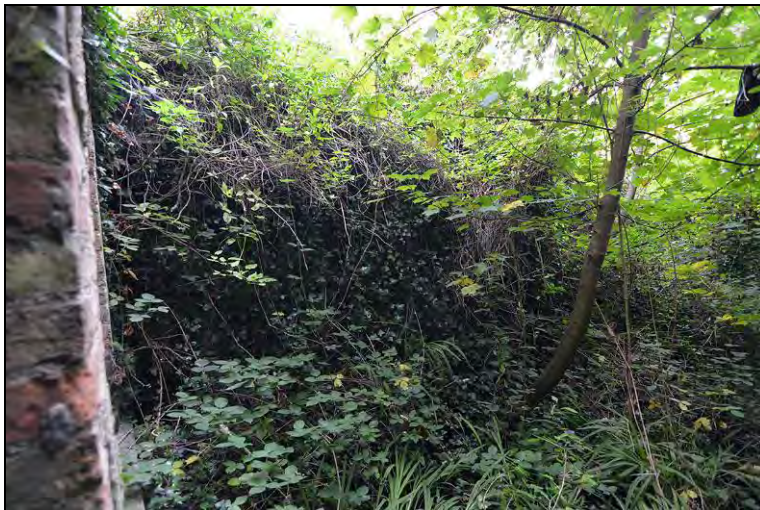
Photograph 10: Overgrown rear yard to Courthouse, looking towards upstanding Town Wall.
