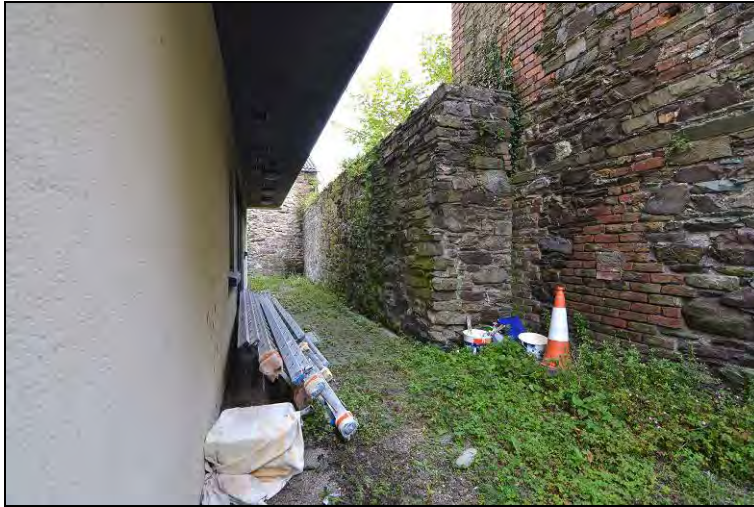
Photograph 6: West facing elevation of Town Wall to rear of Courthouse.
