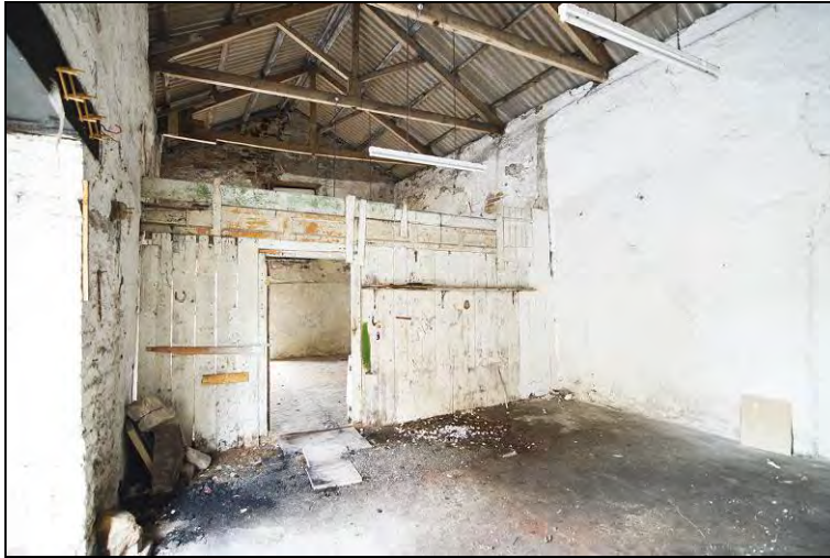
Photograph 18: View of the western space, looking southeast.
