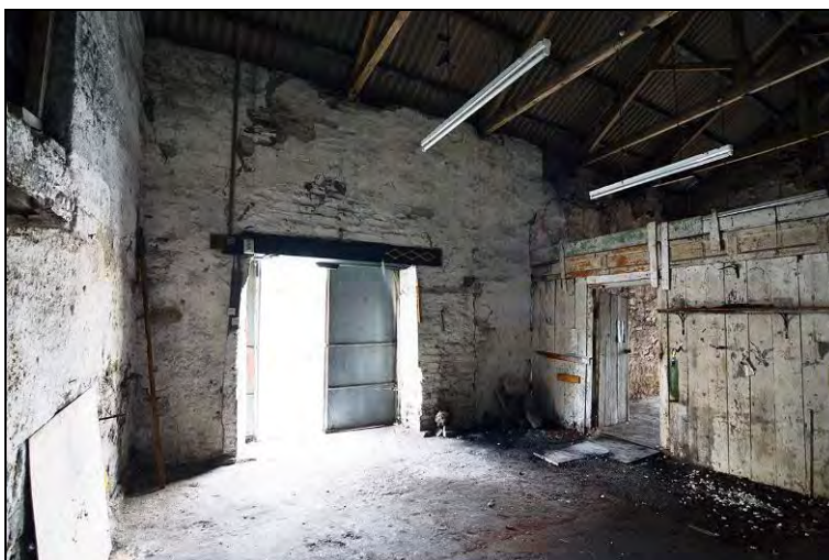
Photograph 20: View of the western space, looking northeast.
