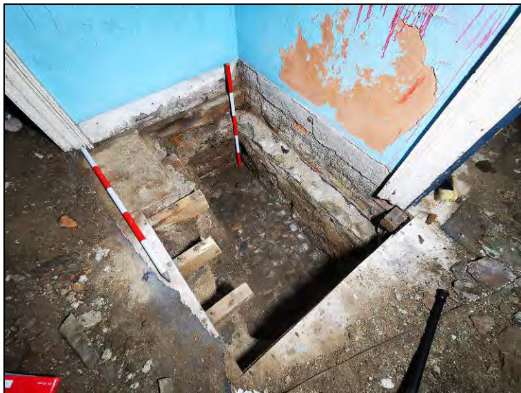
Photograph 21: Test Pit A, looking northeast.
