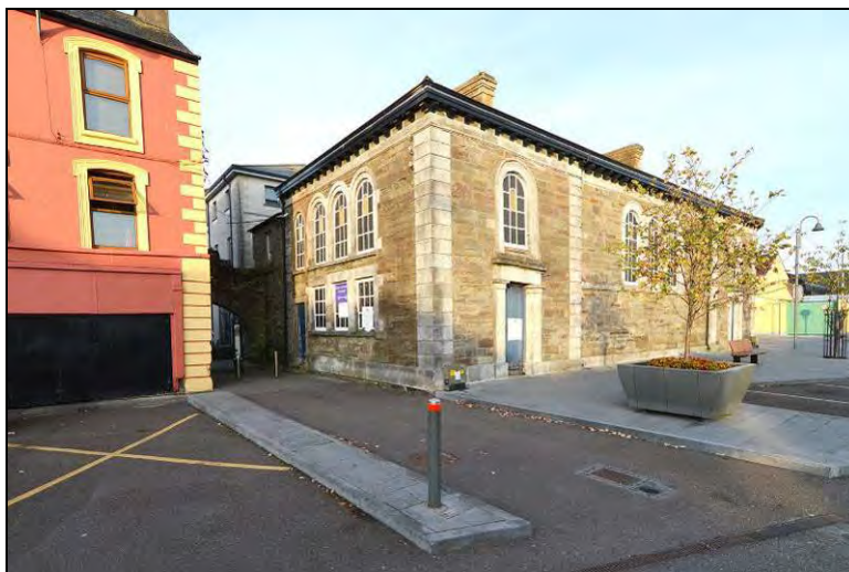
Photograph 5: Southeast corner of the Courthouse, and Quay Lane.
