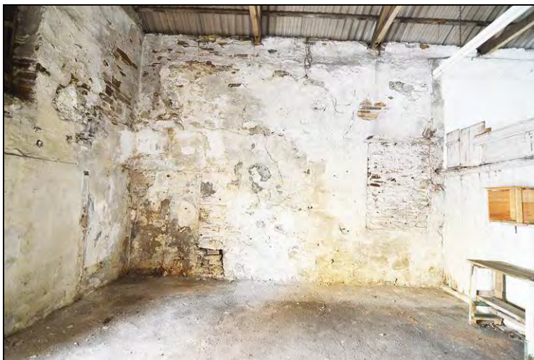
Photograph 14: South elevation of the eastern space.
