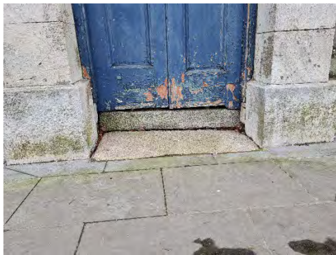
5. Courthouse front door threshold
