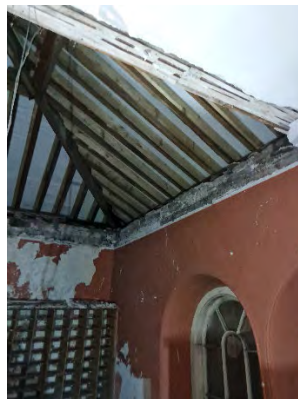
6. Roof of courthouse
