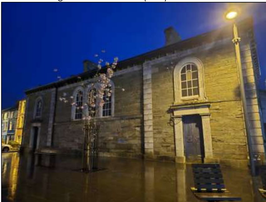
Plate 3 Existing main courthouse (front) which is illuminated - a likely deterrent for bats.
