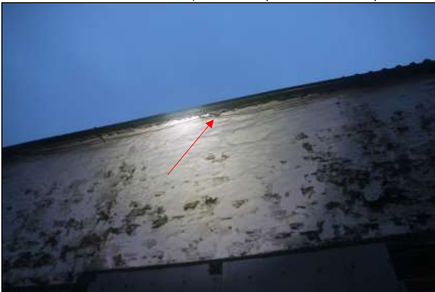
Plate 9 View of potential access point under the corrugated roof.
