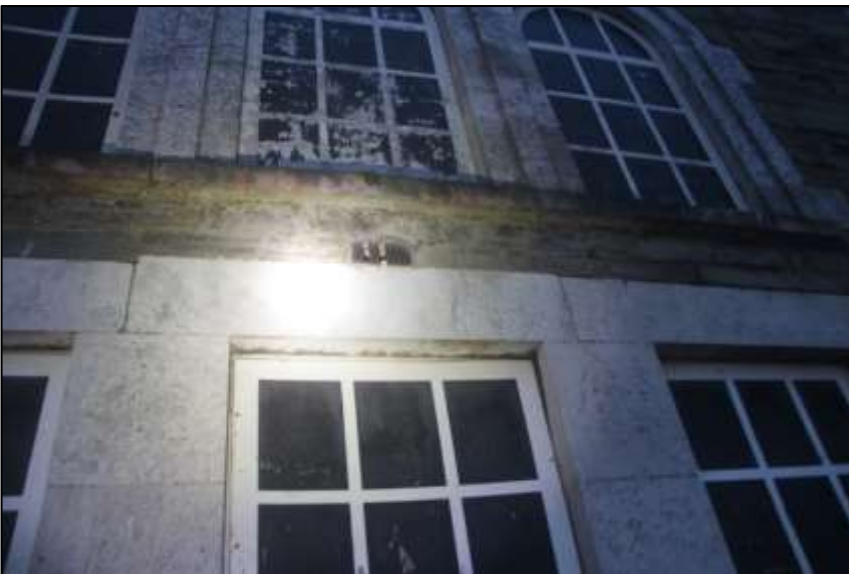
Plate 5 Existing main courthouse (side), torch showing a potential roost feature/entry point.
