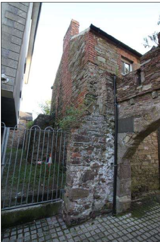
• Fig 33 &34. Southern gable and SW corner with rubble walls and poor pointing, and Cromwells Arch.
