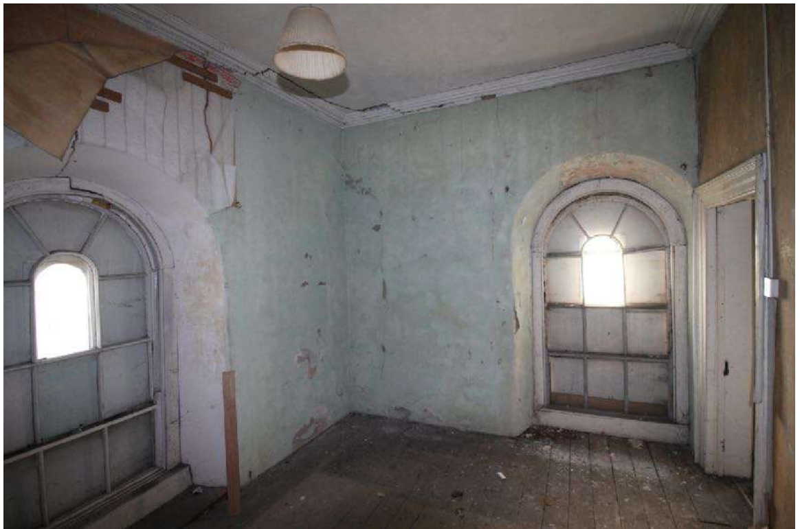
• Fig 91. Room. 16 First floor office off landing.
