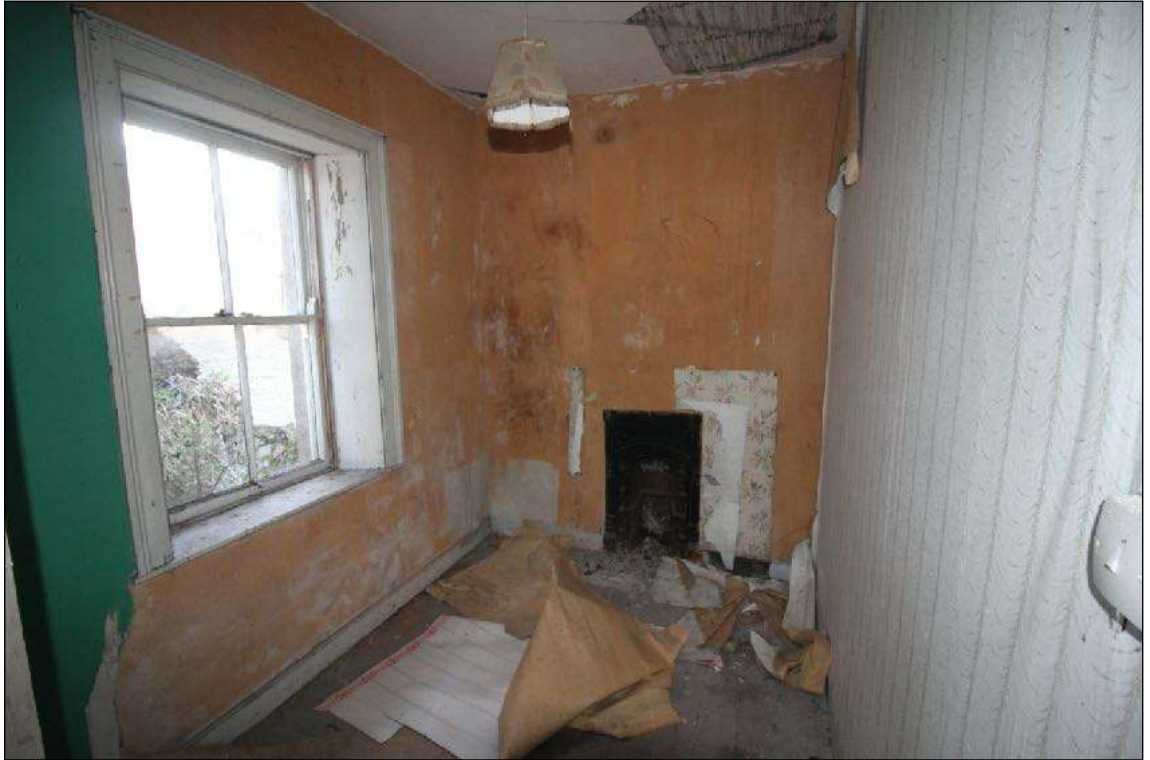
• Fig 94. Room. 17 First floor office off landing.
