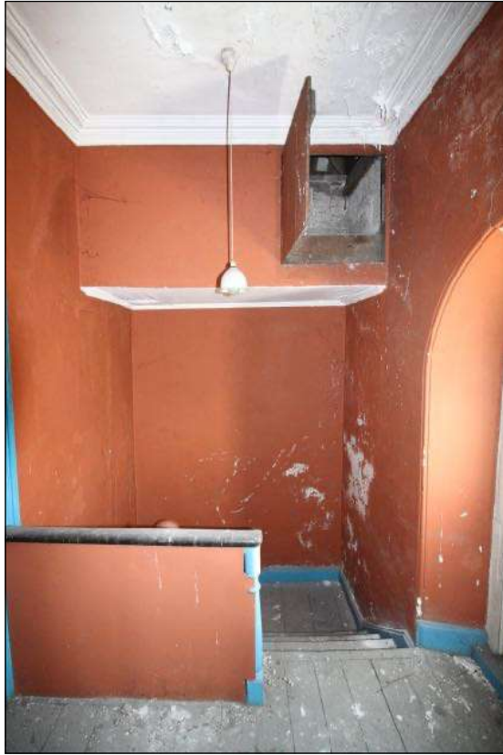
• Fig 98. Room. 19 Main front stairs landing.
