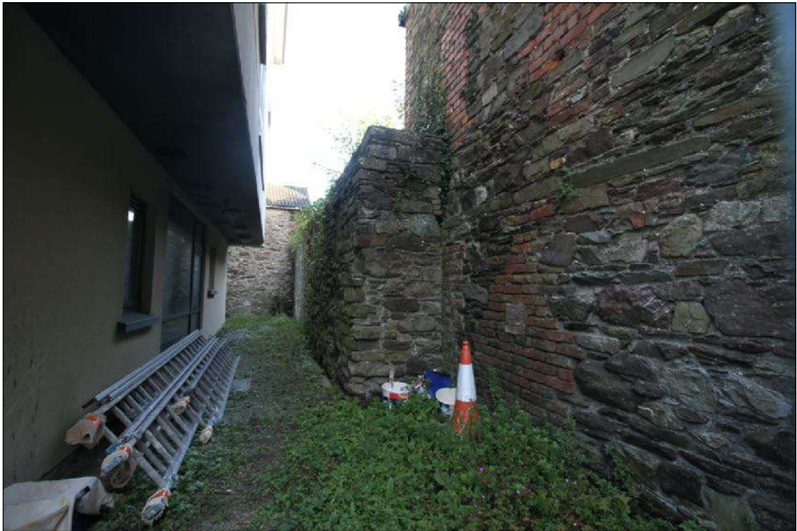
• Fig 37. South West elevation and remains of old City wall.
