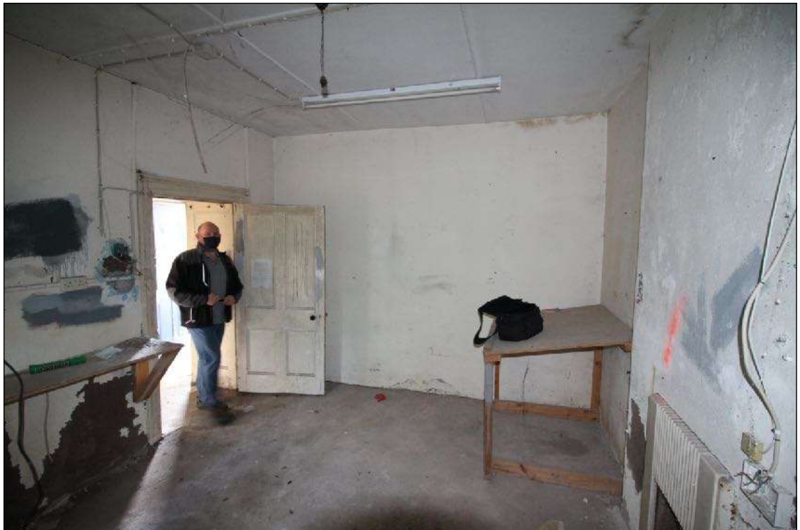
• Fig 58. Room No.5 Rear yard Entrance (former kitchen).
