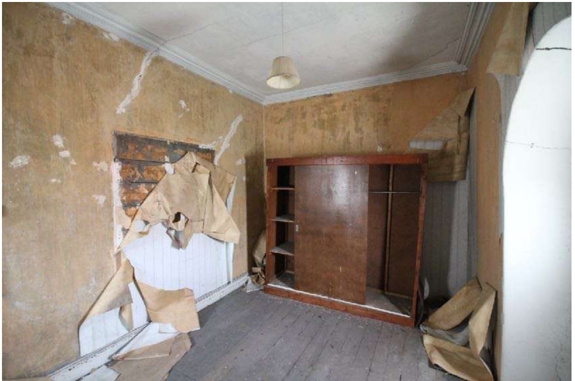
• Fig 92. Room. 16 First floor office off landing.
