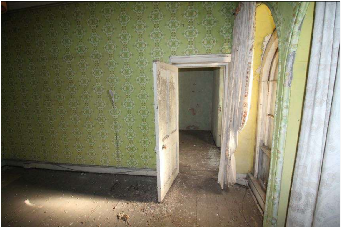
• Fig 89. Room. 15 First floor office off landing.
