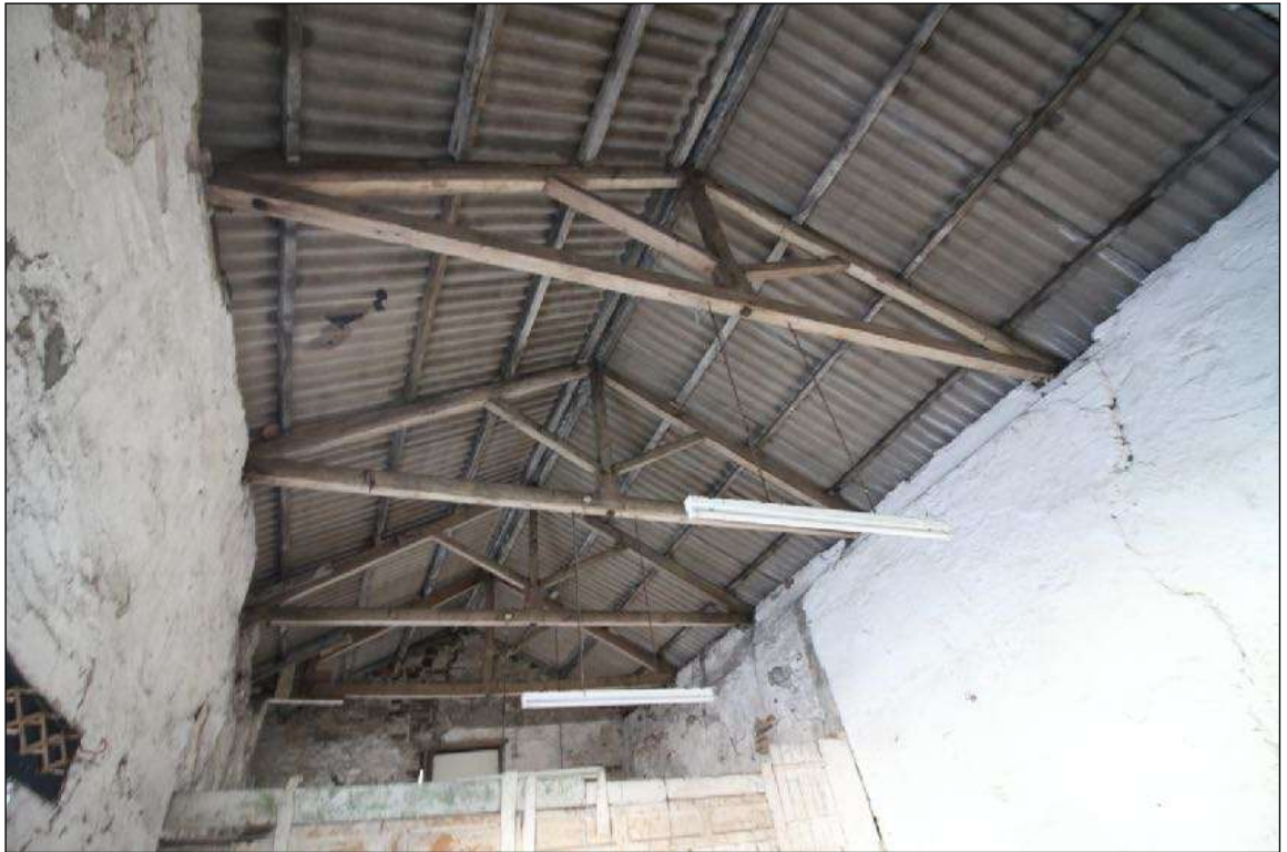
• Fig 119. Roof structure and corrugated sheets above.
