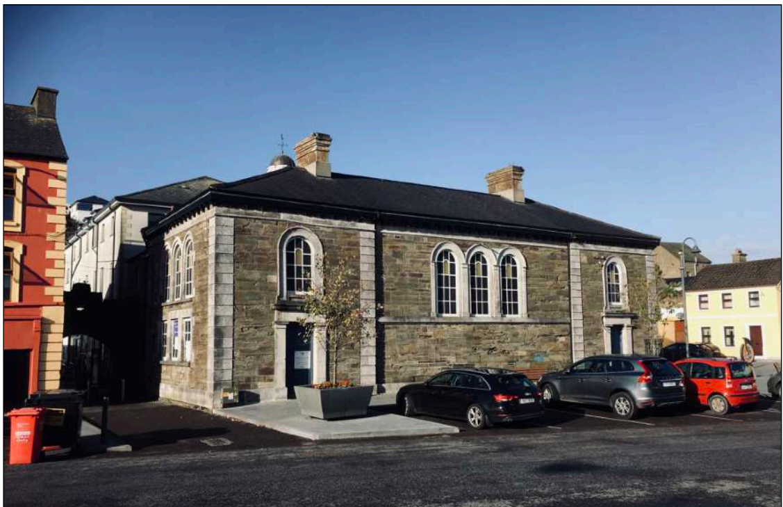
• Fig 18. Courthouse Re-roofed in 2014 by OPW.
