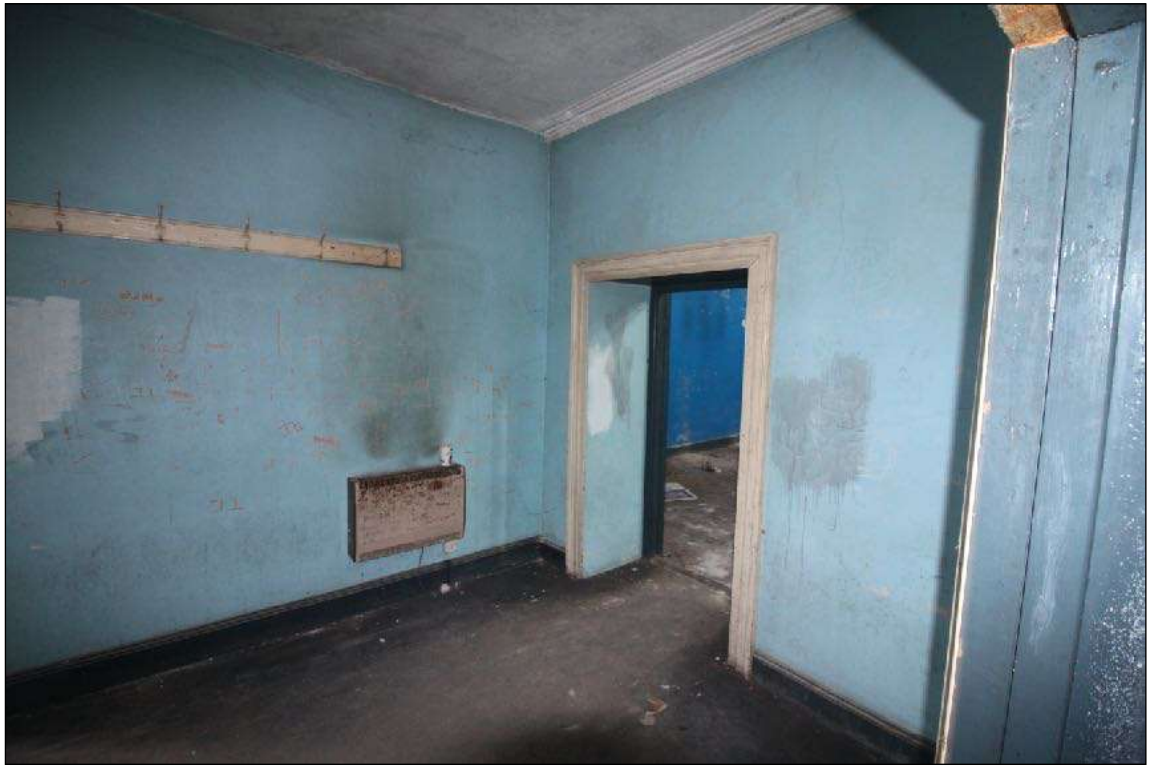
• Fig 52- 53. Room 23. Office.
