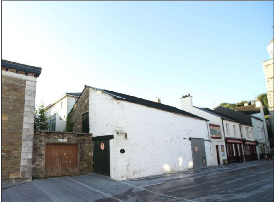
• Fig 109. Side of door Kitchen building, facing Courthouse rear, partially.
