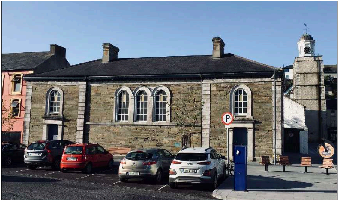
• Fig 17. Courthouse Re-roofed in 2014 by OPW.
