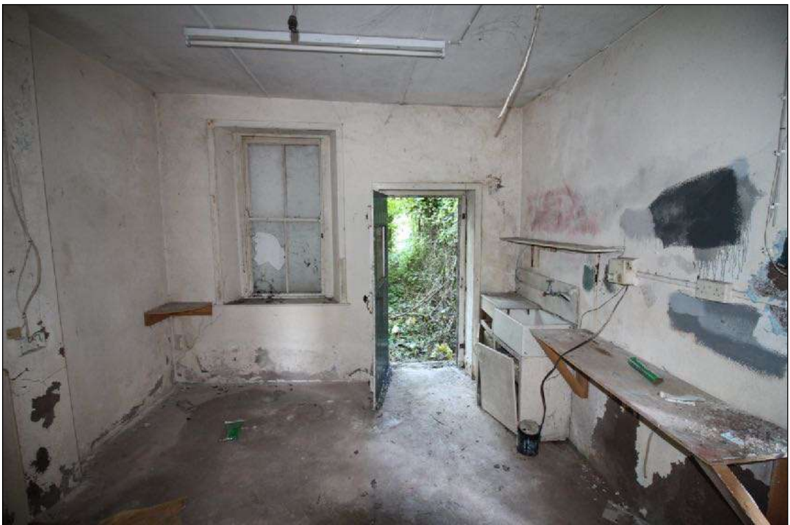
• Fig 59. Room No.5 Rear yard Entrance.
