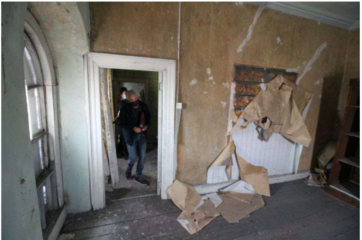
• Fig 93. Room. 16 First floor office off landing.
