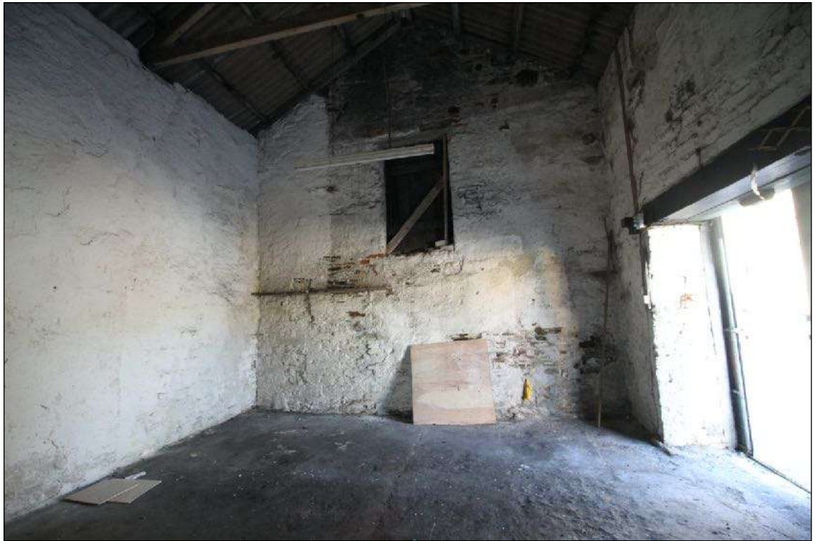
• Fig 121. Door No.2. Access door above to adjoining?
