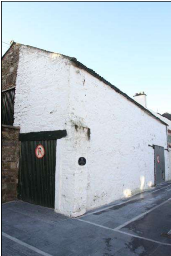
• Fig 112. Corner of Soup kitchen building and second entrance.
