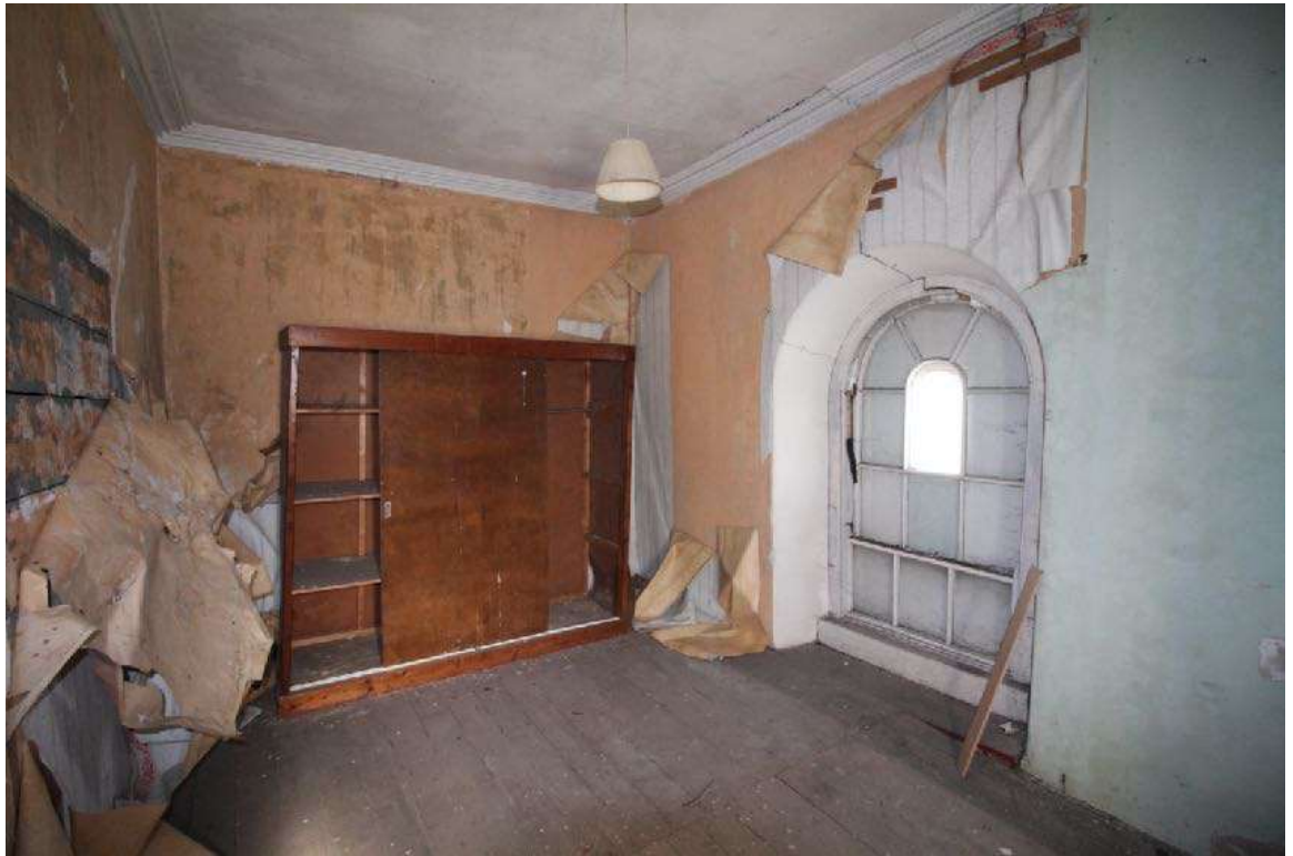
• Fig 90. Room. 16 First floor office off landing.
