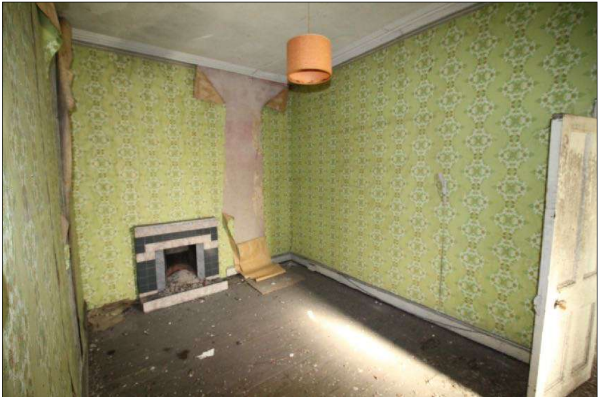
• Fig 85. Room. 15 First floor office off landing.
