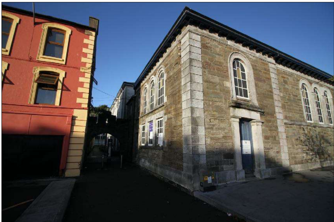
• Fig 36. South Eastern corner.
