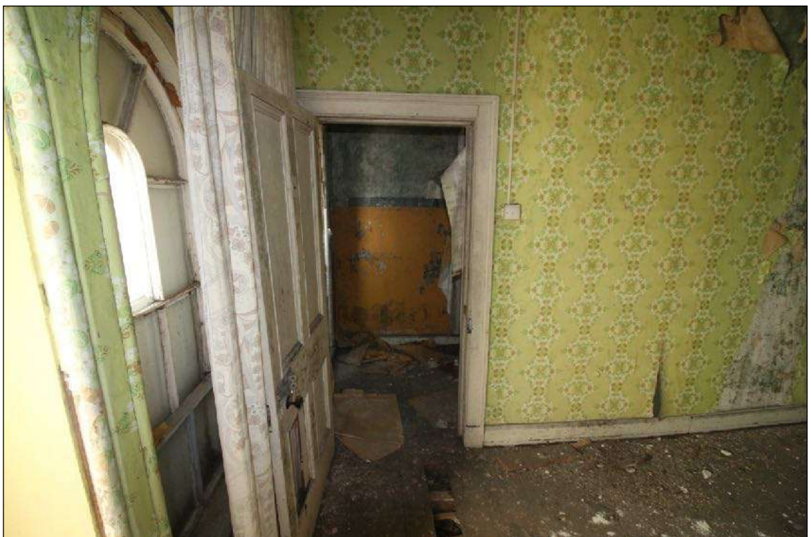
• Fig 86. Room. 15 First floor office off landing.
