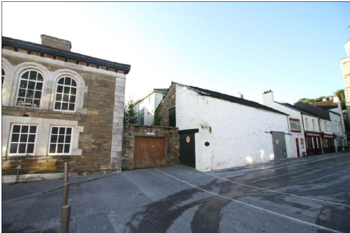
• Fig 40. Link between Courthouse and Soup kitchen.
