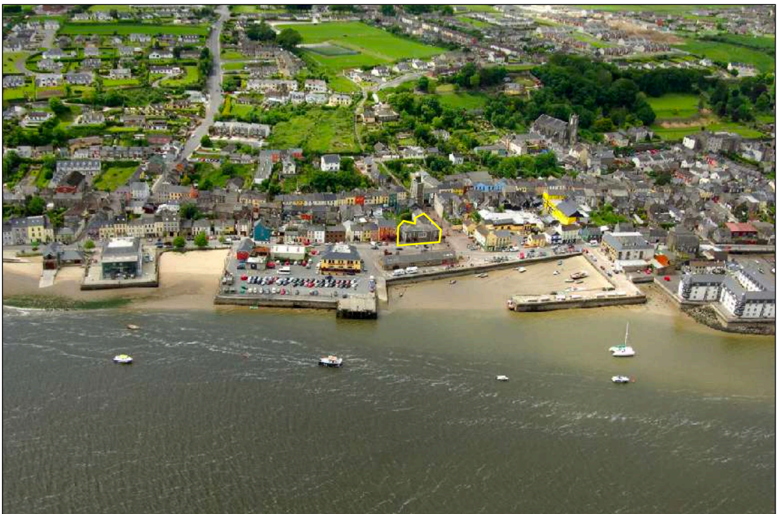
• Fig 4. Site from above.
