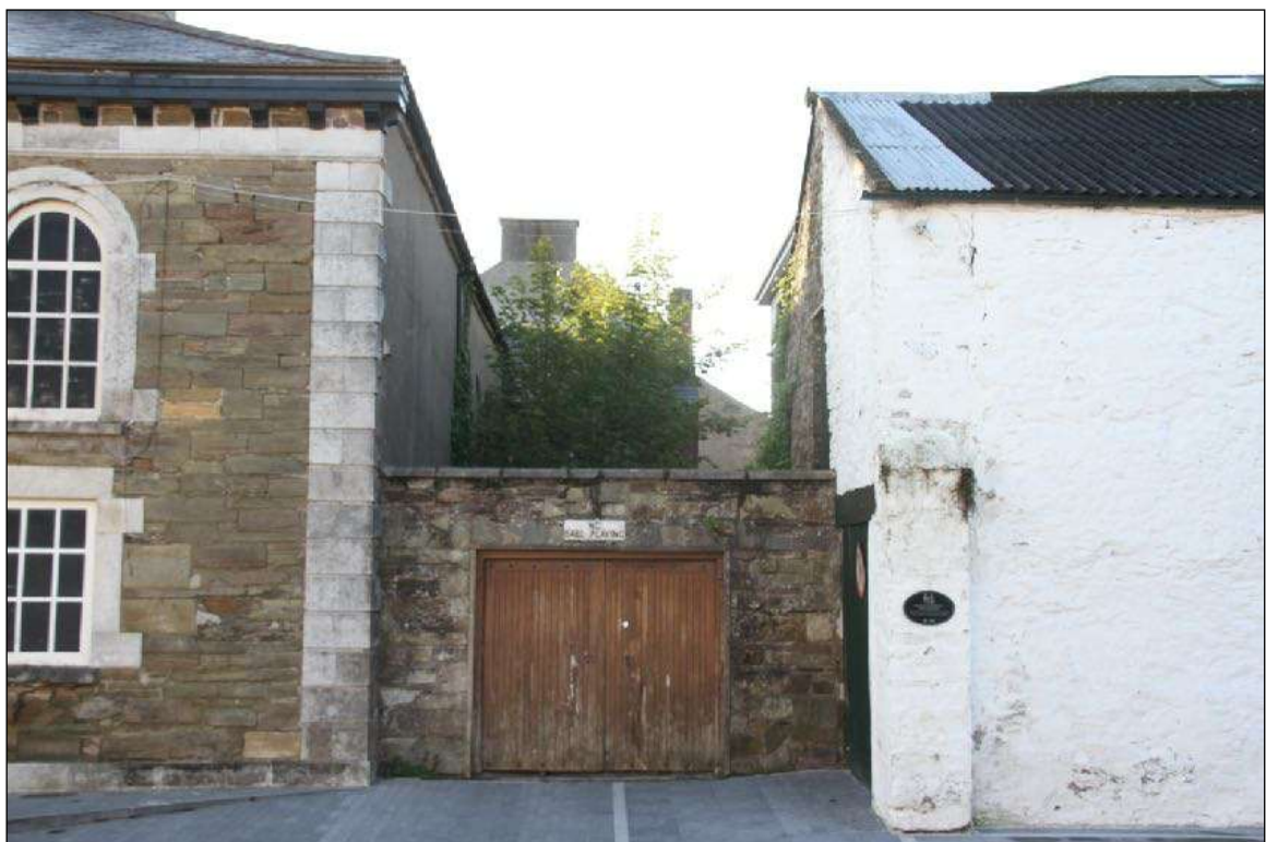
• Fig 24. Linking wall between Courthouse and Soup kitchen.
