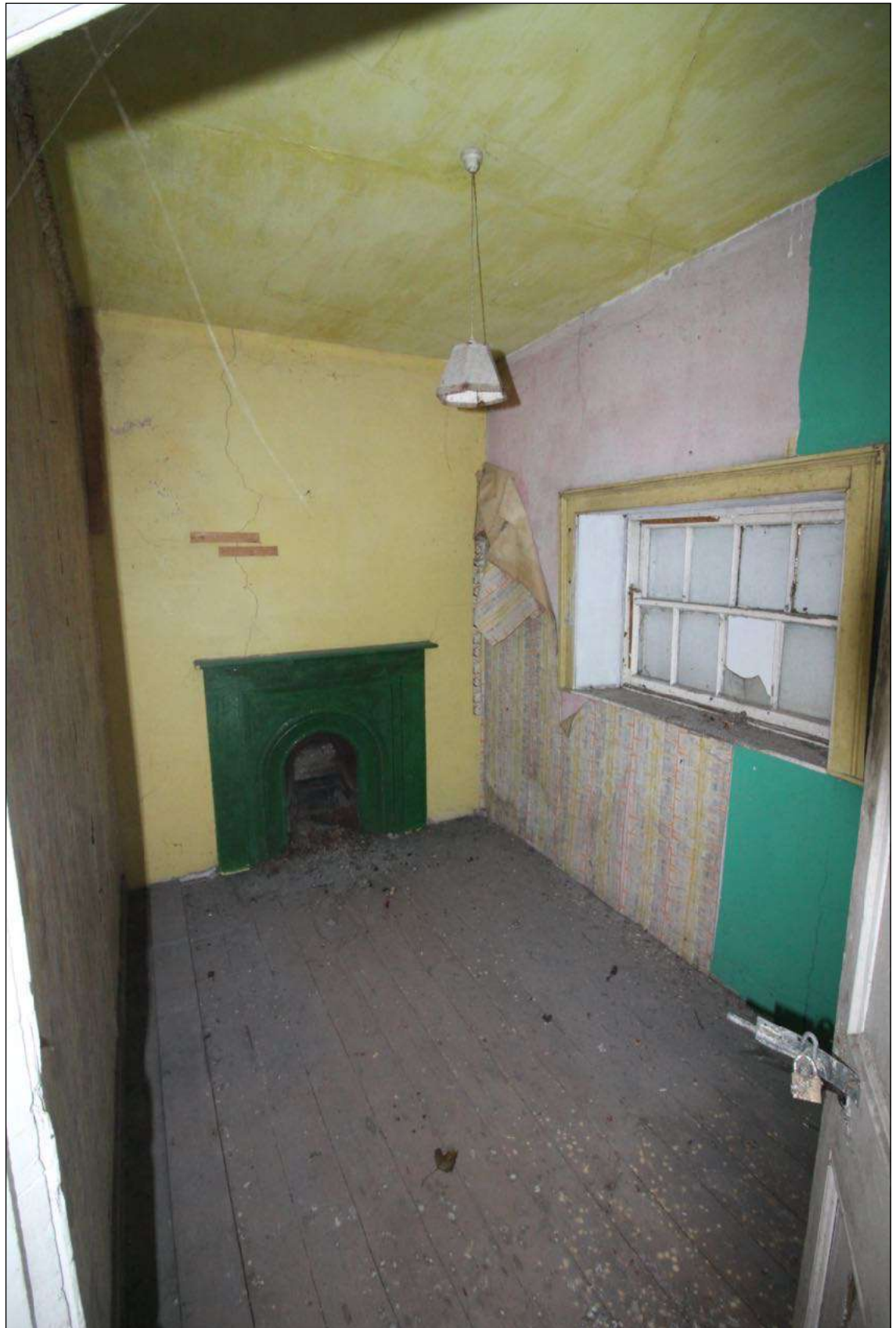
• Fig 97. Room. 18 First floor office off landing.
