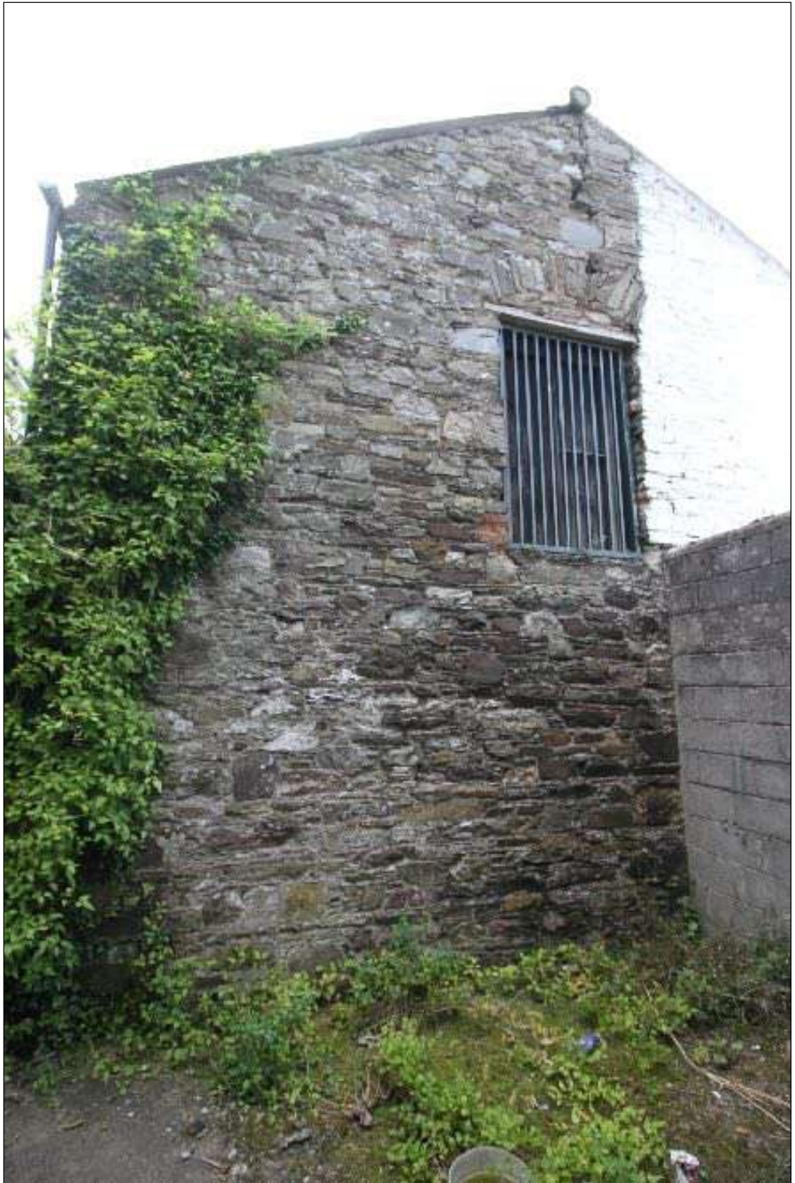
• Fig 108. Side of door Kitchen building, facing Courthouse rear.
