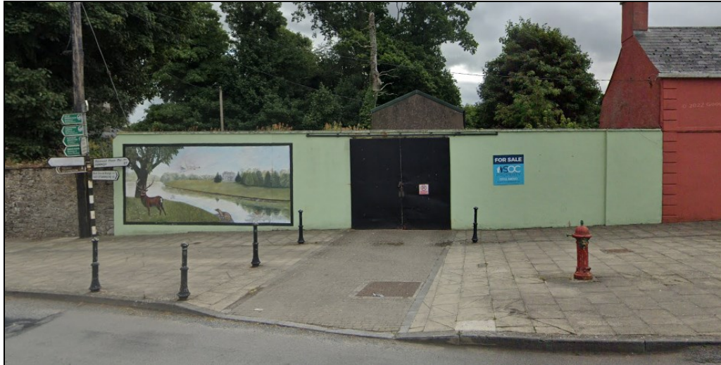
Figure 2: Existing Entrance to Proposed Car Park Site
