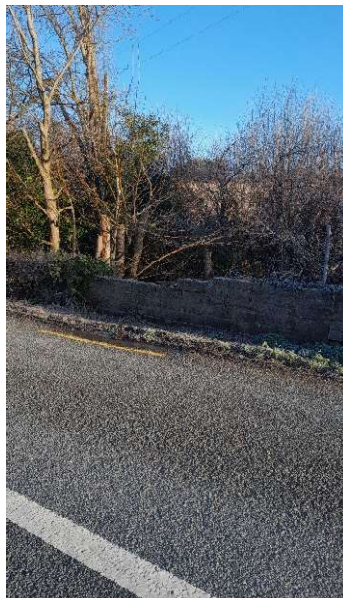
Figure 9 - Parapet Walls of Bridge 1
