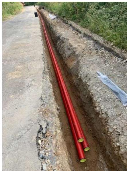
Figure 5 - Typical Underground Duct Installation
