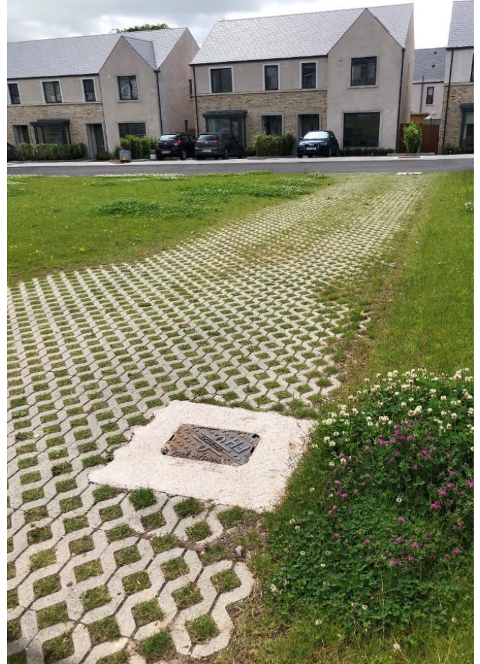
Fig 6.6 Harpers Creek, Glounthaune – Greenspace serving multifunctional purpose (service vehicle access)
