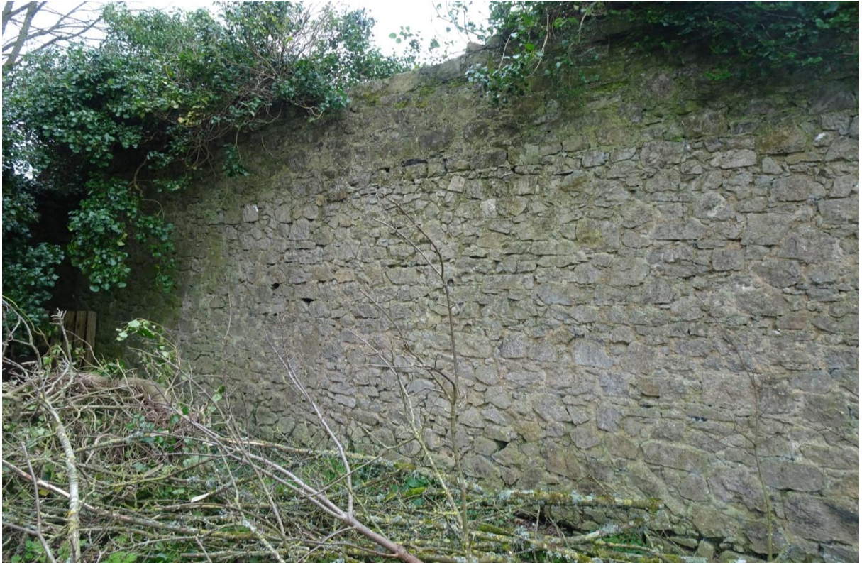
Plate 12 The east boundary wall. Note lack of coursing lines in contrast to the north wall.
