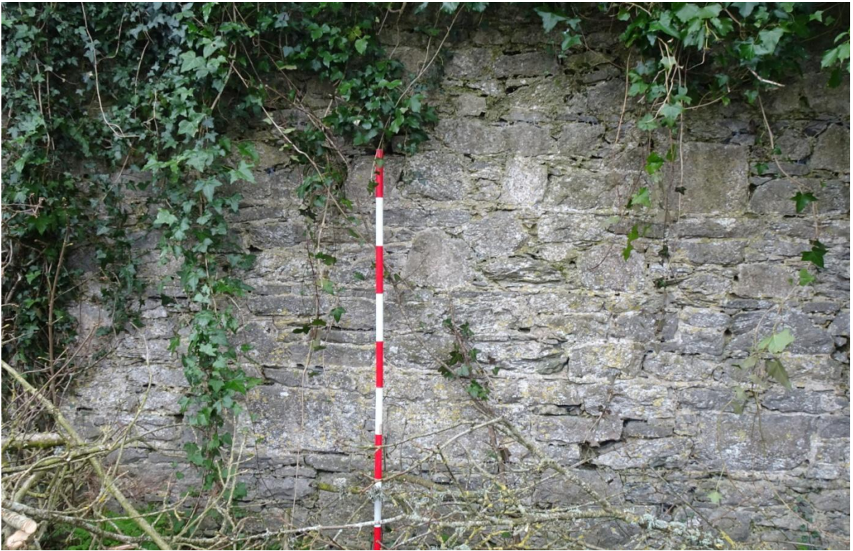
Plate 11 North boundary wall, detailed view of masonry coursing.
