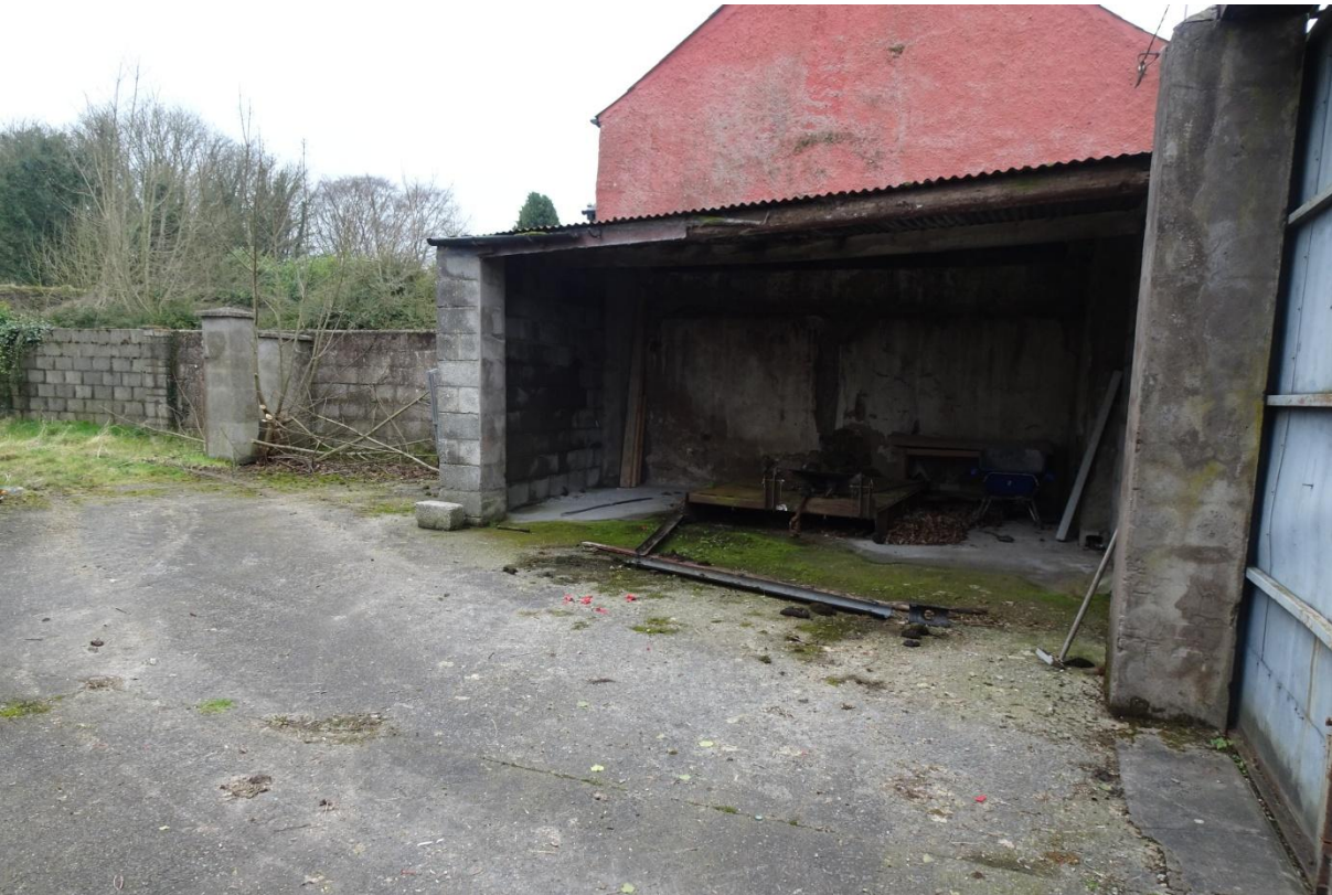
Plate 4 Storage shed in southwest corner of site.
