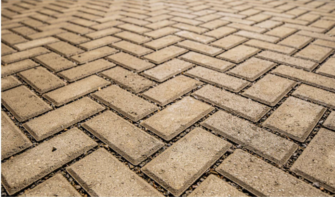
Figure 11: Example of permeable paving.
