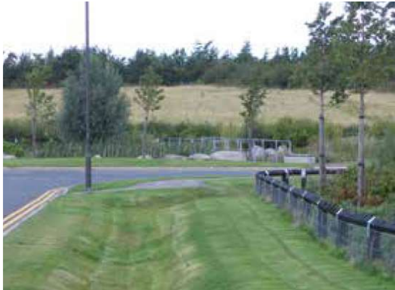
Figure 10: Example of roadside swale from the CIRIA SuDS Manual (C753)
