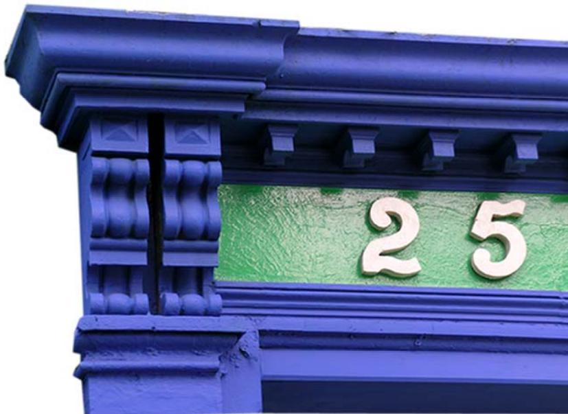
Retain Important Exterior Architectural Features
