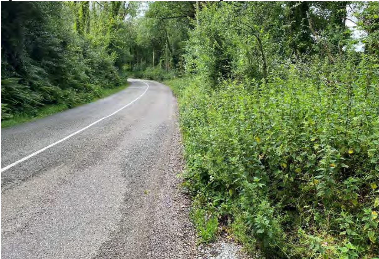
Figure 4: View Westwards from the Site Entrance along the L-6090
