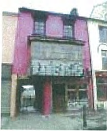
RPS 52 William's Lane 'Arch under Gearagh Bar'
