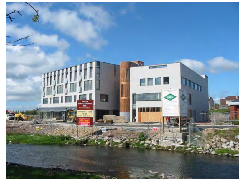
FIGURE 3.9: WATER'S EDGE DEVELOPMENT UNDER CONSTRUCTION (PHASE ONE)
