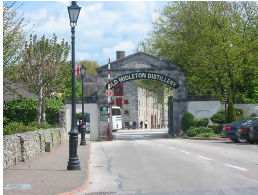
FIGURE 3.5: ENTRANCE TO MIDLETON DISTILLERY
