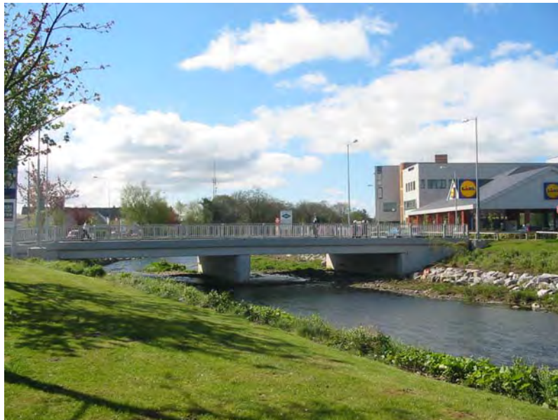
FIGURE 3.10: NEW BRIDGE CONSTRUCTED AS PART OF WATER'S EDGE AND LIDL DEVELOPMENT
