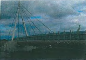
Pedestrian Links over Ilen River
