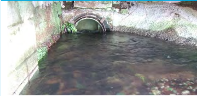
Inlet to Irish Rail Siphon
