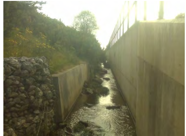
Rail channel at downstream end
