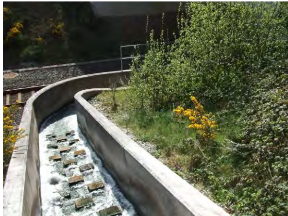
Rail channel at upstream end (cascade)
