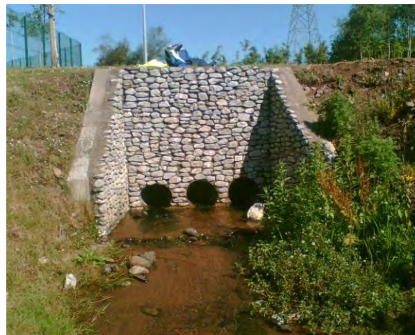
2CA1_1176_US.jpg – downstream face
