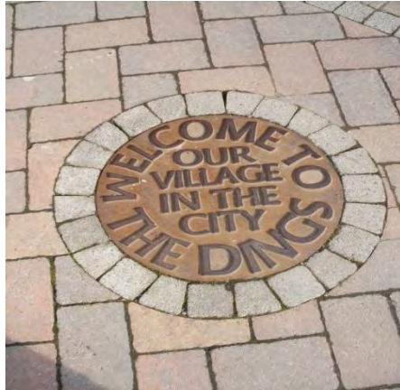
Manhole cover with local personalisation
