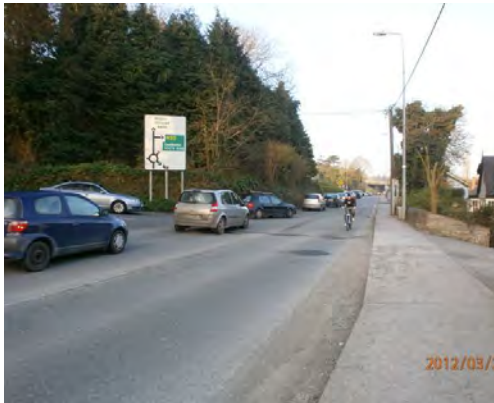
Picture 1: Standing on Rochestown Rd facing west towards St Patrick's Roundabout
