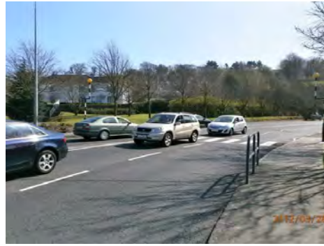
Ped Crossing on Carrigaline Rd arm of Roudabout
