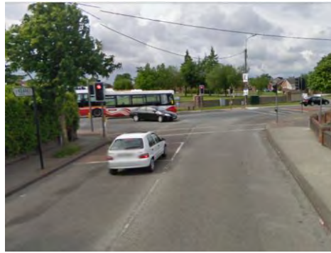
Looking north towards Grange Rd
