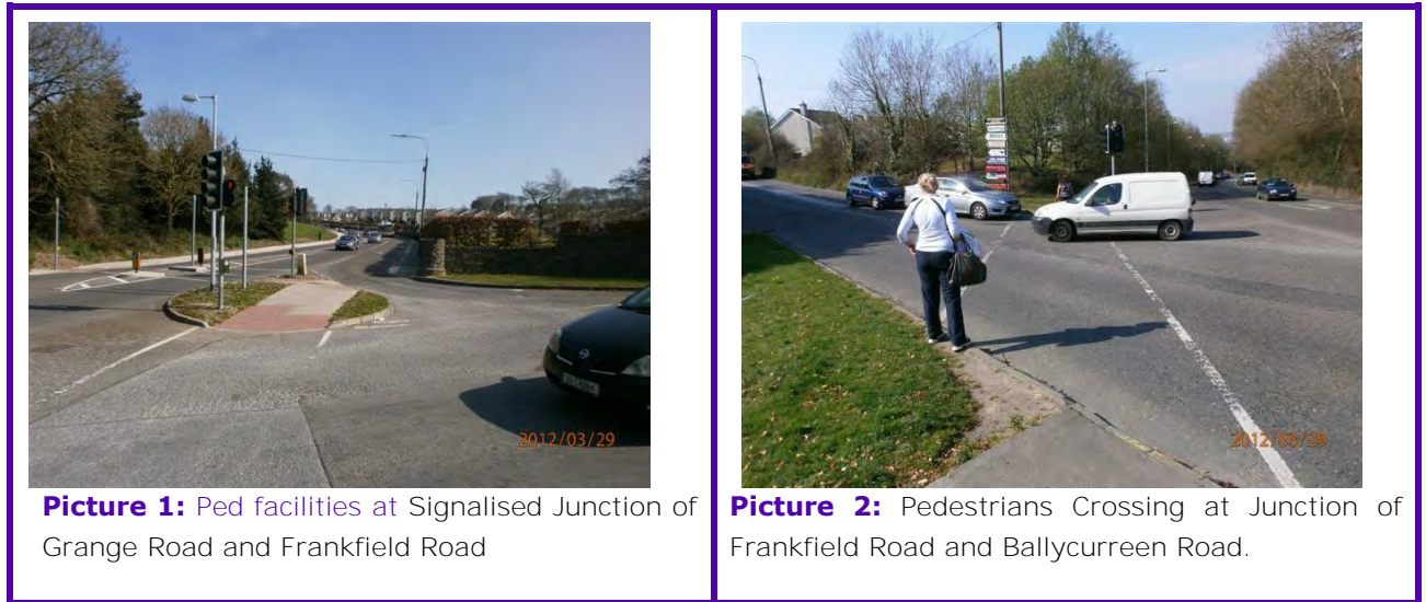
Figure 5-34 Grange / Frankfield Conurbation Pedestrian Facilities
