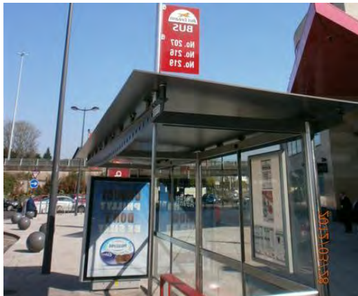
Picture 2: Sheltered Bus Stop at Douglas Village Shopping Centre.
