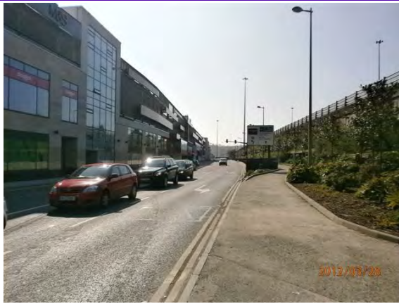
Picture 3: New Link Road facing west
