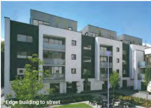
Edge building to street
