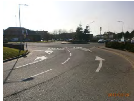
Standing at exit from Douglas Court facing west towards Roundabout.
