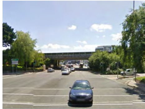
Standing on Douglas Rd facing south towards junction with off ramp.
