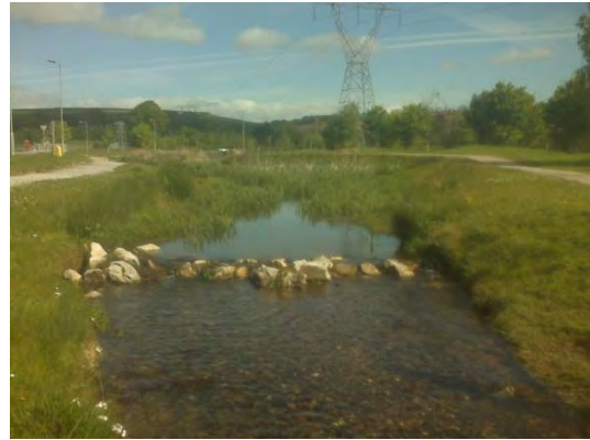
pond / sedimentation area upstream of rail siphon
