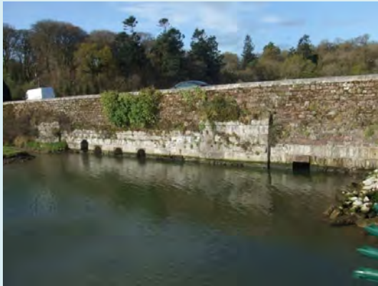
Upstream face of Slatty Bridge
