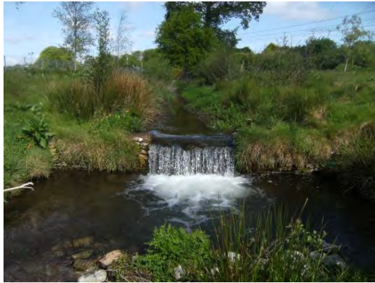
One of two similar weirs upstream of the rail line
