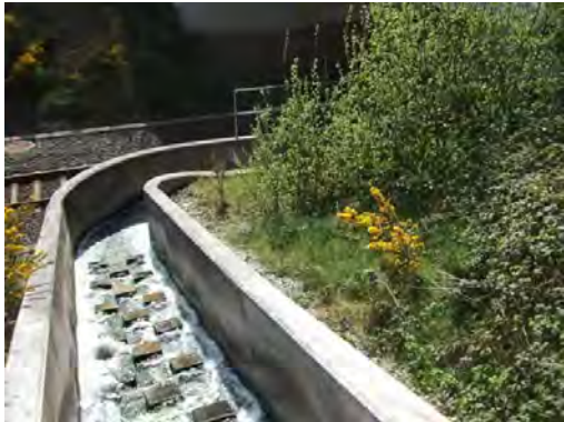
Rail channel at upstream end (cascade)
