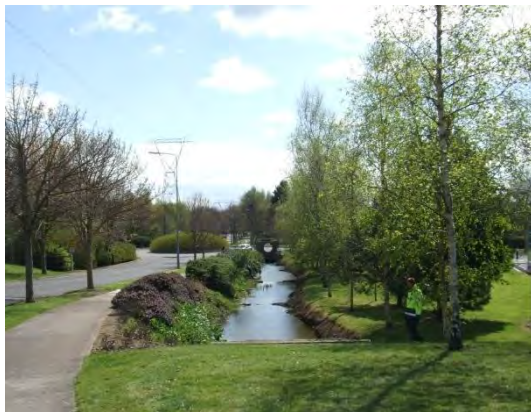
Series of weirs downstream of rail line (looking downstream)
