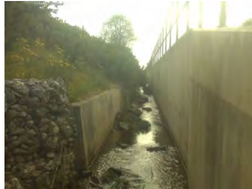
Rail channel at downstream end
