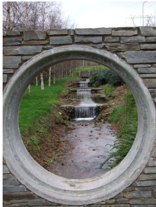
Same series of weirs downstream of rail line (looking upstream)
