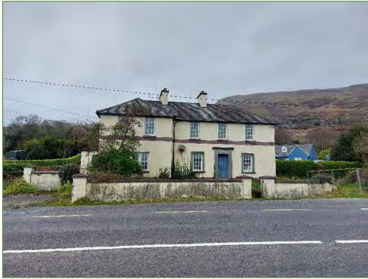
A1. View of the existing building at the proposed site, previously occupied as Adrigole Garda Station, photographed from the R572.
