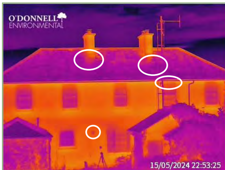
Plate 2.4 Alternative viewshed of thermal camera covering the rear aspect of the former Garda Station. Identified potential access/egress points are highlighted in white circles.
