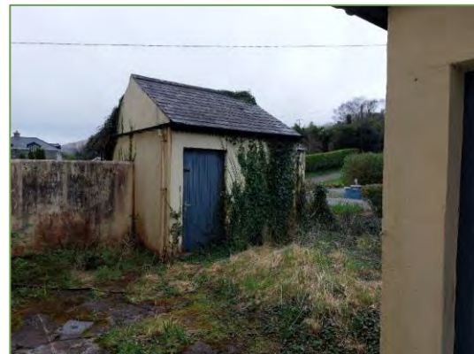
Plate 3.2.2 View overlooking the associated outhouse at the rear of the former Garda Station.
