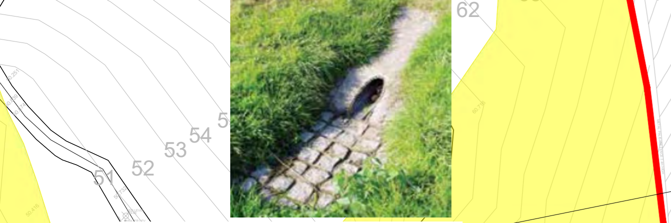
Inlet/Outlet Pipe Opening (300mm Ø pipe) in each of the 5 basins to be constructed with a concrete & cobbled apron to prevent erosion/growth near the pipe opening
