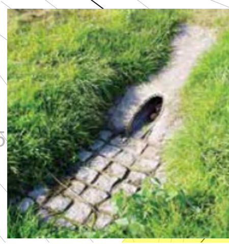
Inlet/Outlet Pipe Opening (300mm Ø pipe) in each of the 5 basins to be constructed with a concrete & cobbled apron to prevent erosion/growth near the pipe opening
