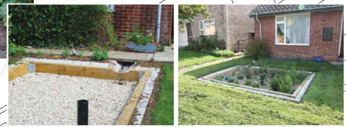
Back Garden - Rain garden Soakaways
