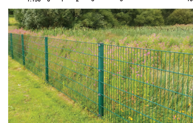
Proposed 1.1m high weld mesh fencing typical to amenity spaces and select attenuation protection.
