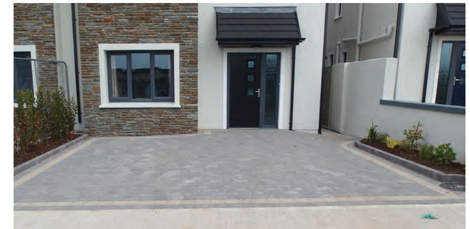
Image of a driveway paved in select coloured concrete unit pavers with planting buffers and rendered boundary walls.
