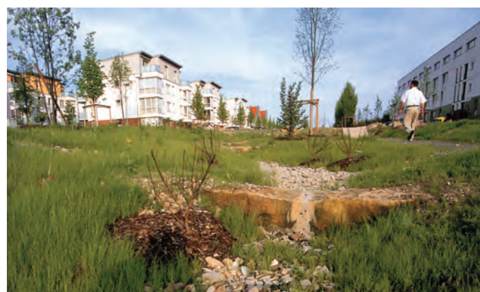
Example of a swale prior to discharge at the attenuation basin. The SuDS swale will typically appear damp or dry.
