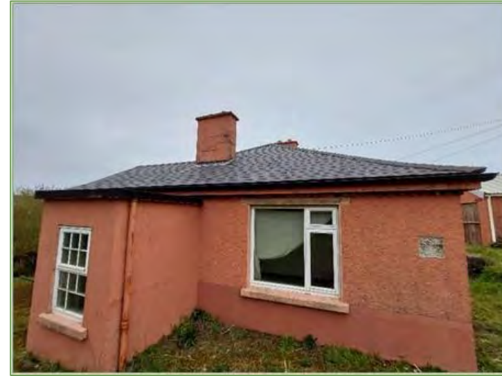
A4. View of the western façade of the existing main building.
