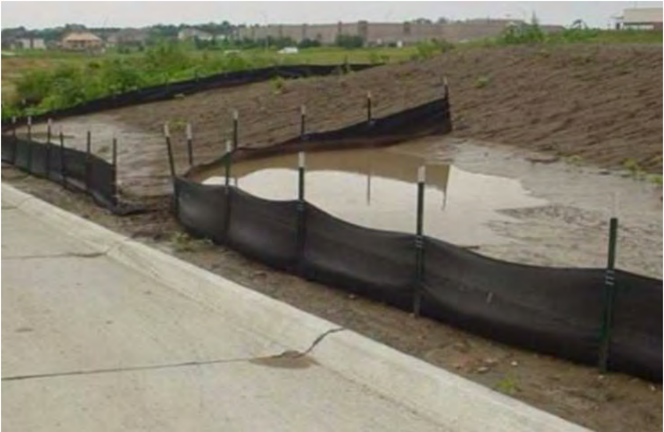
Figure 4 - Typical Silt Fencing Arrangement
