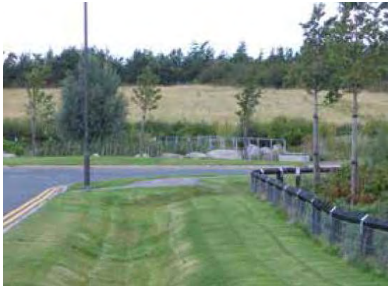
Figure 11: Example of roadside swale from the CIRIA SuDS Manual (C753)
