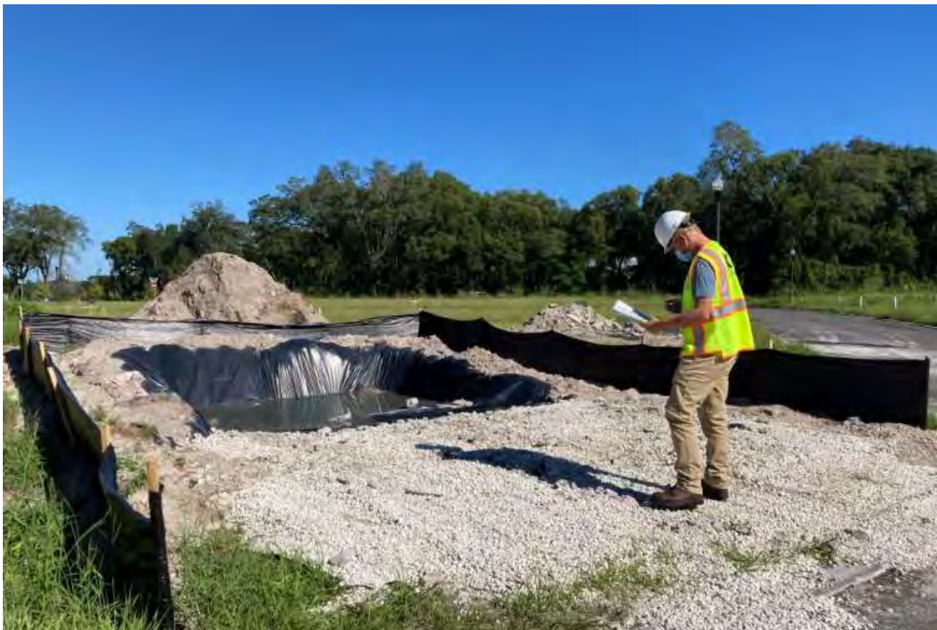
Figure 6 - Concrete Truck Washout Area with Impermeable Liner
