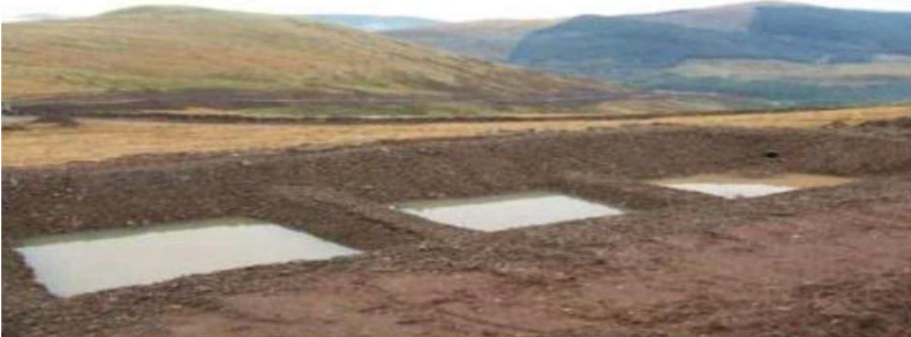
Figure 5 - Settlement Ponds in Series
