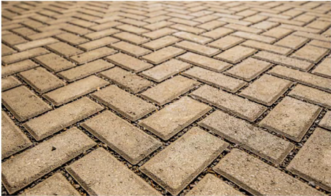
Figure 12: Example of permeable paving.
