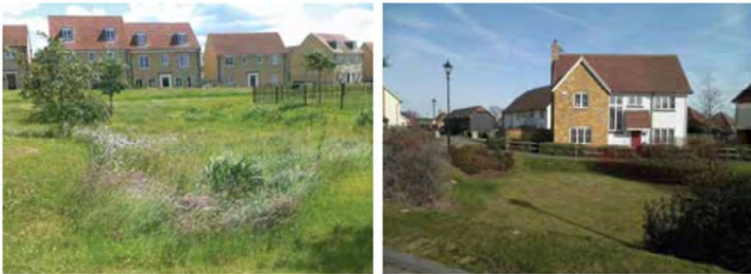
Figure 9: Examples of detention basins by Peterborough City Council in the UK (CIRIA SuDS Manual C753)
