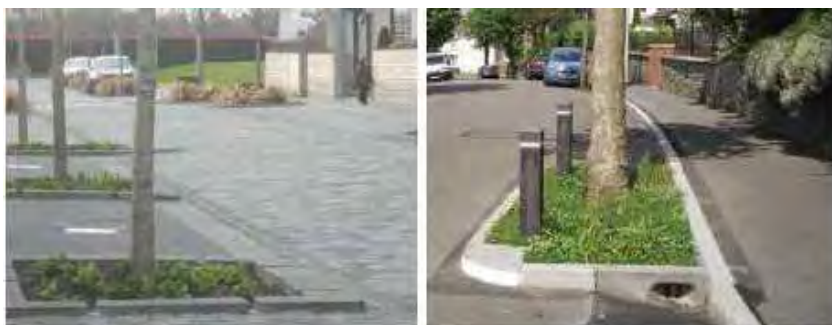
Figure 13: Examples of tree pits in isolated green planters from the CIRIA SuDS Manual
