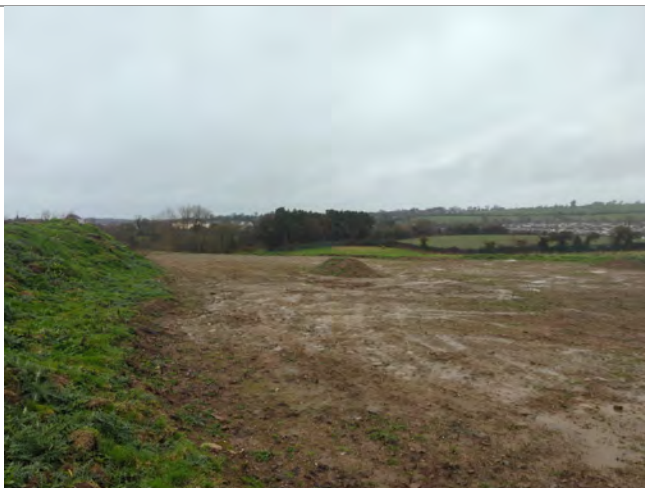
Plate 15. Area of site cleared/bare soil
