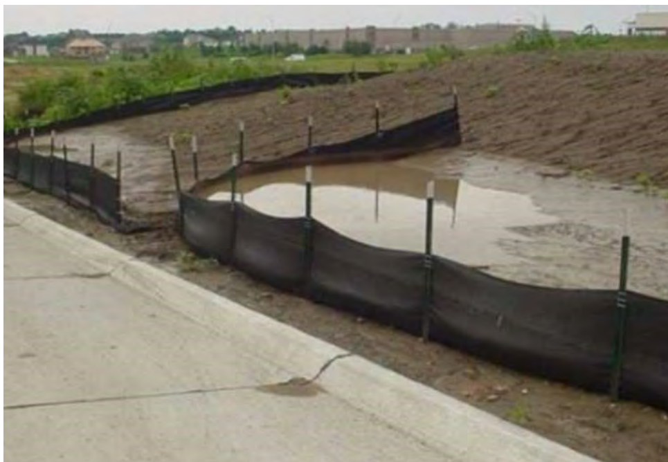
Figure 8 - Typical Silt Fencing Arrangement
