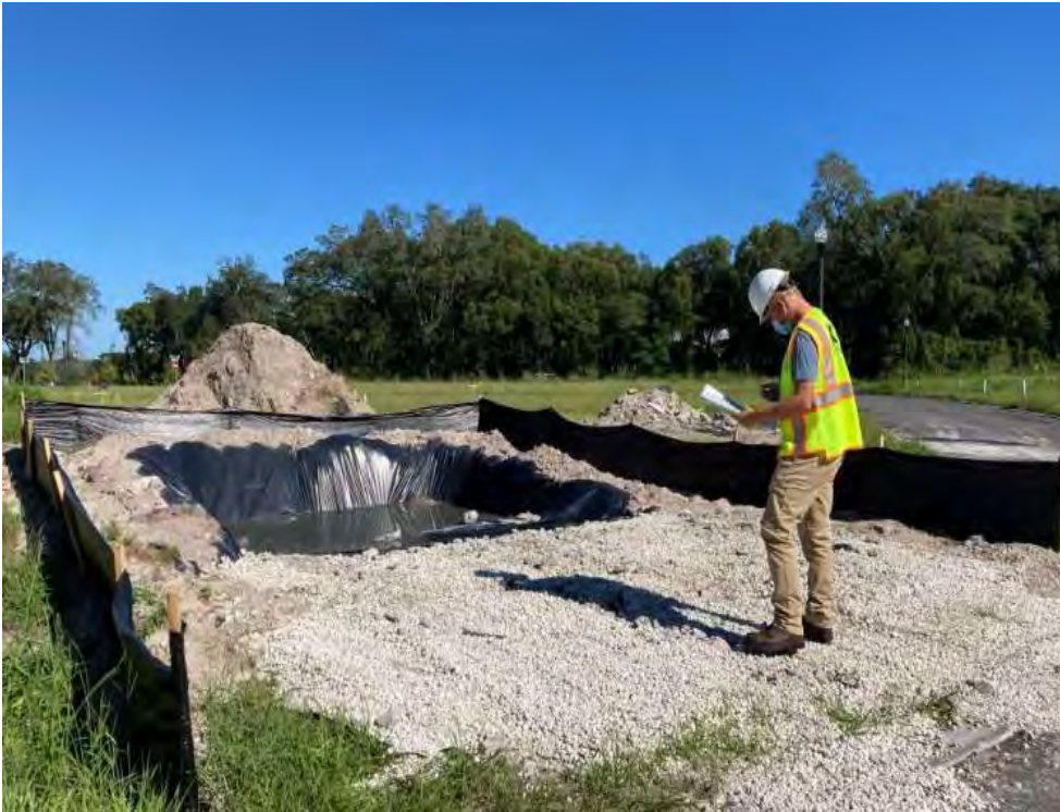
Figure 9. Concrete Truck Washout Area with Impermeable Liner
