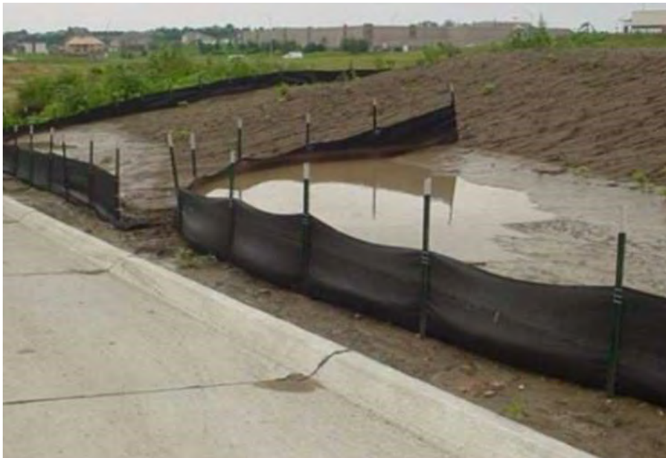
Figure 7 - Typical Silt Fencing Arrangement
