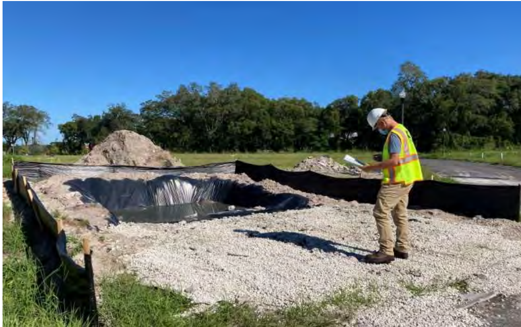
Figure 10. Concrete Truck Washout Area with Impermeable Liner
