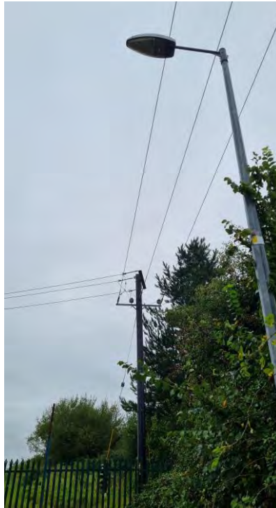
Figure 9: Existing Vegetation/Landscaping, fencing & OH Power lines/Poles at Tie-in
