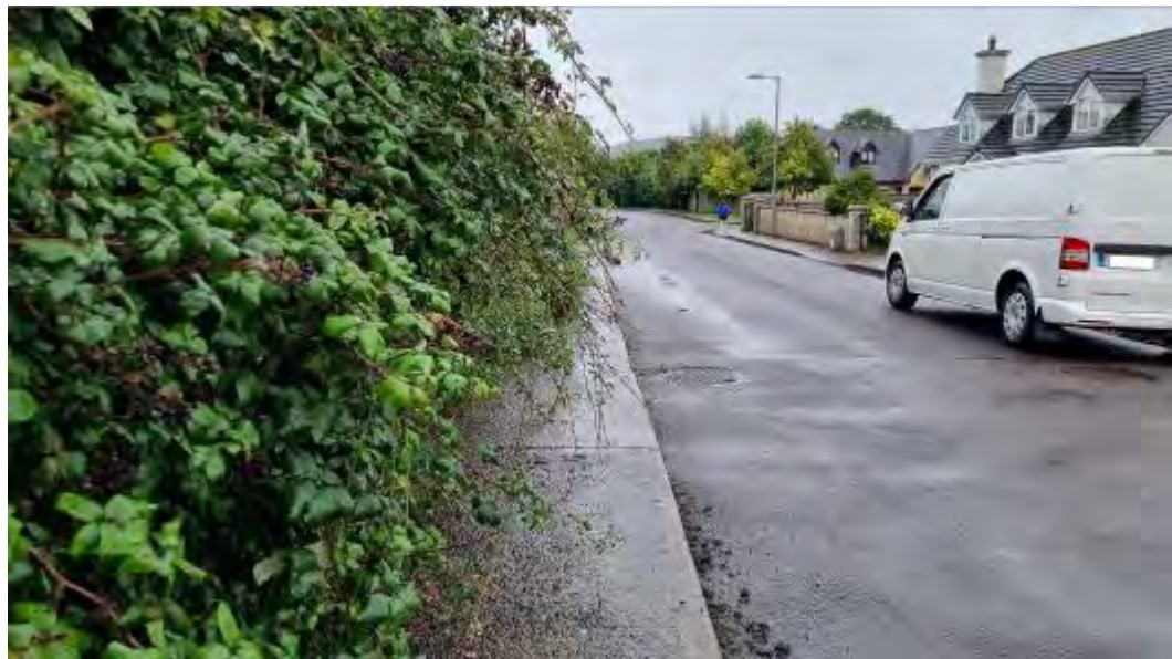
Figure 45: Footway is obstructed by overgrown vegetation at the tie-in
