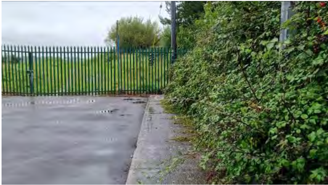
Figure 46: Northbound approach to tie-in showing overgrown vegetation
