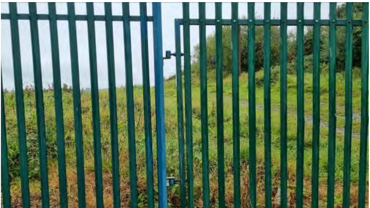
Figure 15: Current Visibility to Left from private Driveway at Tie-In Showing existing fencing and restricted visibility on crest curve
