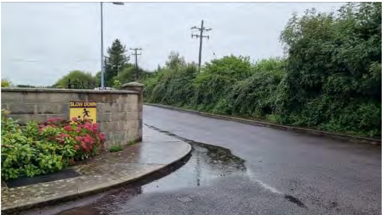
Figure 31: Existing Wall Restricting Visibility to Left from Aldworth Heights (Note Ponding on existing Road)
