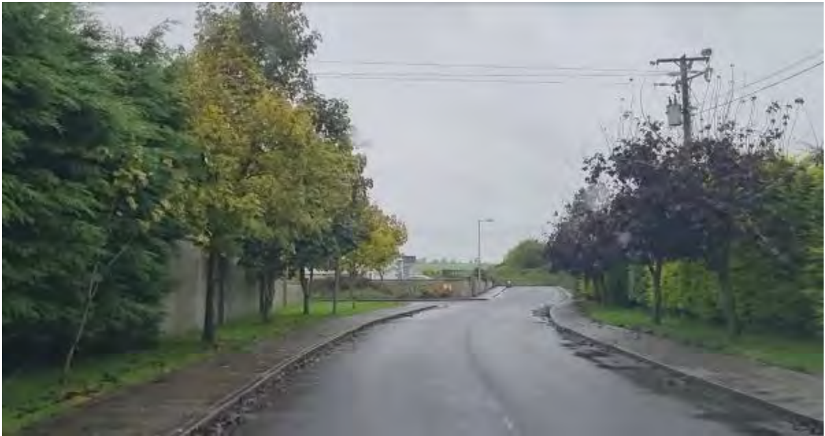
Figure 3: Existing Estate Access road – View Norwards towards Site
