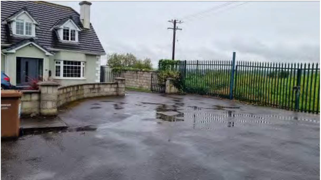
Figure 14: Existing Fencing at Southern Tie-in
