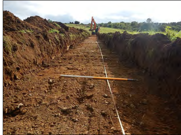
Trench 6, looking S
