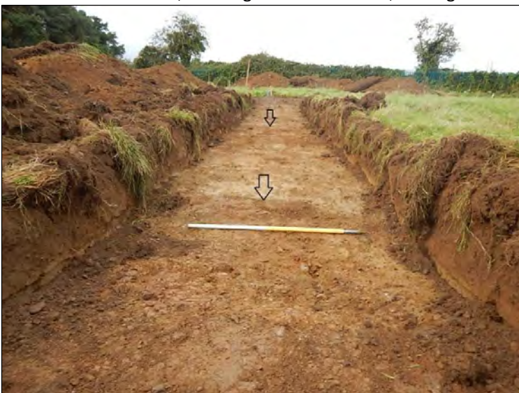
Plate 13: Trench 9, looking NW with F5 in foreground and F6 in background (both indicated by arrows)
