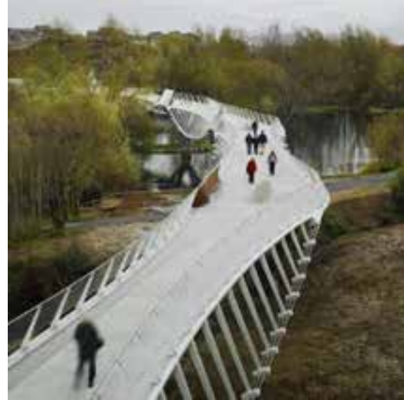
Fig. 5.72 Millennium Bridge, University of Limerick.
