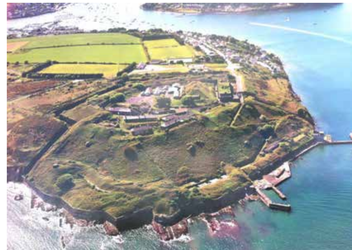
Fig. 2.43 View of Camden Fort. Cork Harbour is punctuated by a number of historic defensive forts around the peninsula.
