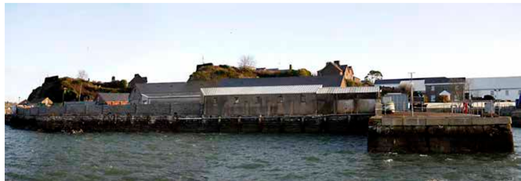
Fig. 3.06 View of island from west showing naval buildings and warehouses at waters edge. The pier is actively used by the Naval Service for dive training due to its convenient close proximity to the deep water channel.
