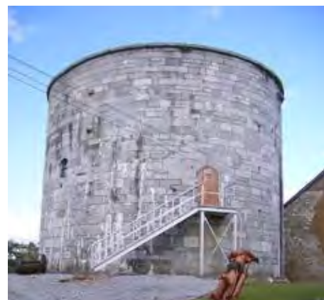
Fig. 3.66 Martello tower, built 1822.
