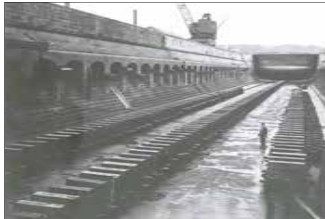
Fig. 2.71 Basin excavation work during the 1870s.
