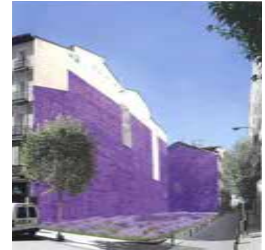
Fig. 5.132 The use of colour and integrated planting to soften a derelict plot.
