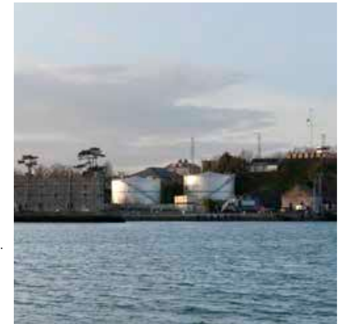
Fig. 3.31 Oil silos on Haulbowline.
