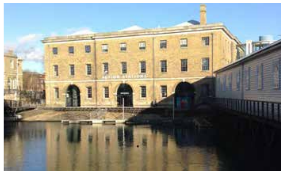
Fig. 3.121 Boathouse 6, a Victorian structure now houses an indoor visitor attraction centre.
