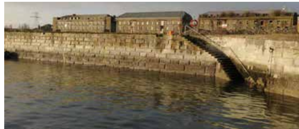
Fig. 2.79 View of the west quay wall.
