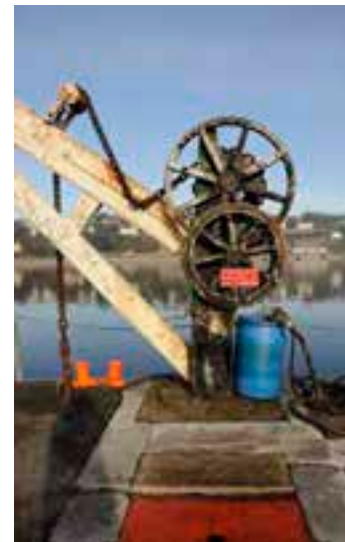
Fig. 5.116 Working crane at north quay wall edge.
