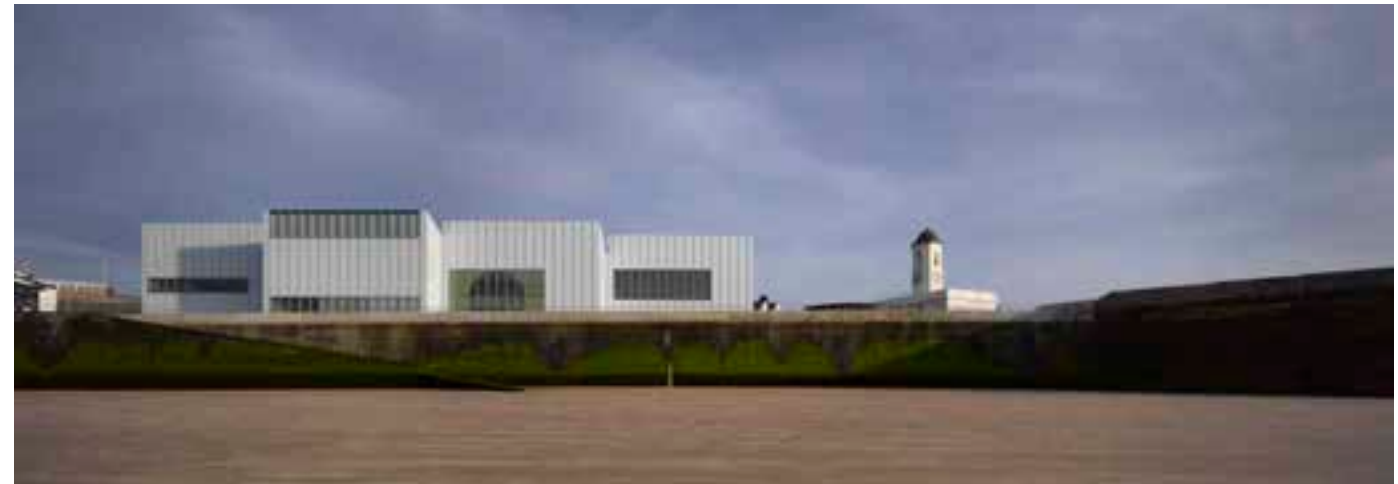
Fig. 5.146 The creation of a landmark building at the end of a promontory.
