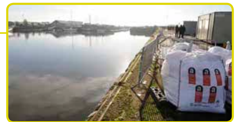
Fig. 2.54 View along the dockyard west wall.
