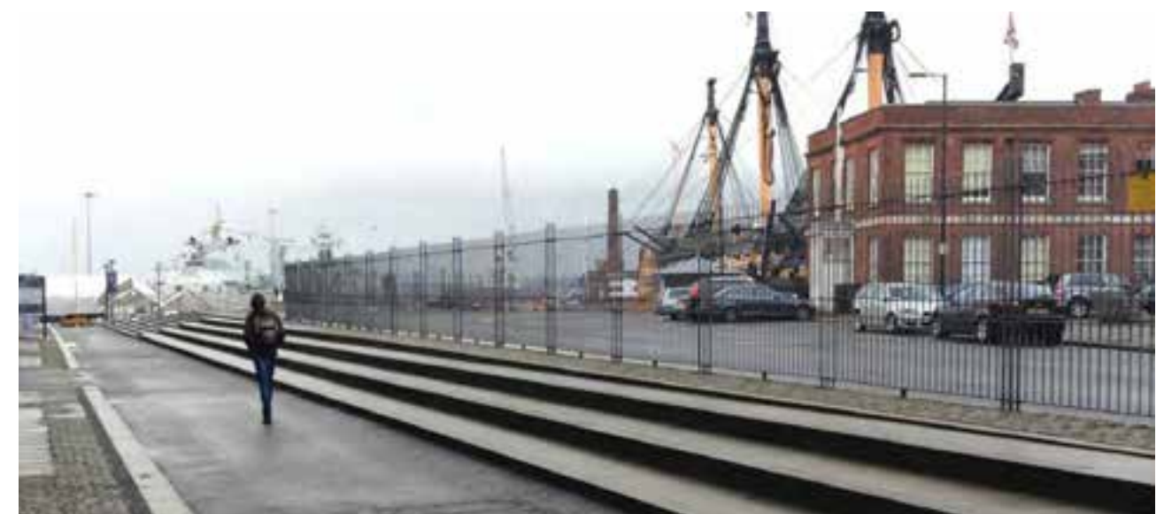
Fig. 3.118 Portsmouth Historic Dockyard. Image shows discrete security boundary.
