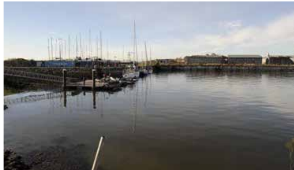
Fig. 2.82 View of the west wall and the south east slipway into the docks.
