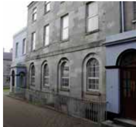
Fig. 3.59 Base HQ, built 1822.
