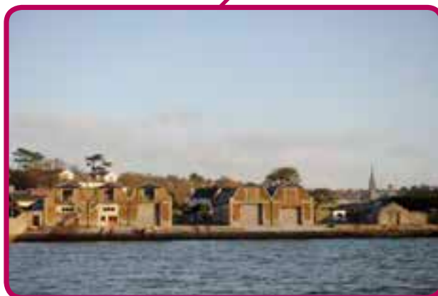
Fig. 2.59 View of the historic boat houses from the south.
