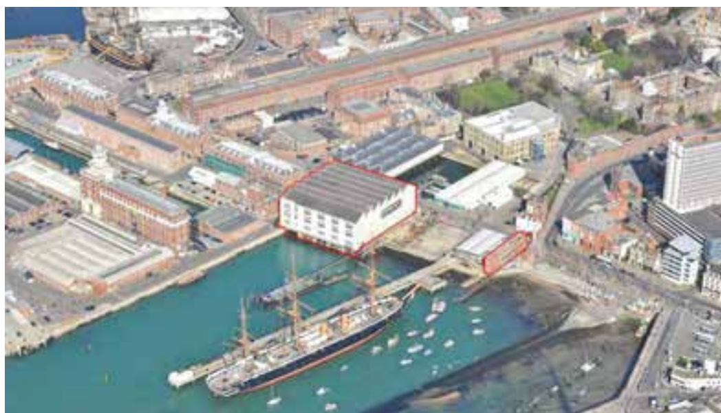
Fig. 3.165 Boat House Number 4, in Portsmouth Historic Dockyard, being renovated for use as a ship building third level college.
