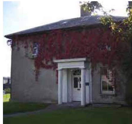
Fig. 3.55 3 bay office building, built 1822.
