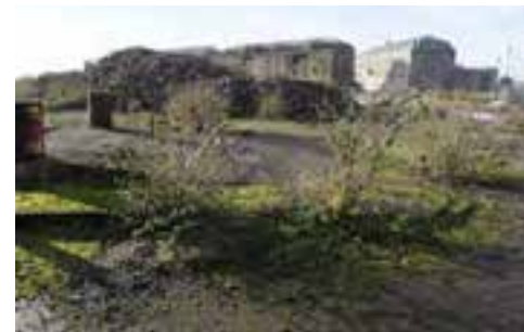
Fig. 2.74 View of the ISPAT site.
