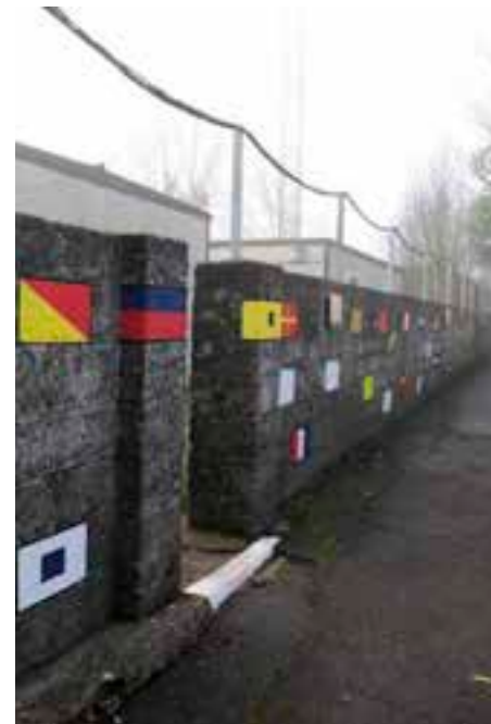
Fig. 3.19 View of more recent boundary walls.
