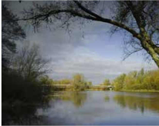
Fig. 5.74 Limerick Living Bridge.
