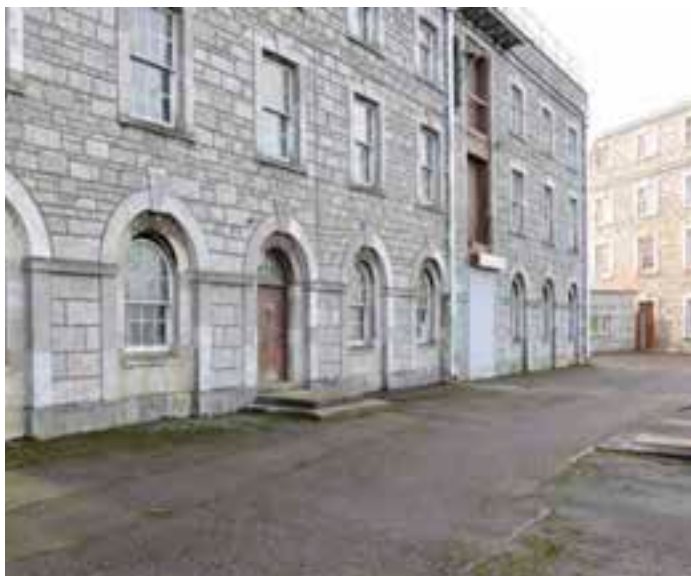
Fig. 5.143 The existing interfaces with the surrounding context is a key consideration for the historic buildings.
