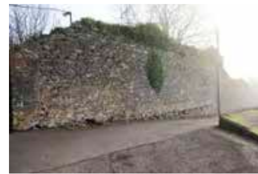
Fig. 5.04 Historic wall on Haulbowline.
