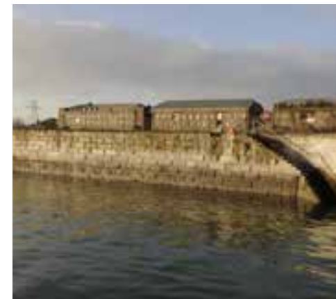
Fig. 2.73 View of the dockyard west wall.
