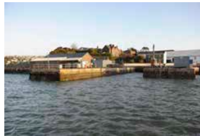
Fig. 3.101 View of the south western naval deep water diving pier.
