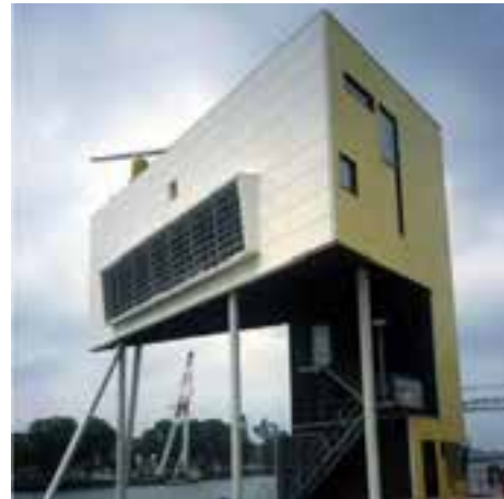
Fig. 5.12 Bridge Watchers House and Quay, Rotterdam.
