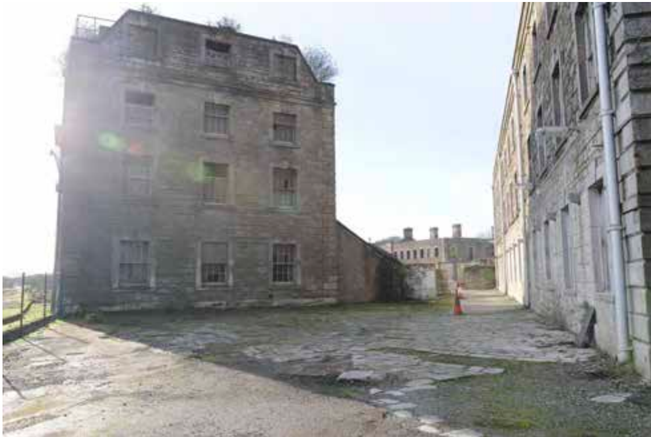
Fig. 5.142 The existing Store Houses provide a substantial floor plate for future adaptive re-use.
