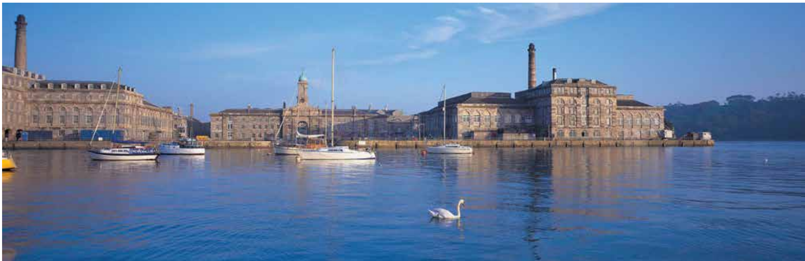
Fig. 3.135 Plymouth Naval Dockyard - View of Marine Basin.
