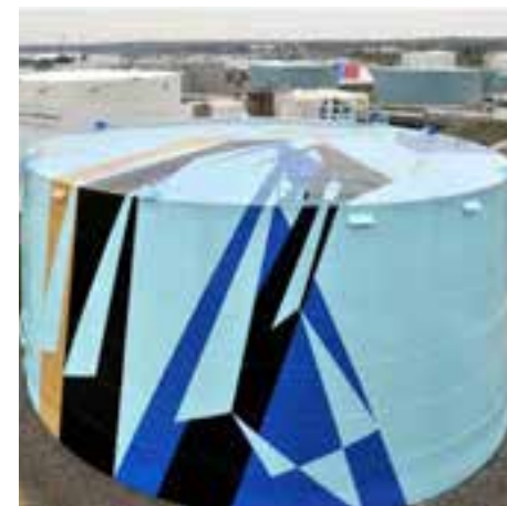
Fig. 5.20 Sprague oil tank, South Portland.
