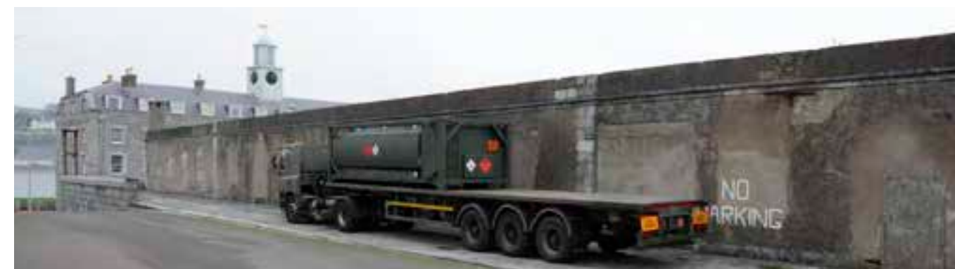
Fig. 3.09 The existing rain water reservoir for the island is housed centrally behind the Store Houses. The view illustrates the screen wall to the reservoir facility.
