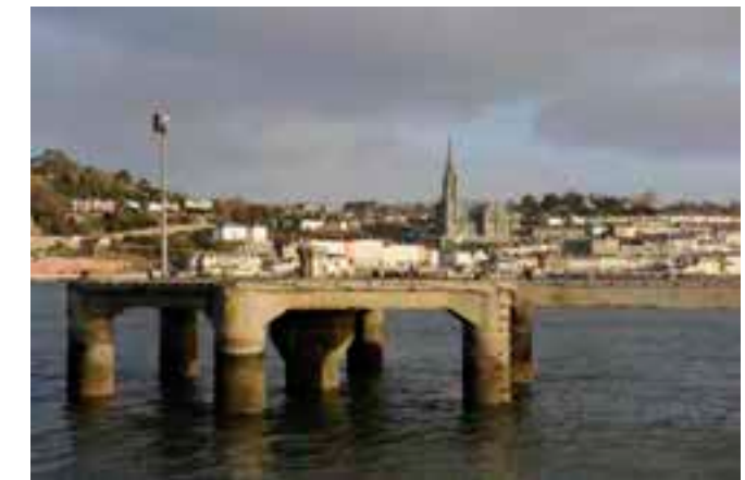
Fig. 3.100 View of the defunct northern pier.
