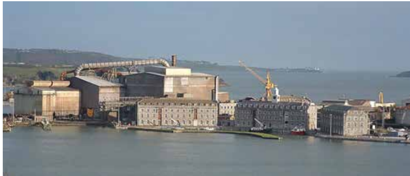
Fig. 3.41 View of Irish steel factory ISPAT. Store Houses dwarfed in foreground.
