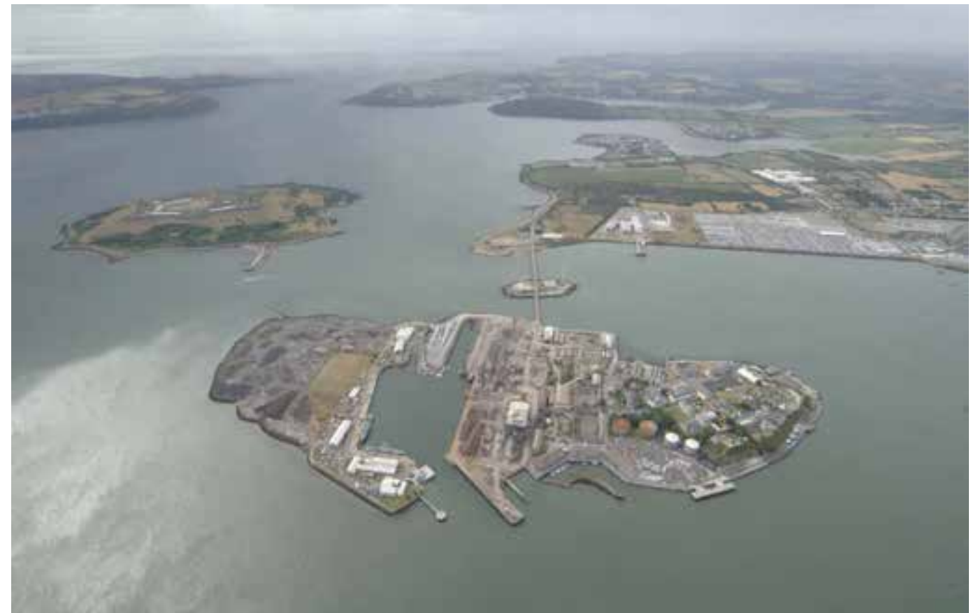
Fig. 3.93 Aerial of Spike and Haulbowline islands from the north. NMCI is also visible in the background. (Image courtesy of the Irish Defence Forces)
