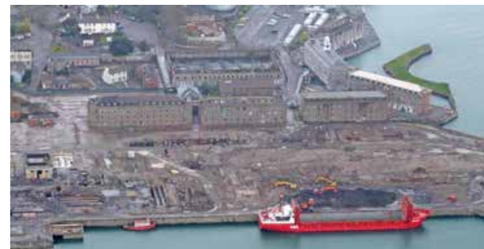
Fig. 3.47 ISPAT site during site clearance.
