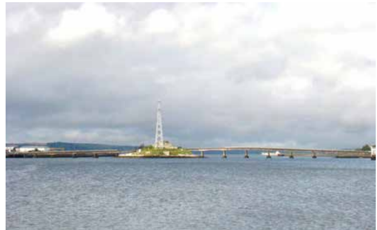
Fig. 8.05 Bridge to Haulbowline Island.
