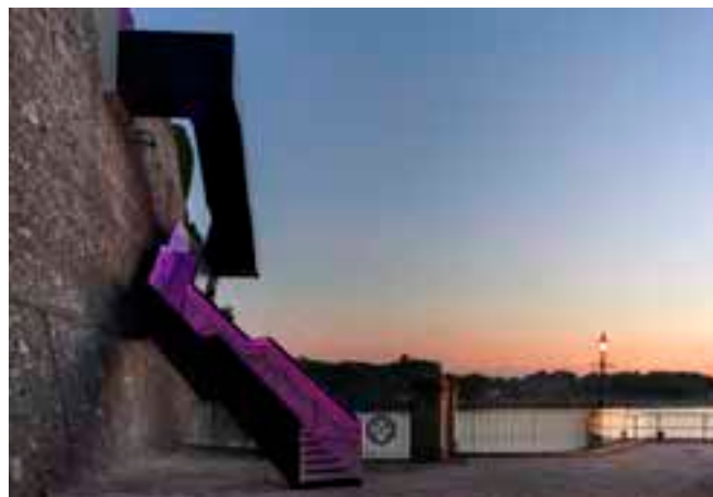
Fig. 5.93 Coast path staircase, Plymouth.
