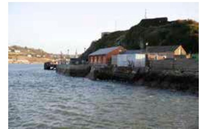
Fig. 3.102 View of the northern naval "daily" access pier.
