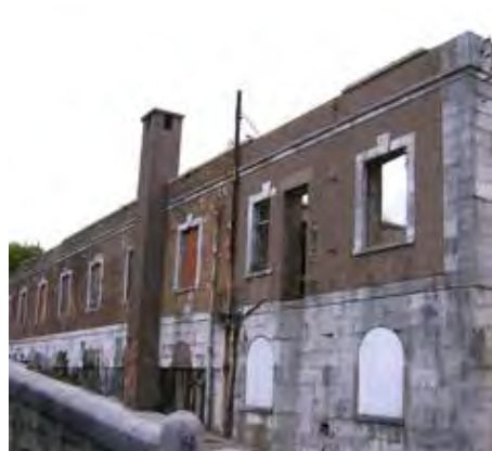
Fig. 3.74 Former tank building, built 1822.
