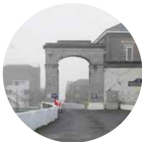
Fig. 2.17 Archway on Haulbowline Island.
