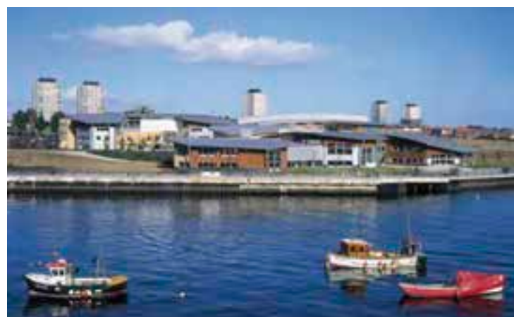
Fig. 5.152 Views of Sunderland University stepping down to the water's edge.
