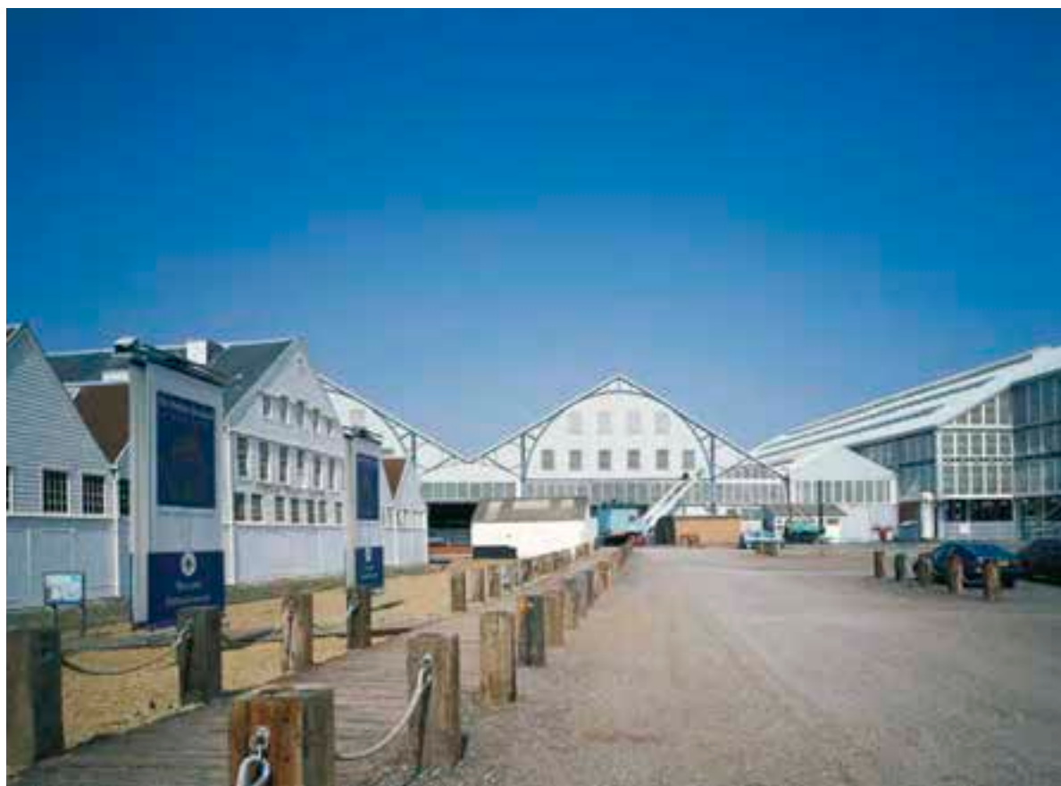
Fig. 3.127 Chatham Historic Dockyard after renovation.
