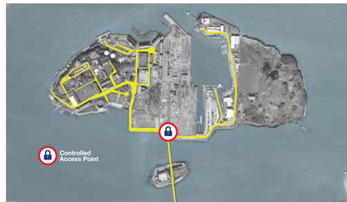
Fig. 3.26 Roads on the island and point of restricted access. Access to the island is restricted, controlled at the central arrival point by naval security.
