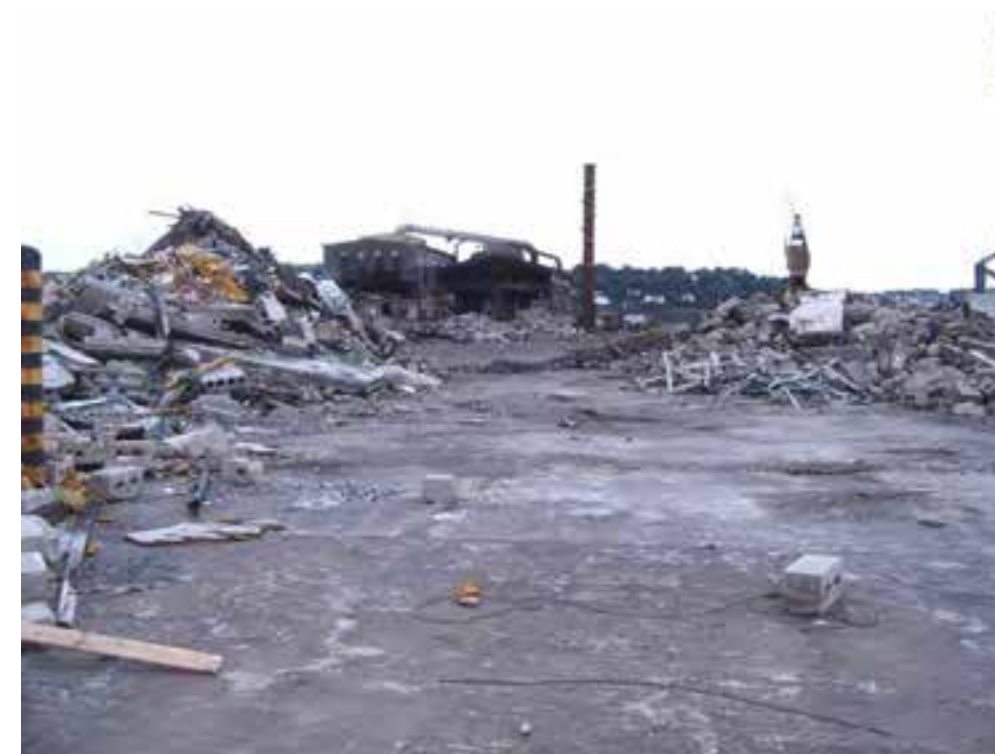
Fig. 3.45 ISPAT photographed looking north, after demolition.
