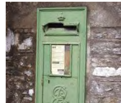
Fig. 3.80 Cast-iron letter box, erected c. 1905.
