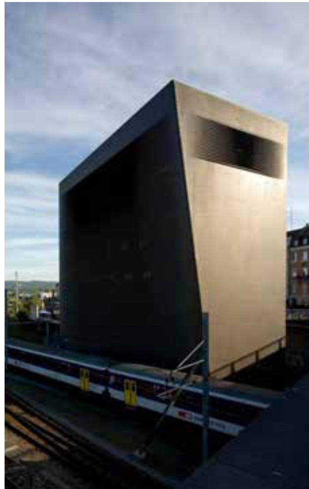
Fig. 5.147 Industrial but crafted signal box, Basel.
