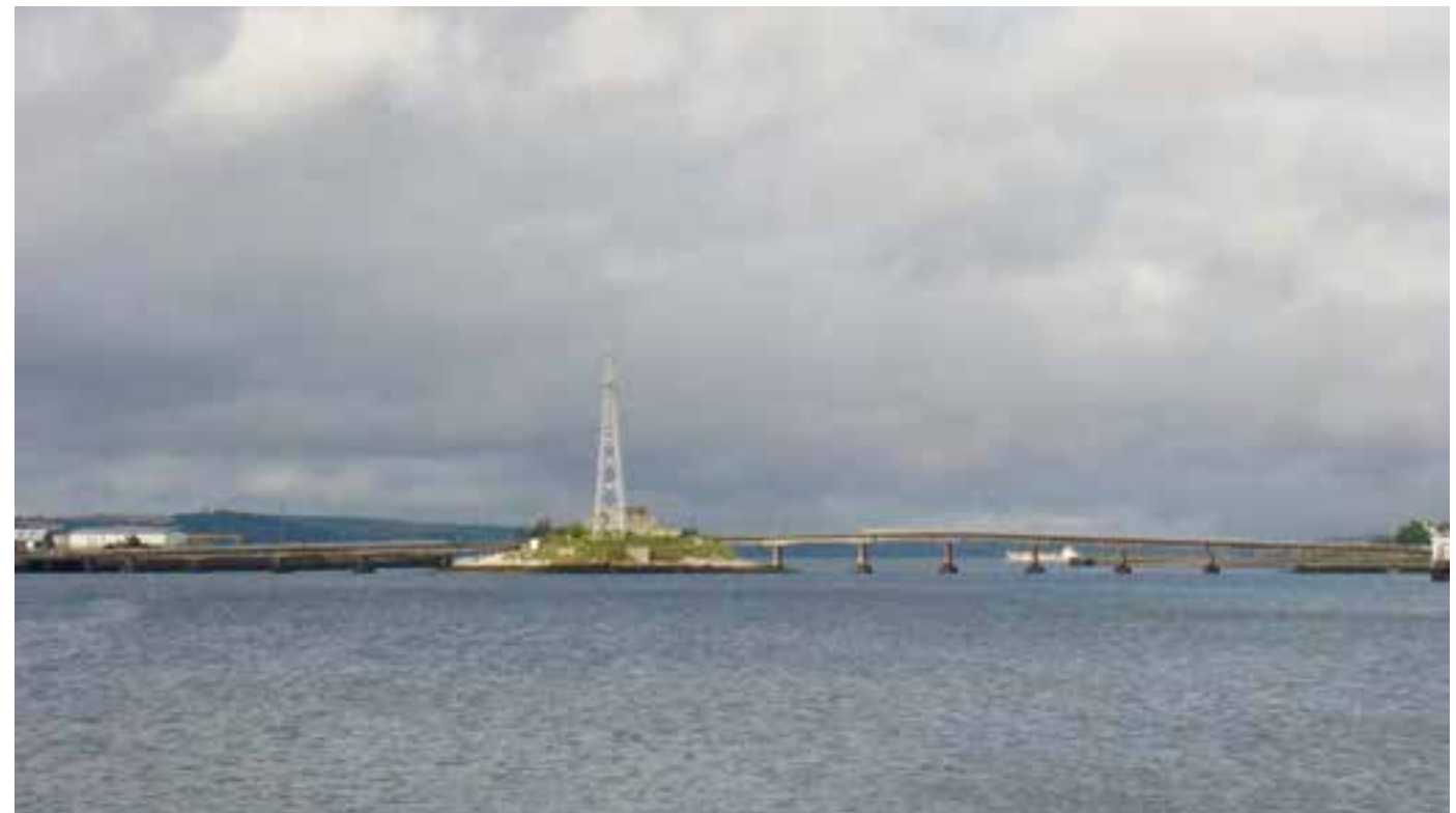
Fig. 3.107 The existing bridge has been recently refurbished to cater for larger vehicles; particularly important during the remediation works of the East Tip. This will also allow for greater logistical movements by road for the Naval Service.
