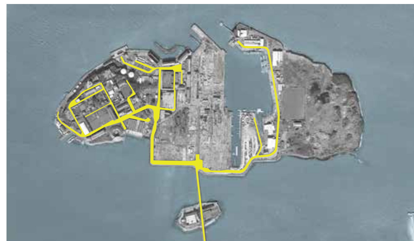
Fig. 3.98 Roads on Haulbowline Island. The island has a number of informal roads that allow access throughout.
