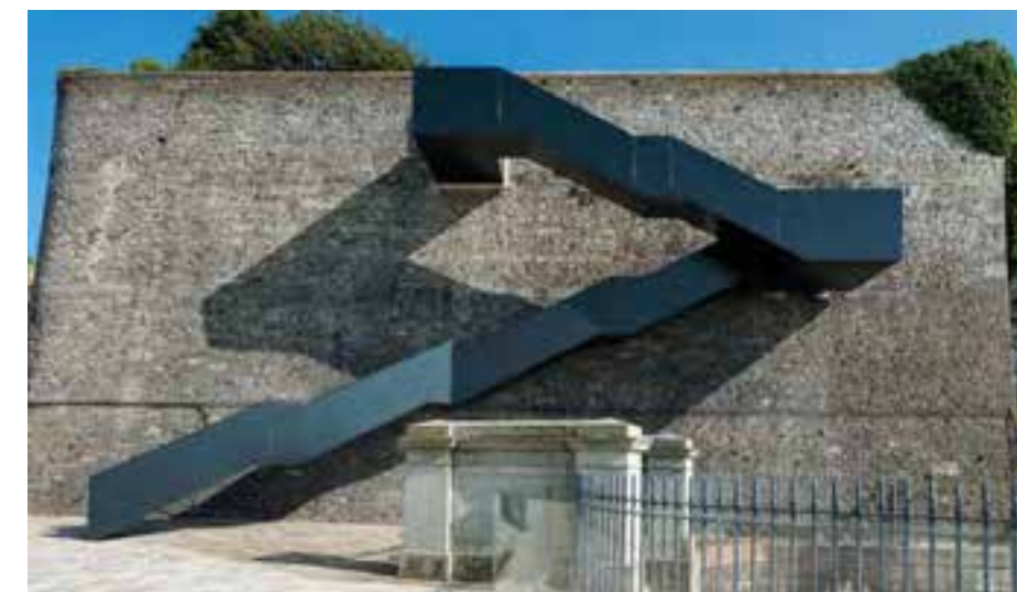
Fig. 3.138 Coast Path Staircase, Plymouth.
