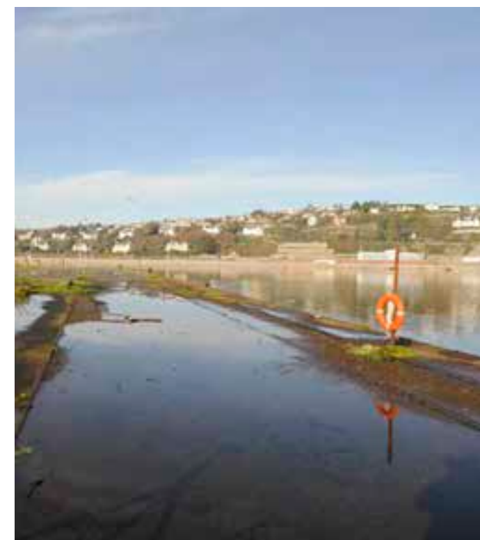
Fig. 3.11 Flooding on the island.
