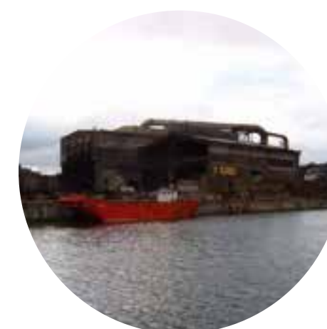
Fig. 2.26 ISPAT factory during its dismantling.
