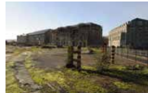
Fig. 2.75 View of the ISPAT site.
