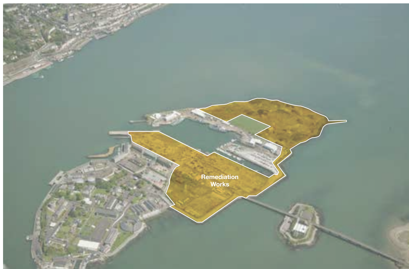
Fig. 5.158 Phase 00 - Remediation Works.
