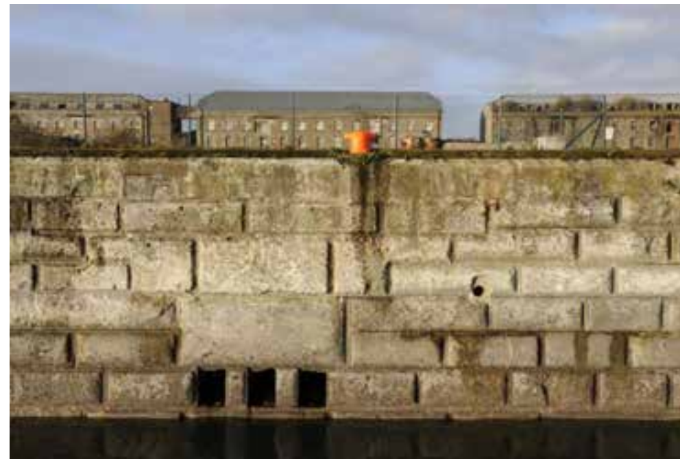
Fig. 2.80 Detailed view of the west wall still in good working order.
