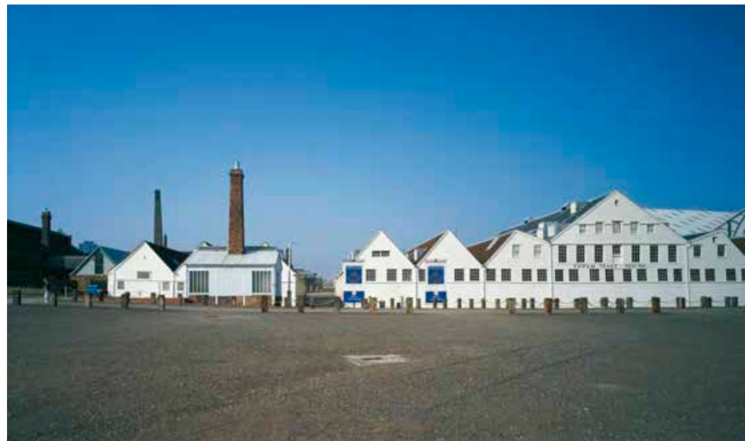
Fig. 3.128 Chatham Historic Dockyard - Mast Houses & Mould Loft after renovation.
