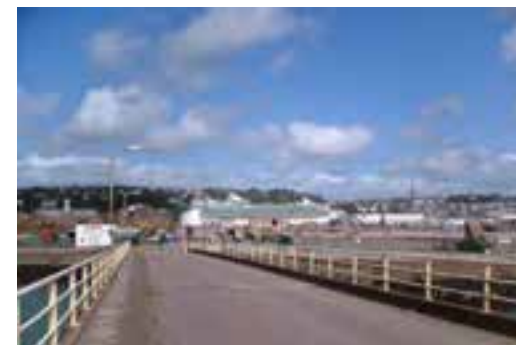
Fig. 5.08 View of island approach via road.
