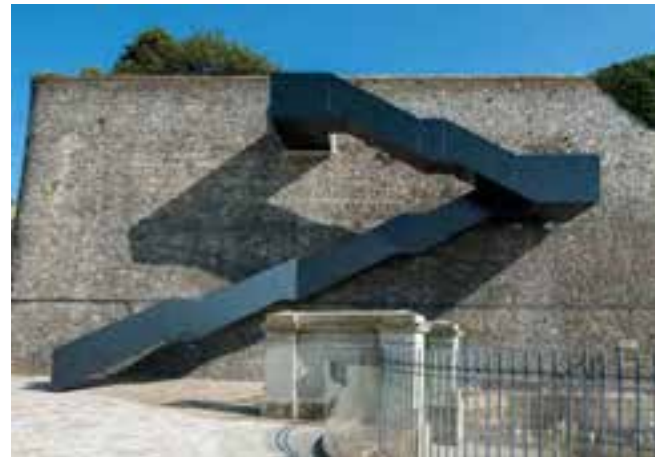
Fig. 5.92 Coast path staircase, Plymouth.
