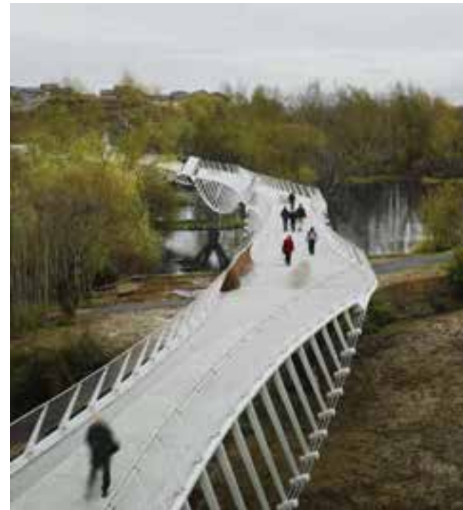
Fig. 6.14 Millennium Bridge, University of Limerick.
