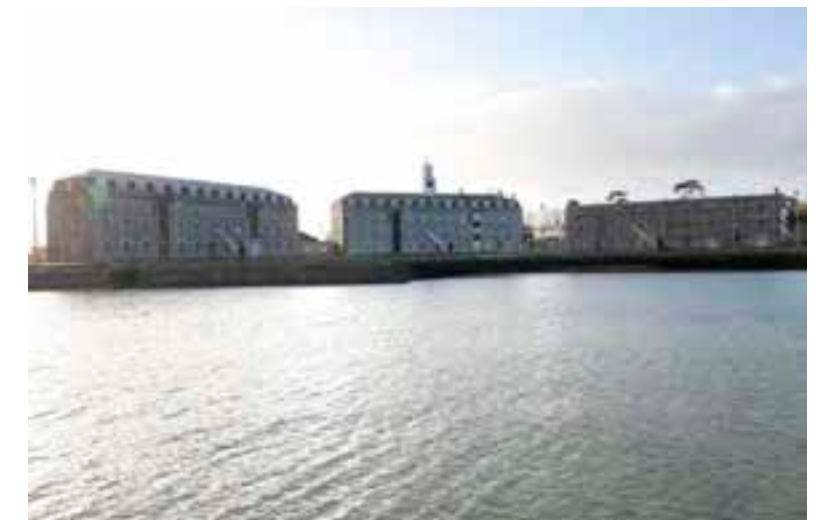
Fig. 1.09 Haulbowline Store Houses viewed from the northern sea approach.
