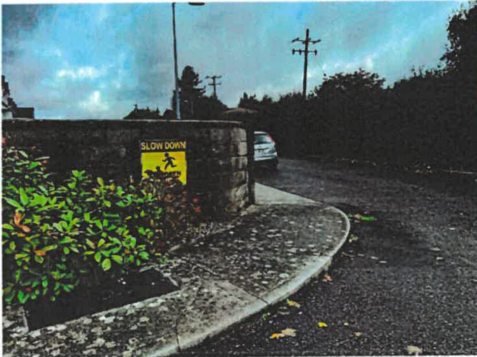
3m setback, 1.2m high view to the North "Junction B"
