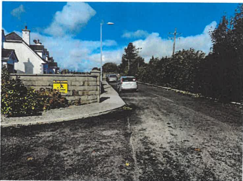
Common parking situation in front of houses 11,12 & 13
