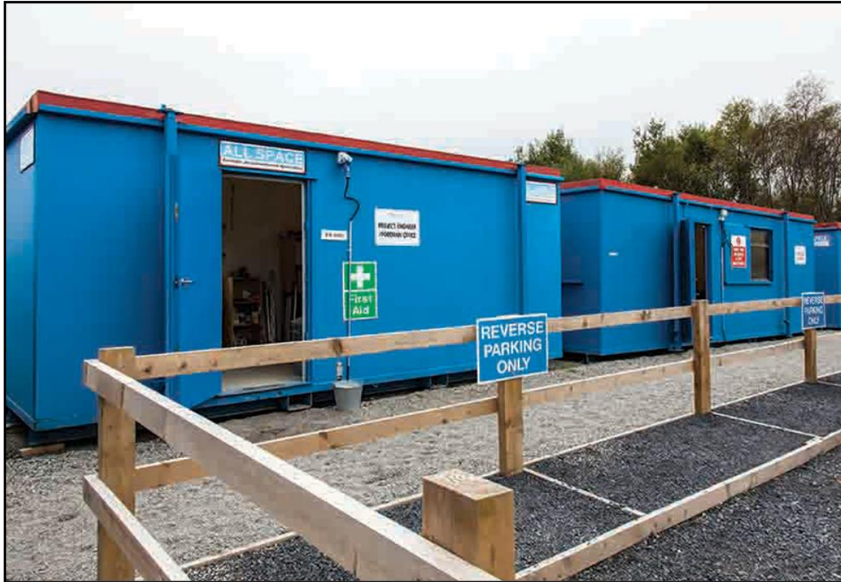
Figure 4-1: Typical temporary site construction compound
