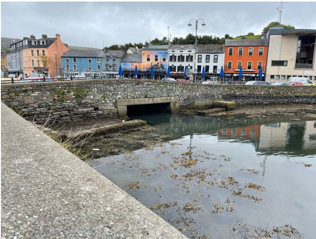
Plate 6: View of culvert visible from harbour, taken from south.
