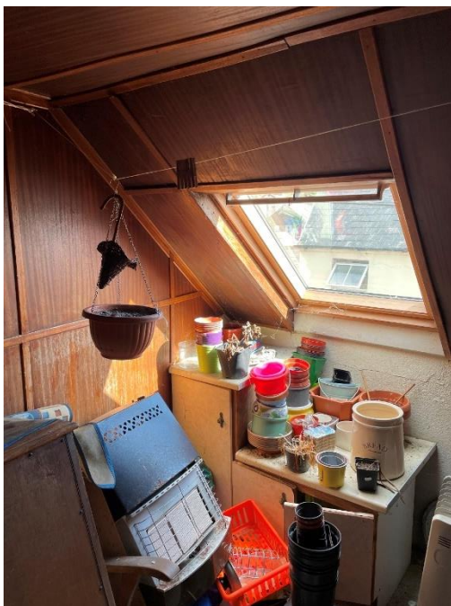
68 Interior of Building C. Attic room. Walls have been dry-lined. Not original to build. (credit: Cork County Council)
