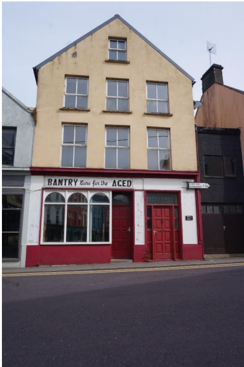
34 Exterior of Building B.
