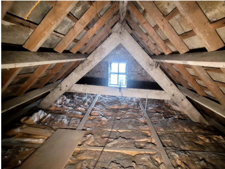
55 Interior of Building B. Original roof structure has been retained. Evidence of parging. (credit: Cork County Council)
