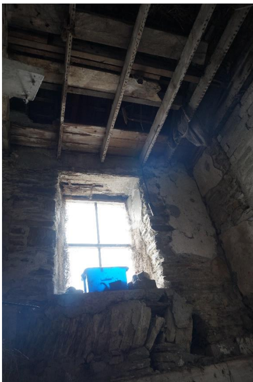
81 Interior of Building D. Original stone structure is exposed. Timber roof joists.
