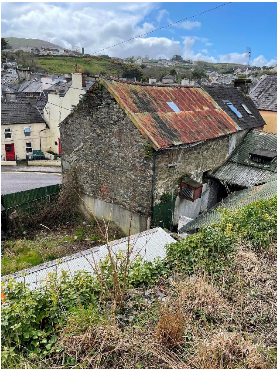
86 Rear of Building D. (credit: Cork County Council)
