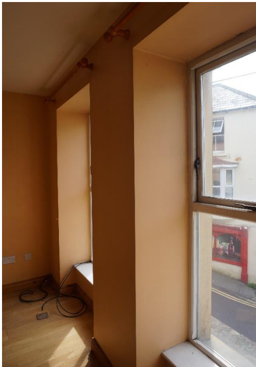
43 Interior of Building B. Walls have been dry-lined. Not original to build.
