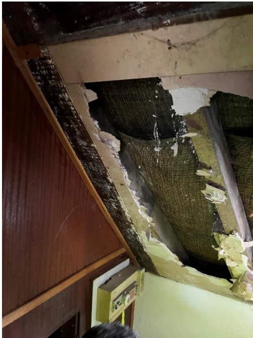
55 Interior of Building B. Original roof structure has been retained. Evidence of parging. (credit: Cork County Council)
