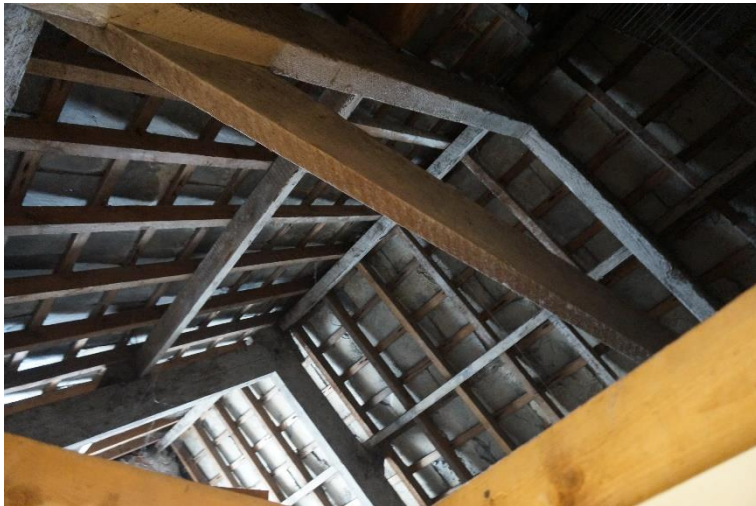
53 Interior of Building B. Original roof structure has been retained. Evidence of parging. (credit: Cork County Council)
