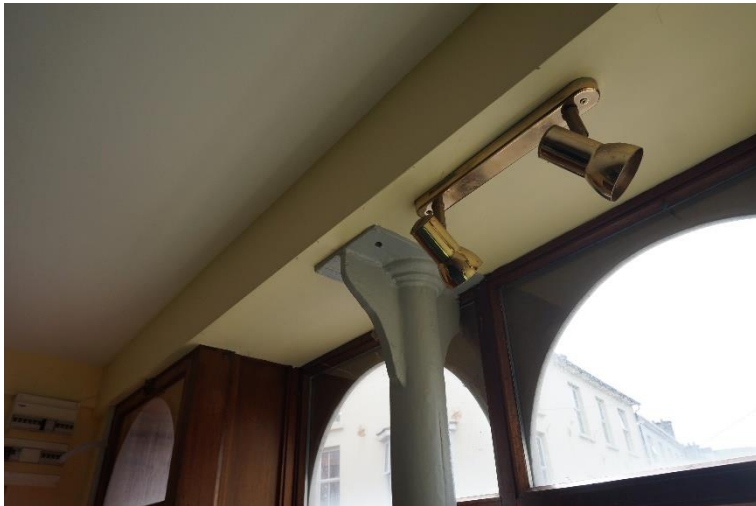
37 Interior of Building B. Reveal of alterations and cast-iron column. (credit: Cork County Council)
