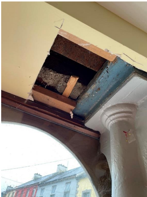
37 Interior of Building B. Reveal of alterations and cast-iron column. (credit: Cork County Council)
