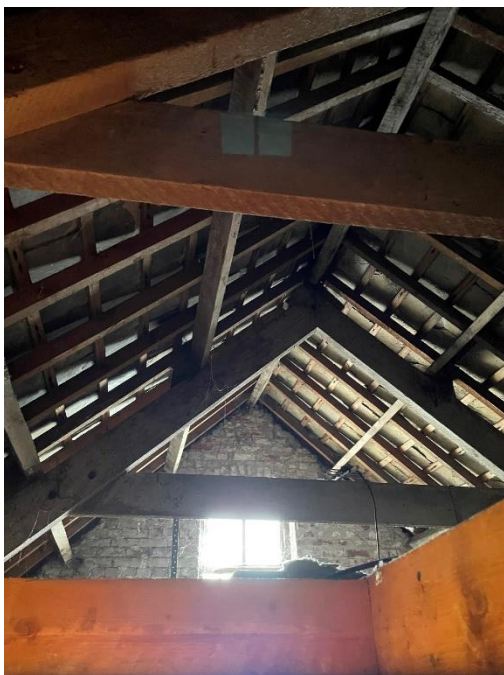
53 Interior of Building B. Original roof structure has been retained. Evidence of parging. (credit: Cork County Council)
