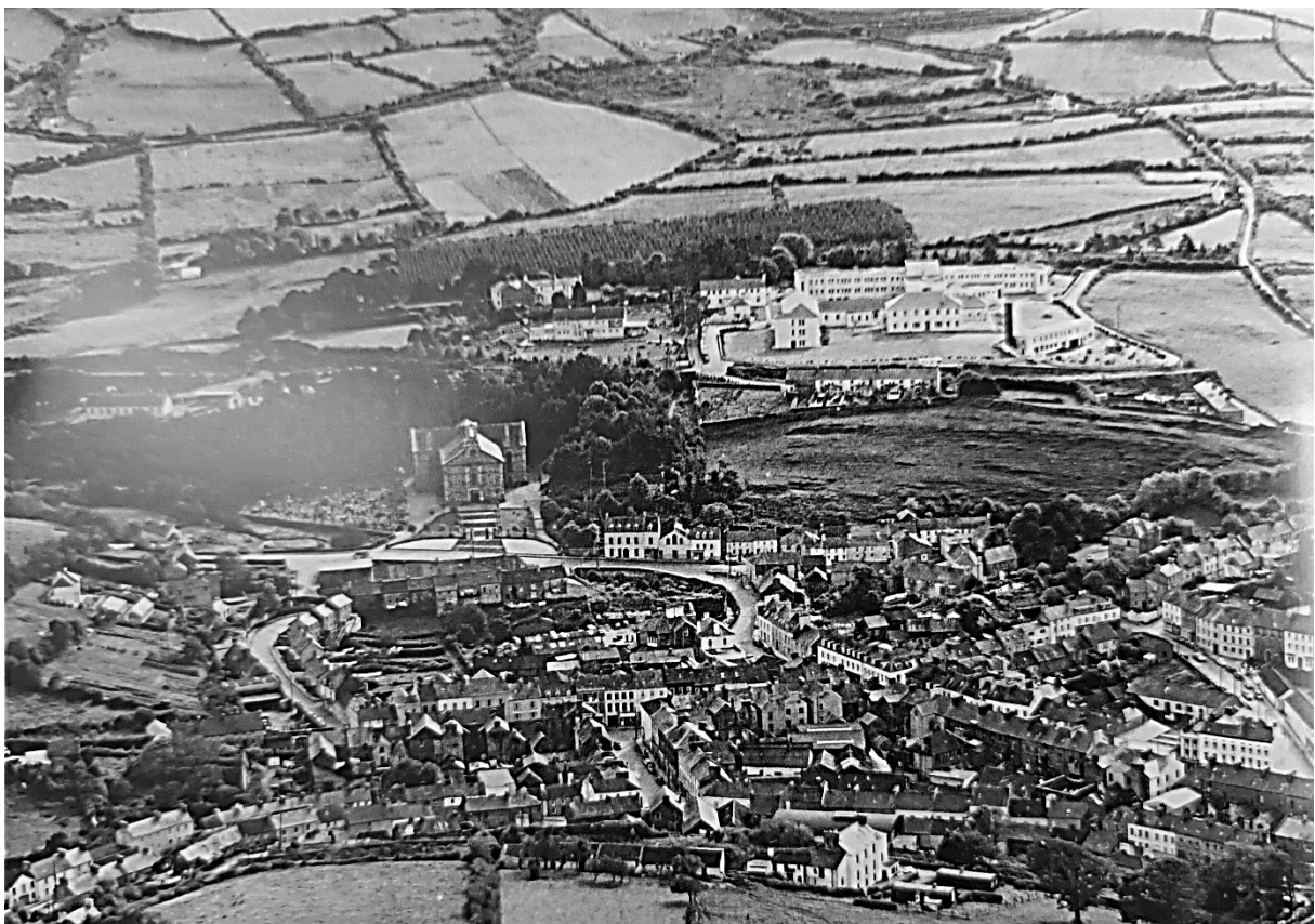
Figure 17 - Aerial View of Bantry Town taken c.1970.
