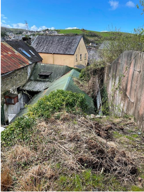
85 Rear of Building D. (credit: Cork County Council)
