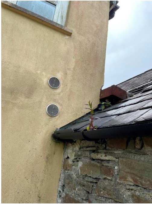
58 Rear elevation of Building B. Ventilation detail. (credit: Cork County Council)
