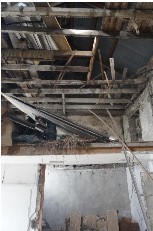
74 Interior of Building D. Evidence of timber roof joists, some may have been replaced. Exposed original stone structure.
