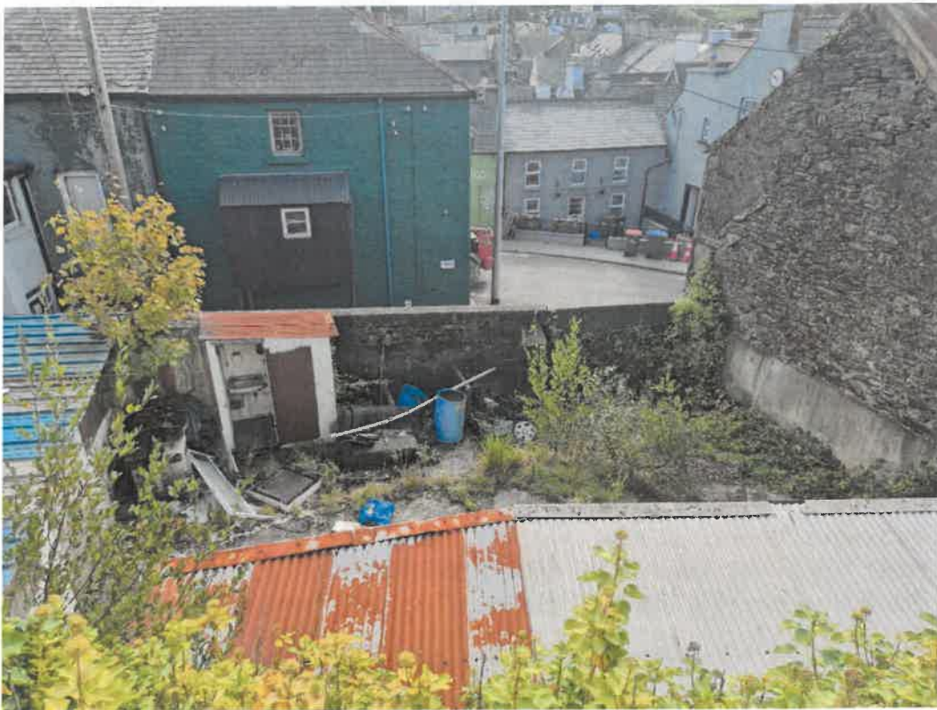
Photograph 2.2 Yard within the Proposed Social Housing Development
