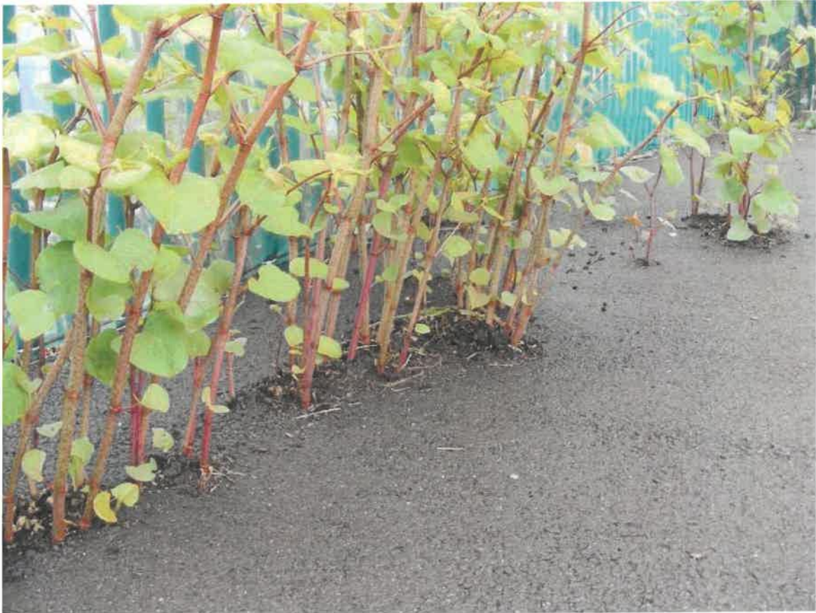
Photograph 1.1 Japanese Knotweed breaking through a bituminous surface in Cork City (Source: John O’ Donovan, O’ Donovan Agri-Environmental Services)
