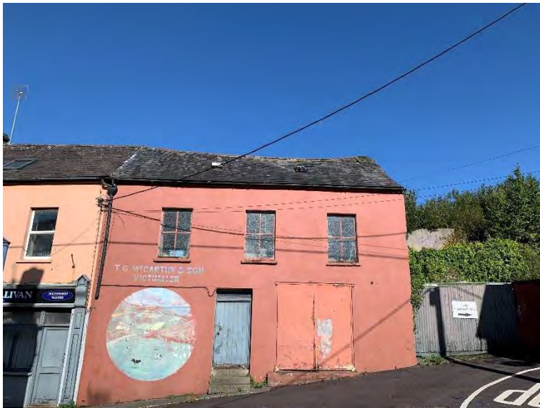
Plate 3-1: Building 1 and partial view of Building 2
