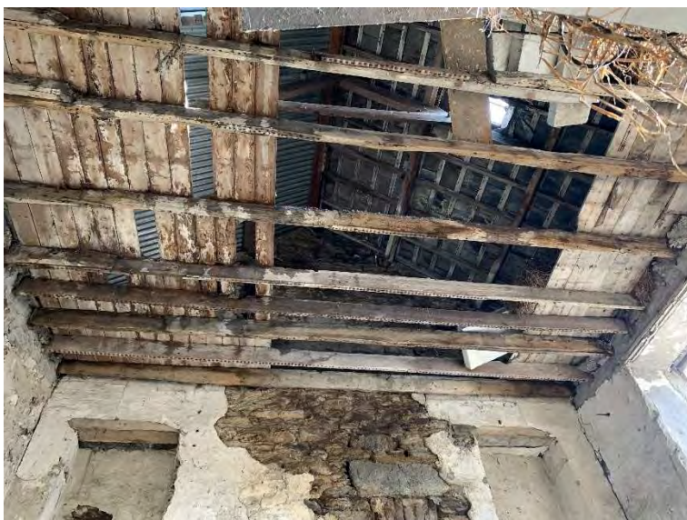
Plate 3-2: Remaining ceiling and roof of building 1
