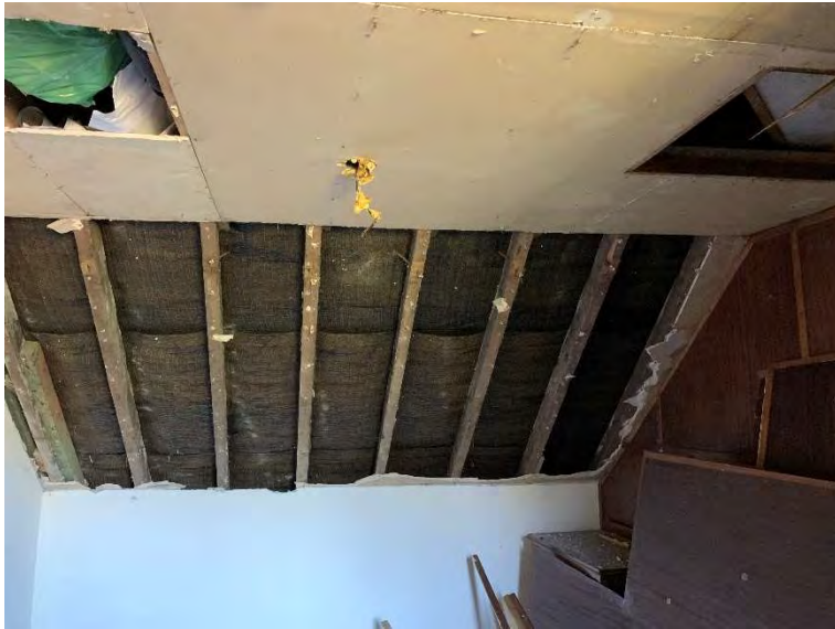
Plate 3-5: Roof space within building 2- small and cluttered
