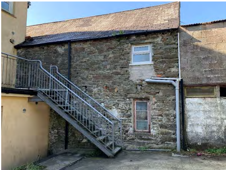
Plate 3-8: Stonewall and slate roof on eastern elevation of building 4
