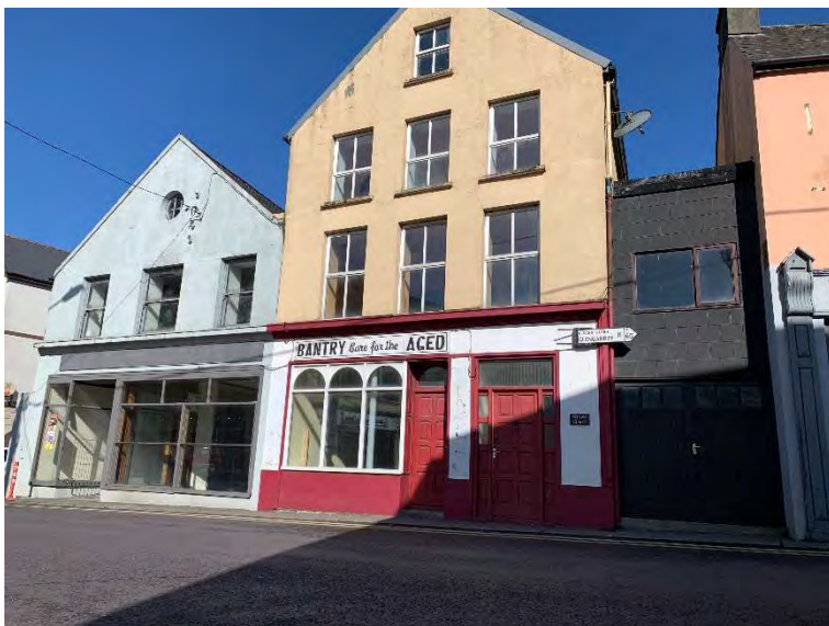
Plate 3-6: Building 3 and building 4, with a partial view of building 2
