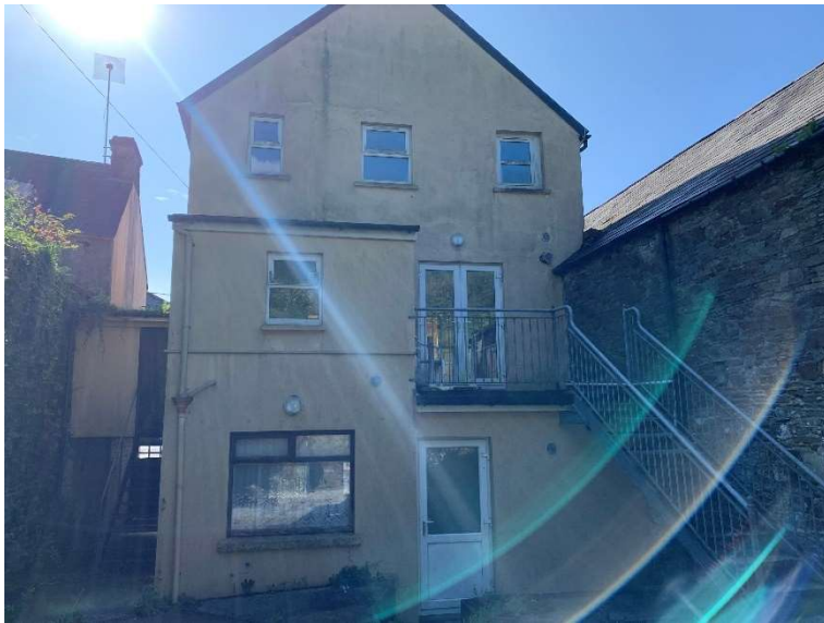
Plate 3-7: Rear (northern elevation) of building 3
