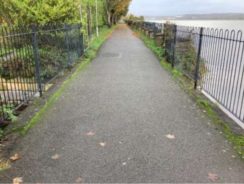
Plate 8: Deck of railway bridge RPS 01475, looking NW.
