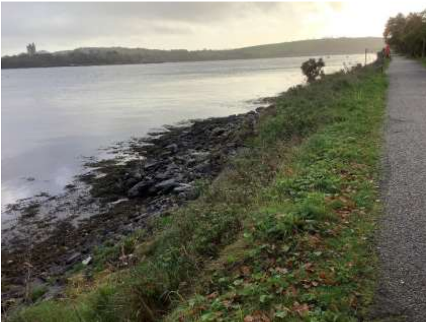
Plate 13: Railway embankment at shoreline to NW of Abbott's Bridge, looking E.
