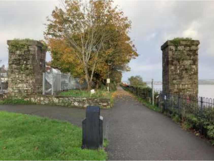
Plate 7: Abutments of foot bridge indicated on 25-inch OS map, looking NW.
