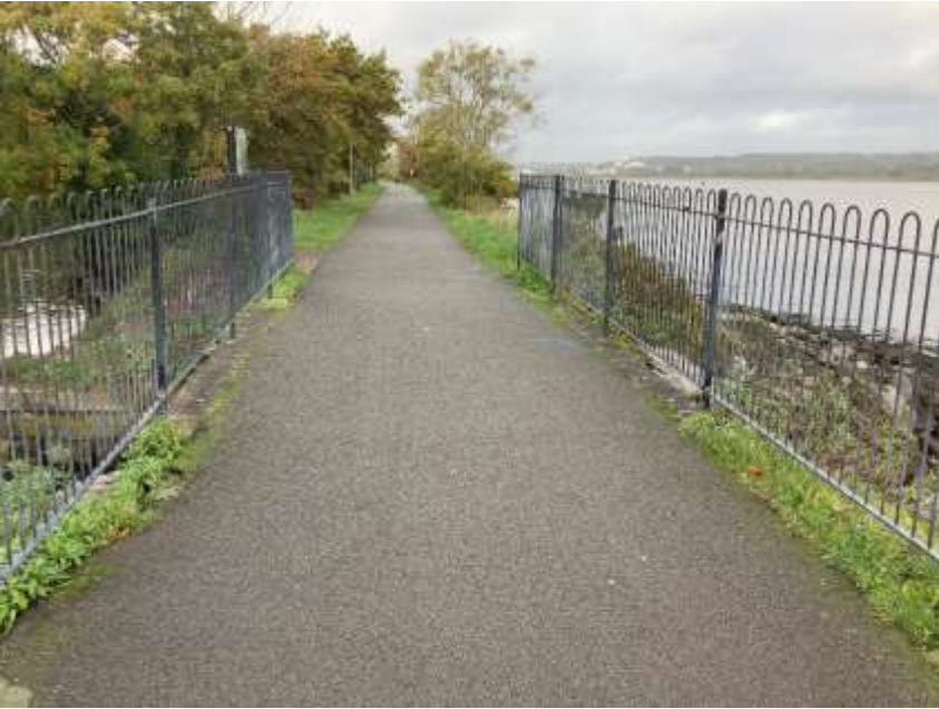
Plate 11: Deck of Abbott's Bridge RPS 01476, looking NW.
