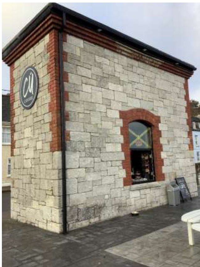
Plate 3: RPS structure 01469 Water Tower to west of proposed route, looking NW.
