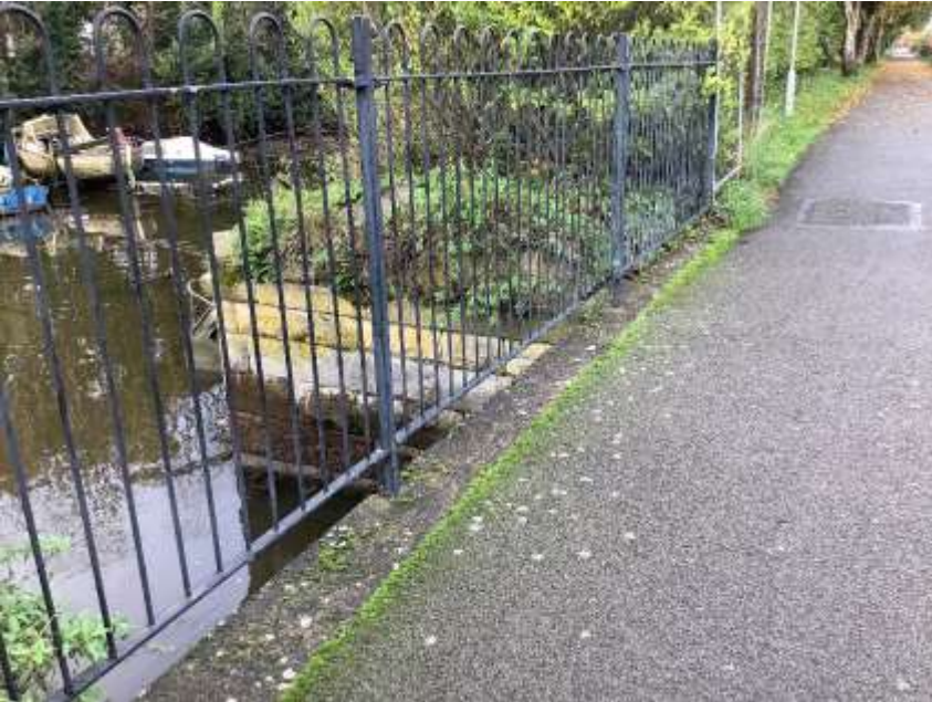
Plate 9: Abutment of bridge RPS 01475, looking W.
