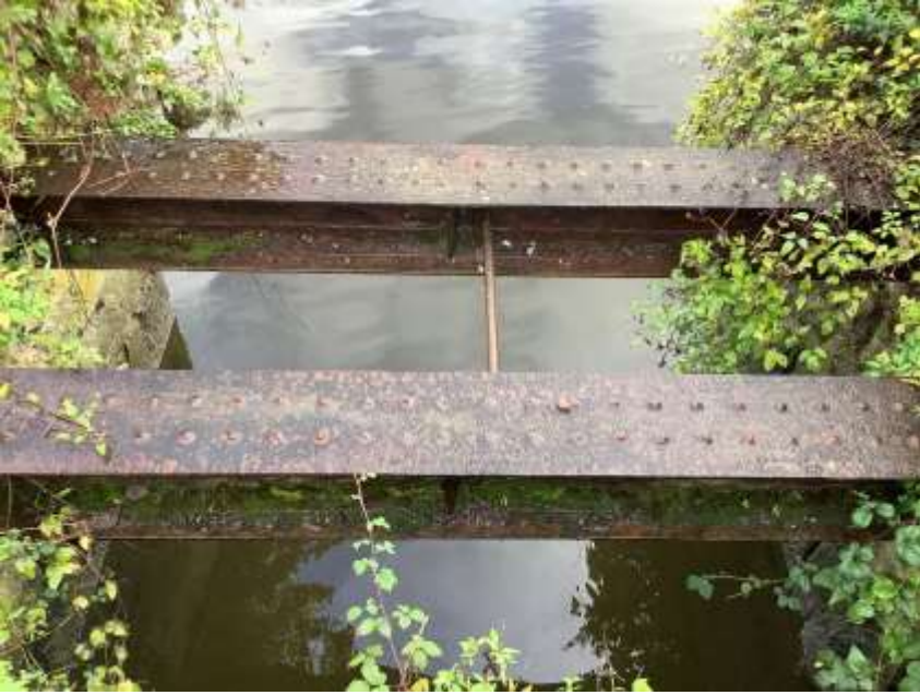
Plate 6: Girders immediately E of bridge in Plate 5, looking E.
