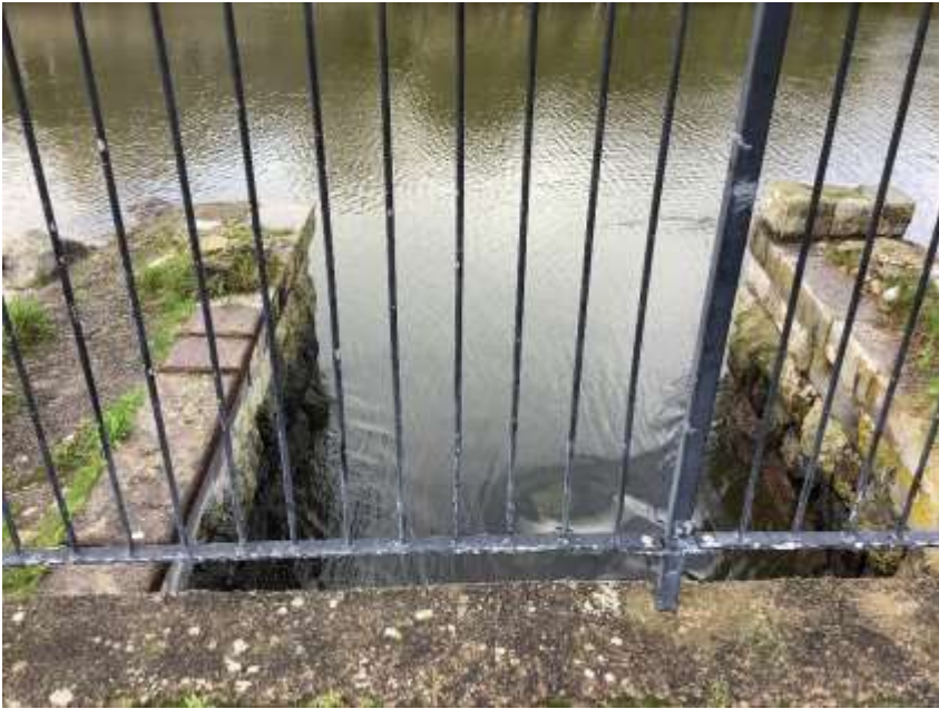
Plate 12: Abutments at SW side of Abbott's Bridge.
