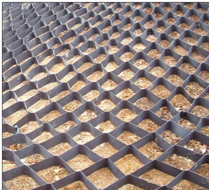
Plate 1-1 - Typical cellular soil confinement system.
