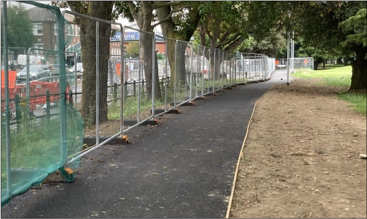
Plate 1-5 - Finish path and reinstate area alongside.
