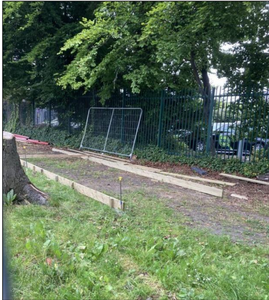
Plate 1-2 - Prepare the proposed pedestrian and cycle path for the cellular confinement system.
