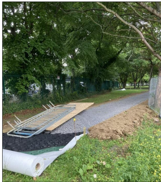
Plate1-4 - Reuse excavated soil to build slope off path.
