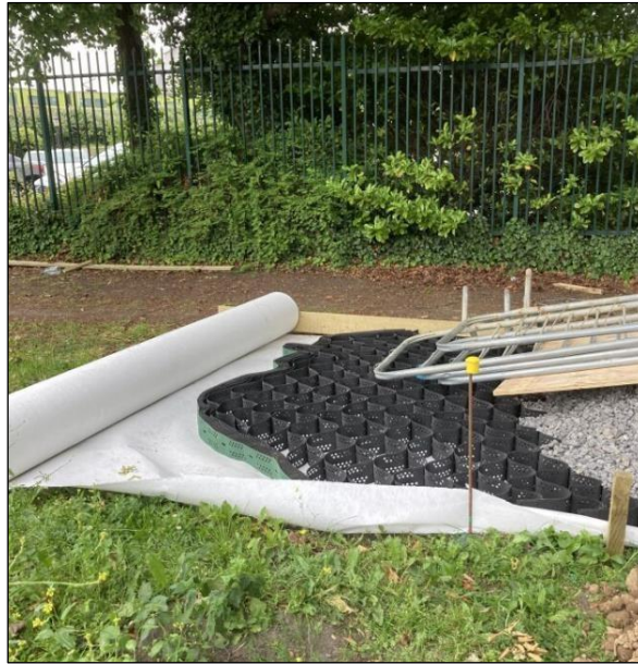
Plate 1-3 - Fill cellular material confinement system to evenly distribute loads across the proposed pedestrian and cycle path.
