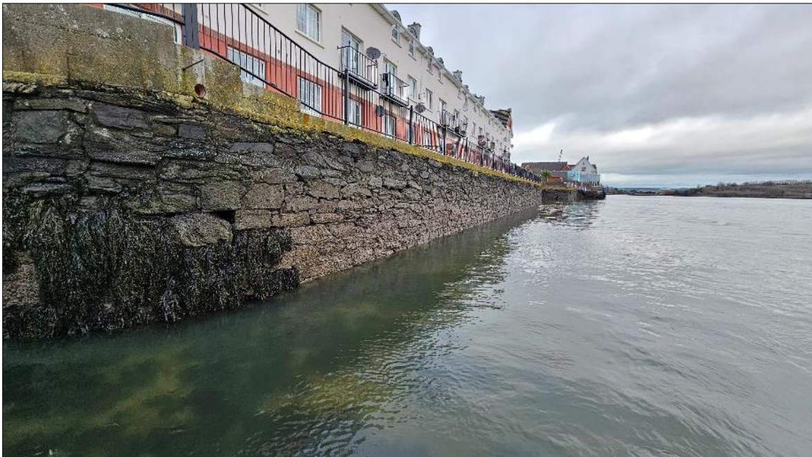
Plate 3.4 The old quay wall at Granary Wharf, Passage West
