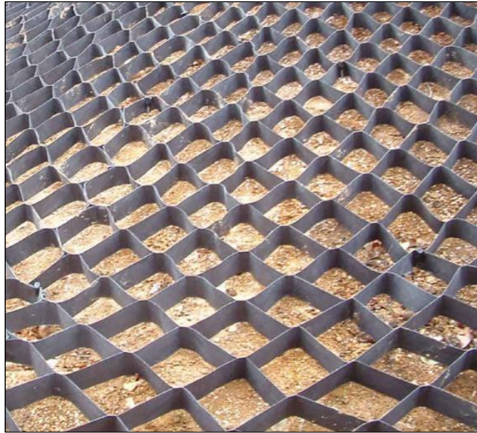
Plate 1-1 - Typical cellular soil confinement system.
