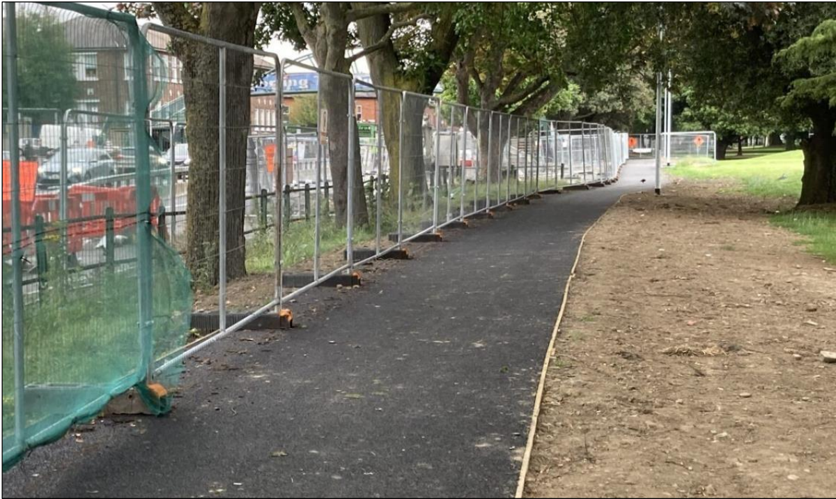
Plate 1-5 - Finish path and reinstate area alongside.
