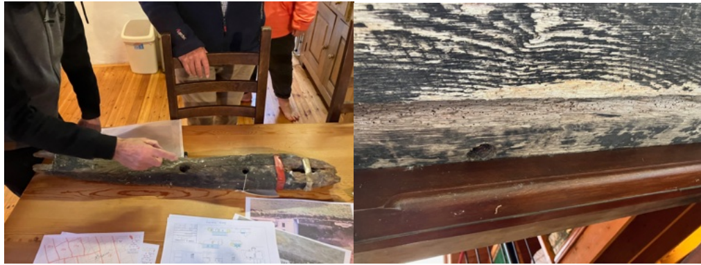
The owners report that when they were working on this cottage they found a stone drain under the floor, which sloped away from the fireplace, and that they relaid the flagstones.
