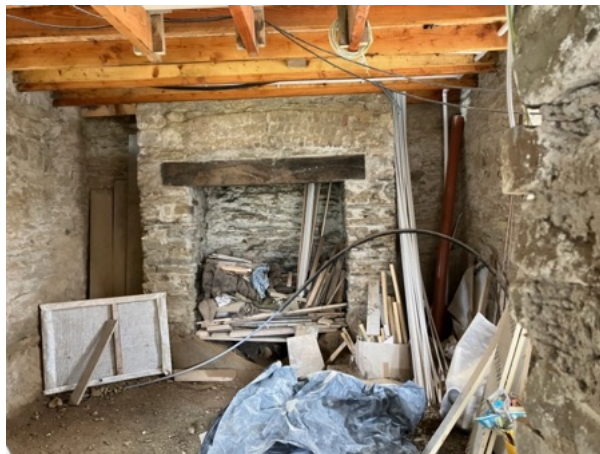
In the kitchen annex the fireplace has had the timber lintel replaced. There was a range installed.
