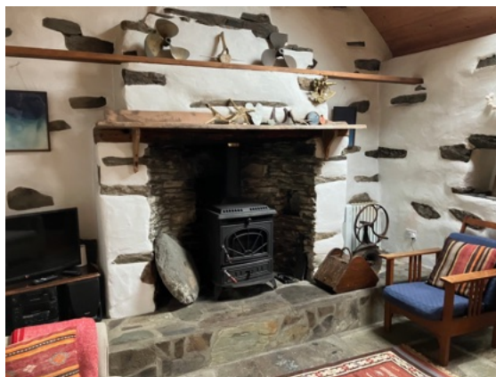
The hearth has an unusual curved background, and the chimney stack is partially external to the gable.
