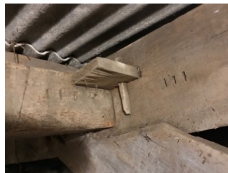
Top right: corbel top row Centre left: large purlins Centre right: pegged A-frame beams in stable. Bottom left: stable building showing good quality masonry partially rendered with lime.
