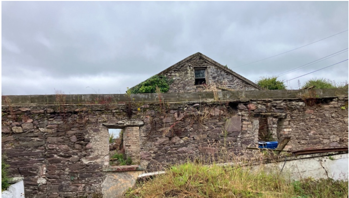
The house previously had a large central chimney stack which was removed since the most recent occupation. Window reveals are made of brick, which may be local as there was a brickworks at Youghal nearby but some bricks appear to be handmade.
