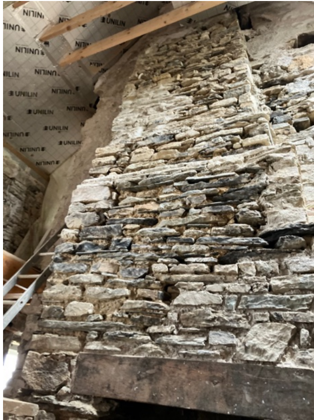
In the kitchen annex the fireplace has had the timber lintel replaced. There was a range installed.
