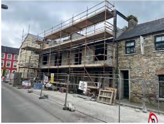
Construction of 6 units in Bandon
