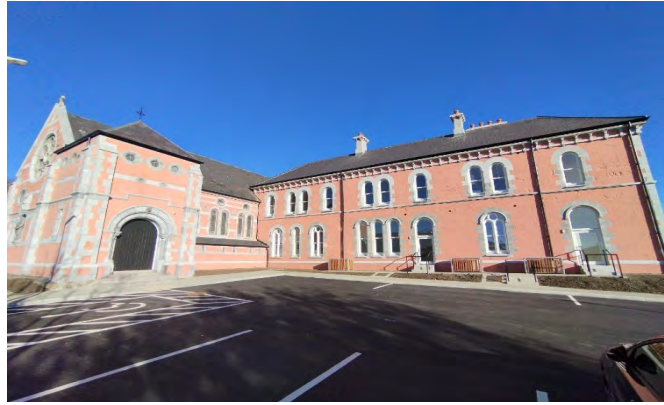
Construction of 18 units at Bantry Convent
