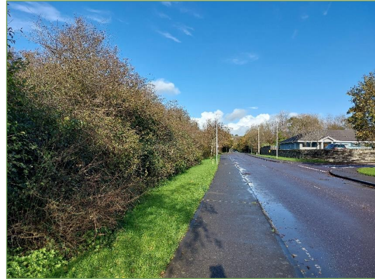
A6. View looking north along the L3235 at the southern extent of the proposed scheme.
