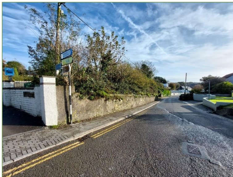
Plate 3.2.1 – Buildings and artificial surfaces dominating the habitats contained within the development boundary, primarily in the form of public roadways.
