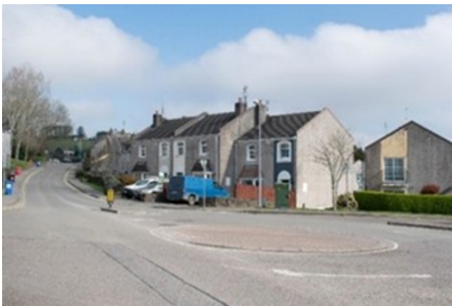
Image 1-5: Wide junction splays, absence of dropped kerbs and tactile paving make many junctions inaccessible, unsafe and difficult to cross for pedestrians, particularly for those with a disability, older adults, or people with buggies, and facilitate increased speeds by motorists.
