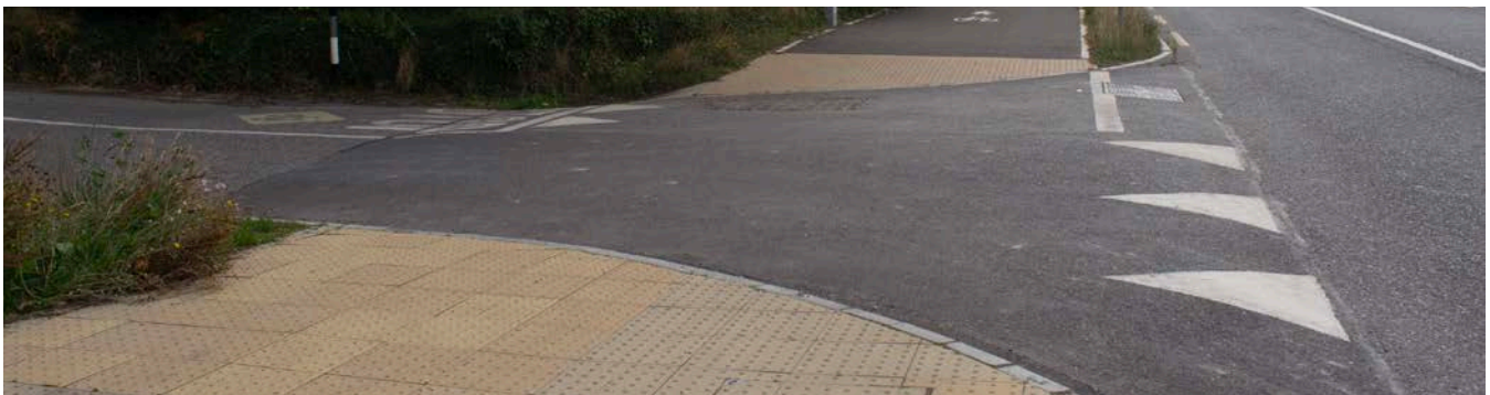
Image 6-1: Example of a Priority Side Entrance Treatment at Glounthaune as part of Cork County Council's Dunkettle to Carrigtwohil Pedestrian and Cycle Route. Source: DBFL.
