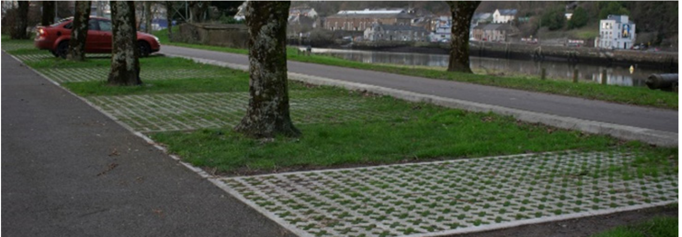
Image 6-2: Example of Grasscrete used on Car Parking Bays at The Marina, Cork. Source: DBFL
