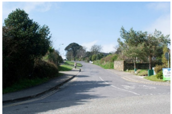
Image 1-5: Wide junction splays, absence of dropped kerbs and tactile paving make many junctions inaccessible, unsafe and difficult to cross for pedestrians, particularly for those with a disability, older adults, or people with buggies, and facilitate increased speeds by motorists.
