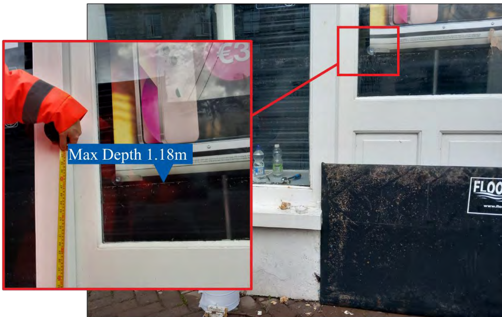
Figure 73: Wrack Mark at Three Shop
