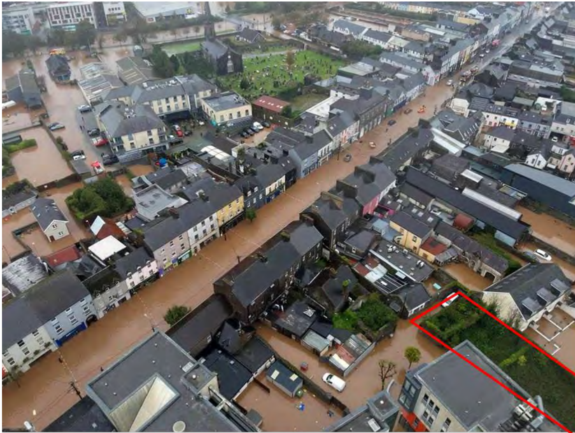
Figure 1.3: Aerial view of the flood on the Main Street and its surroundings.
