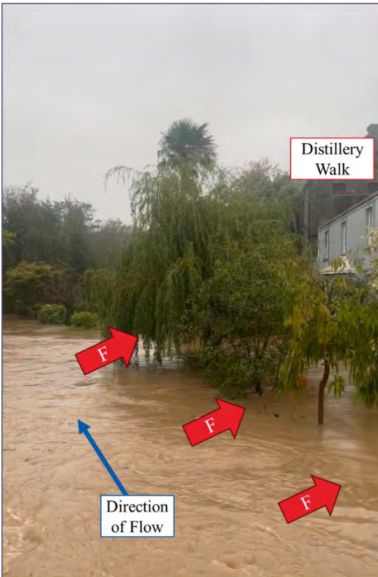
Figure 80: Flooding of Right Bank Downstream of Lewis Bridge
