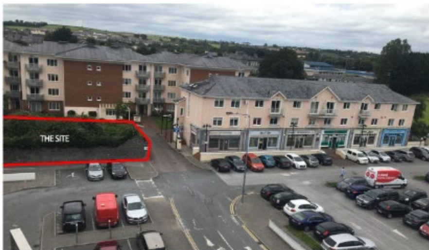
Figure 3. View from neighbouring building looking north across the public car park towards site.
