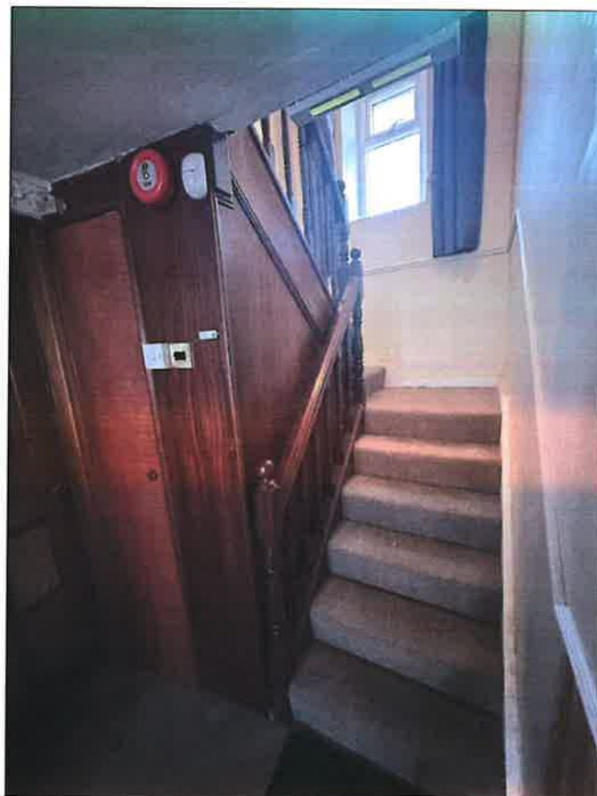
Plate 5: Modern hardwood staircase
