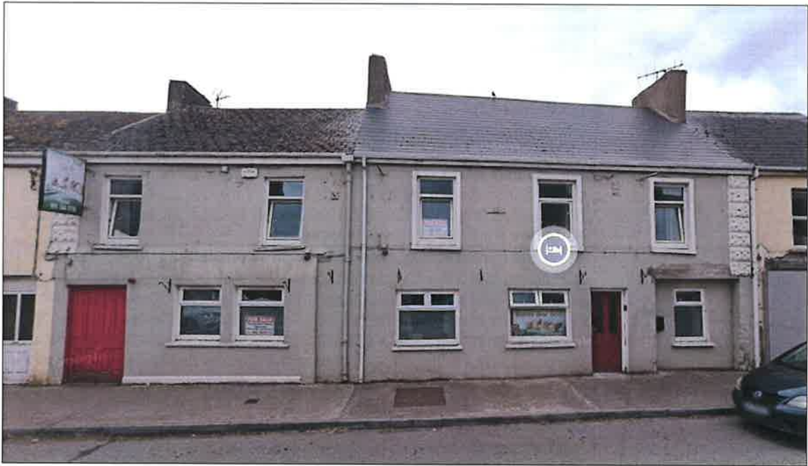
Figure 3: Street elevation of the building in 2022 (Source: Google Streetview)
