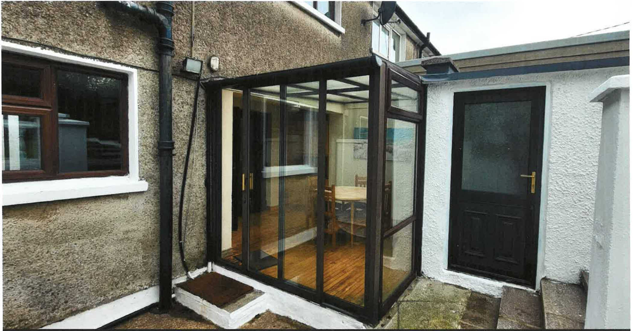
Photo of Extension to rear of 11 Raheen Park Youghal. (Shed to right is part of original structure)
