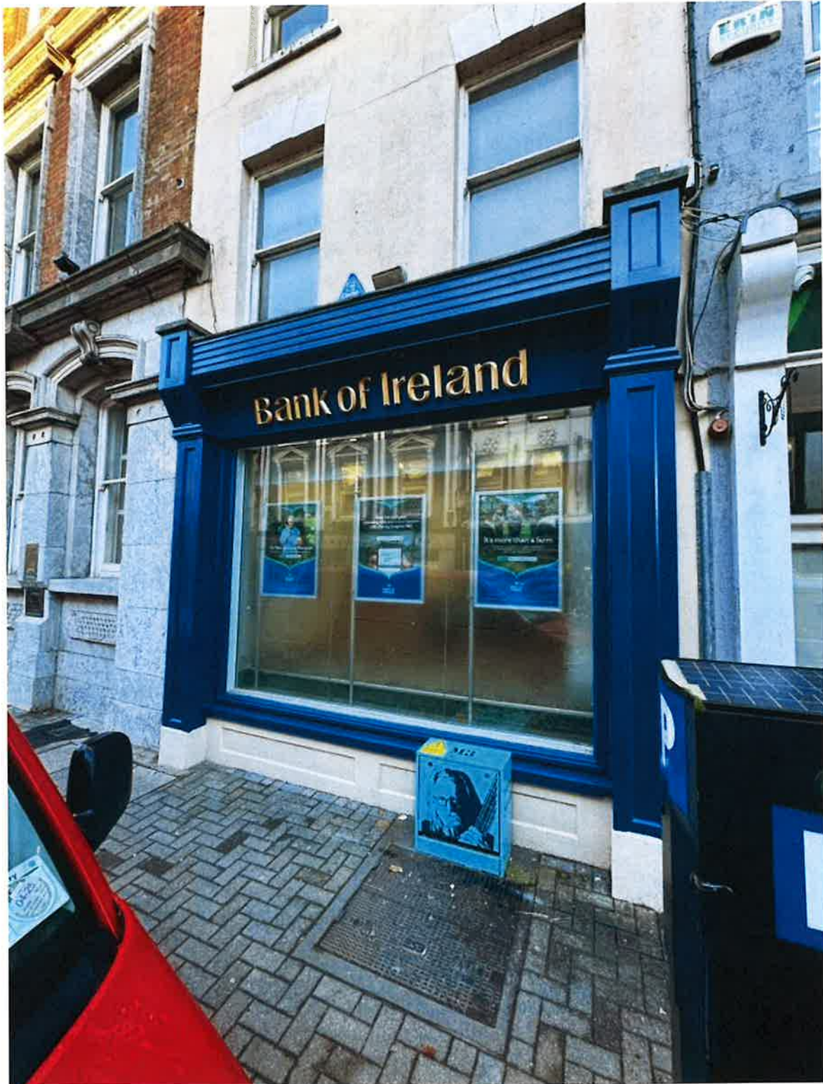
Plate 4: Modern shopfront to No. 9 South Main Street – this unit was amalgamated into the purpose-built bank building that occupies No. 8 South Main Street.
