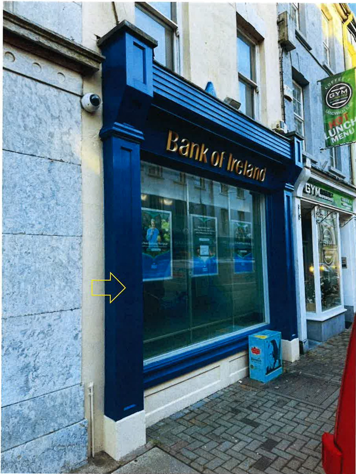
Plate 5: View of proposed location of the external defibrillator (on the timber pilaster of the modern shopfront)
