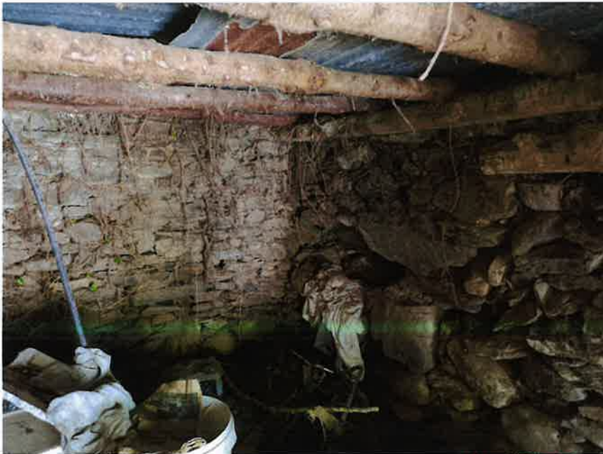
Image 003: Interior of Existing Stone Outbuildings
