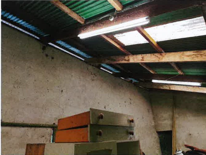
Image 002: Interior of 148.90M2 Barn
