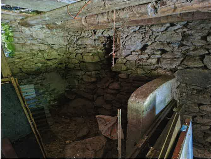
Image 004: Interior of Existing Stone Outbuildings
