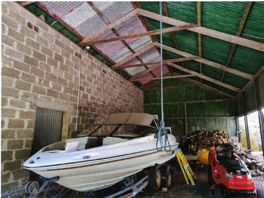
Image 001: Interior of 148.90M 2 Barn
